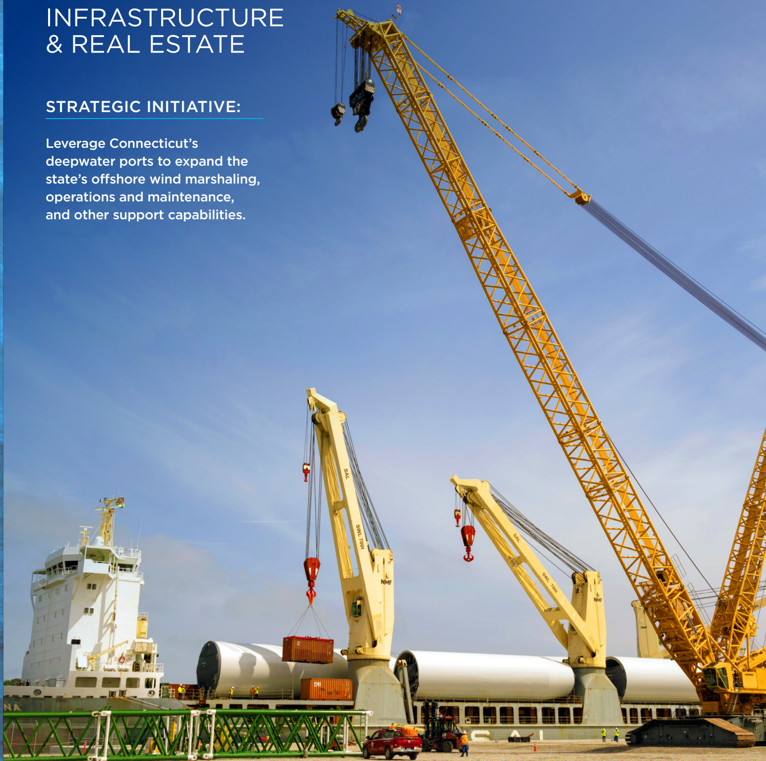
July 2023: Workers unload tower sections delivered to State Pier Terminal in New London for staging and assembly before deployment to offshore lease areas in support of Ørsted/Eversource's South Fork Wind project. Photo credit: Ørsted
