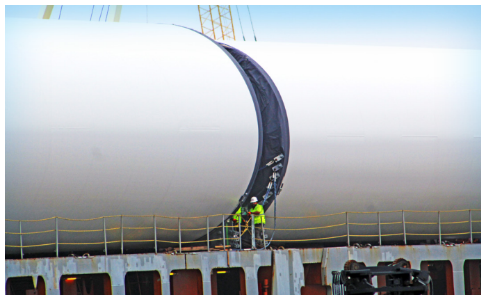
Tower sections being offloaded at State Pier Terminal. Photo credit: Quinn & Hary Marketing/Public Relations
