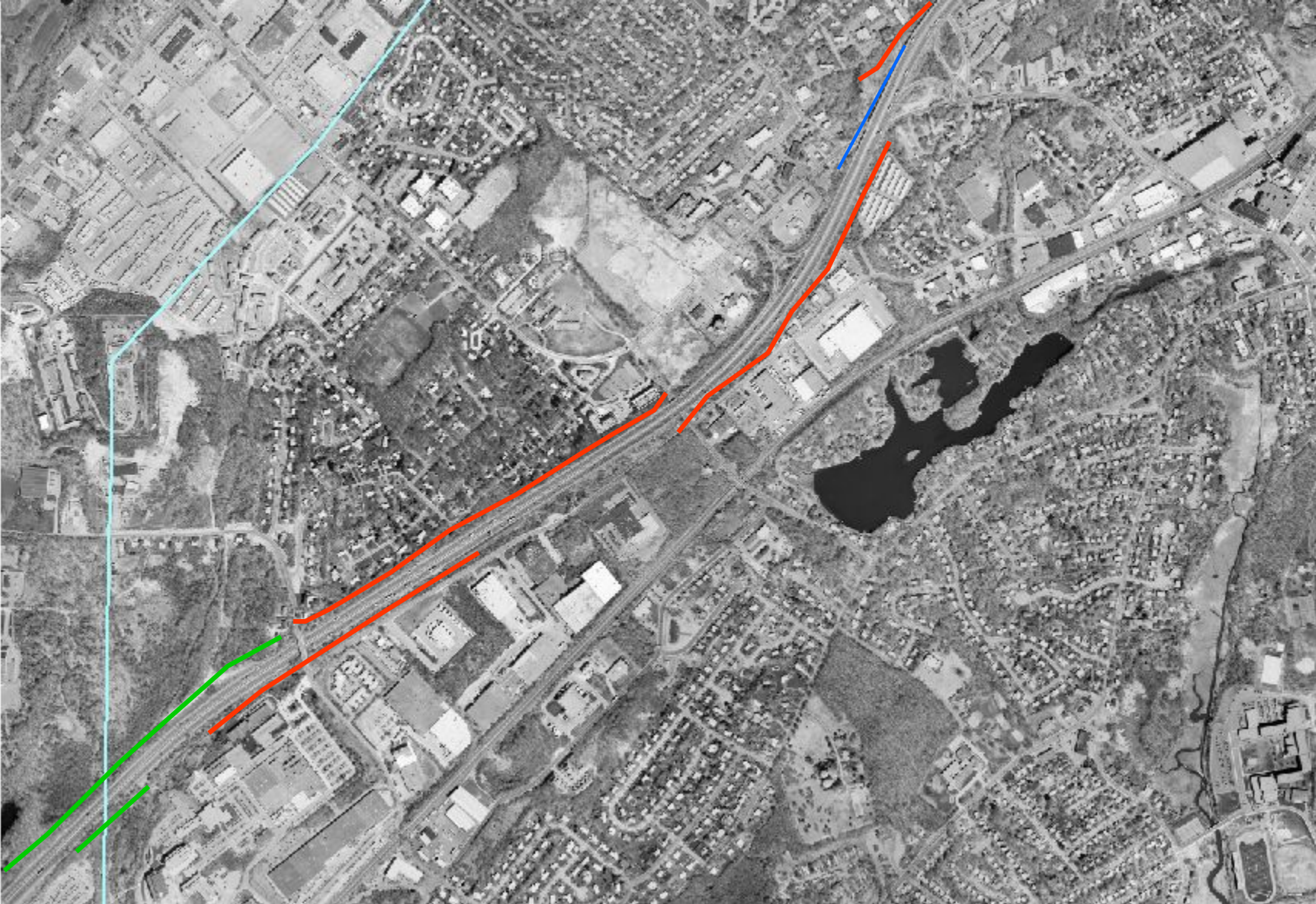
Flood plain/wetland , raised bed/rock cuts , and buildings adjacent to highway
