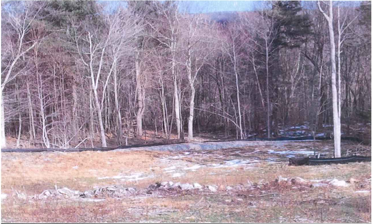
E&S Controls on Eastern Boundary as viewed from access
