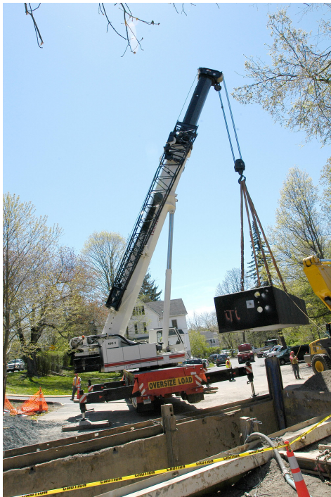
Figure 3-1: Typical Splice Vault Installation
