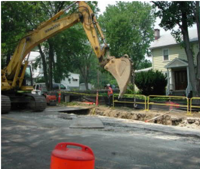
Figure 3-3: Typical Cable Trench in Residential Area
