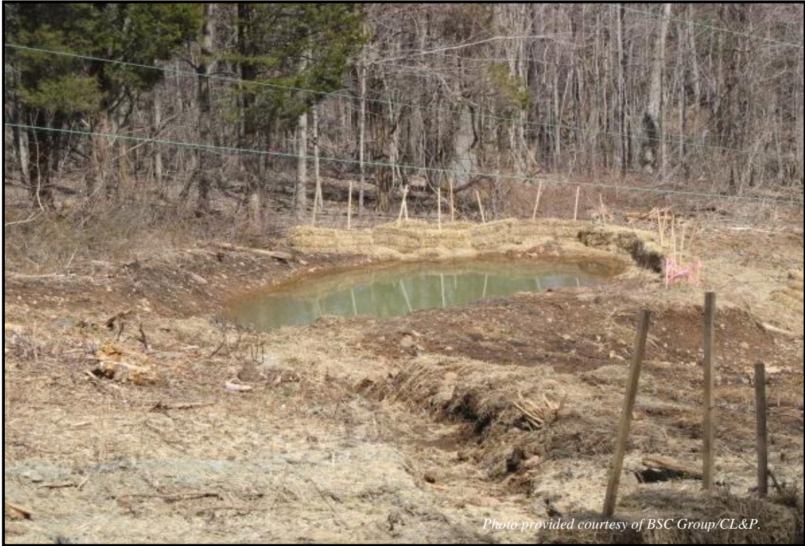
Sedimentation basin with hay bale filters.
