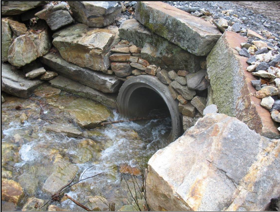
Culvert and riprap for stream crossing.
