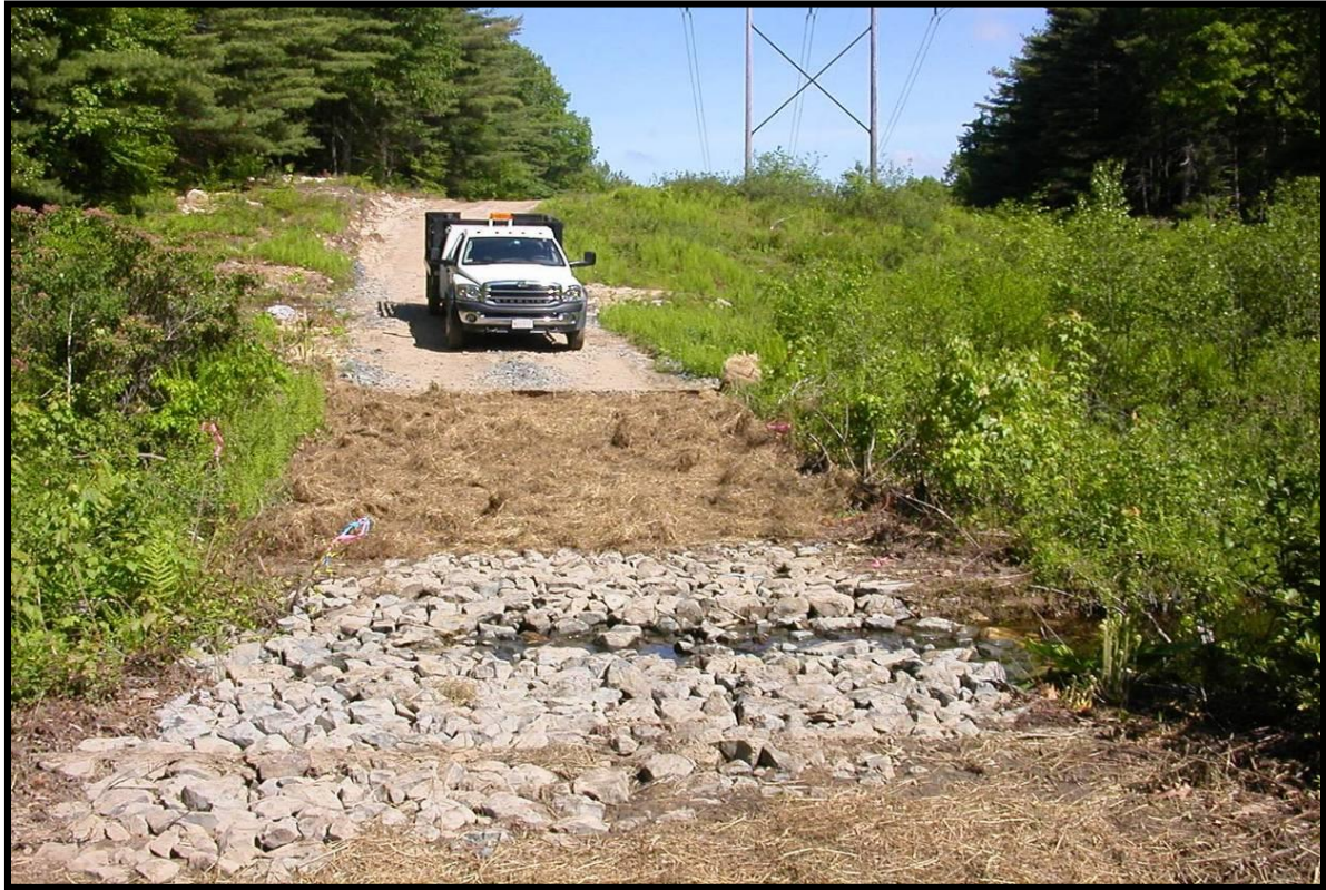
Intermittent stream crossing with angular stone.
