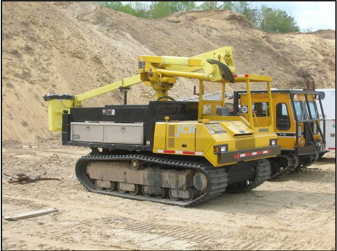
Equipment with rubberized tracks.
