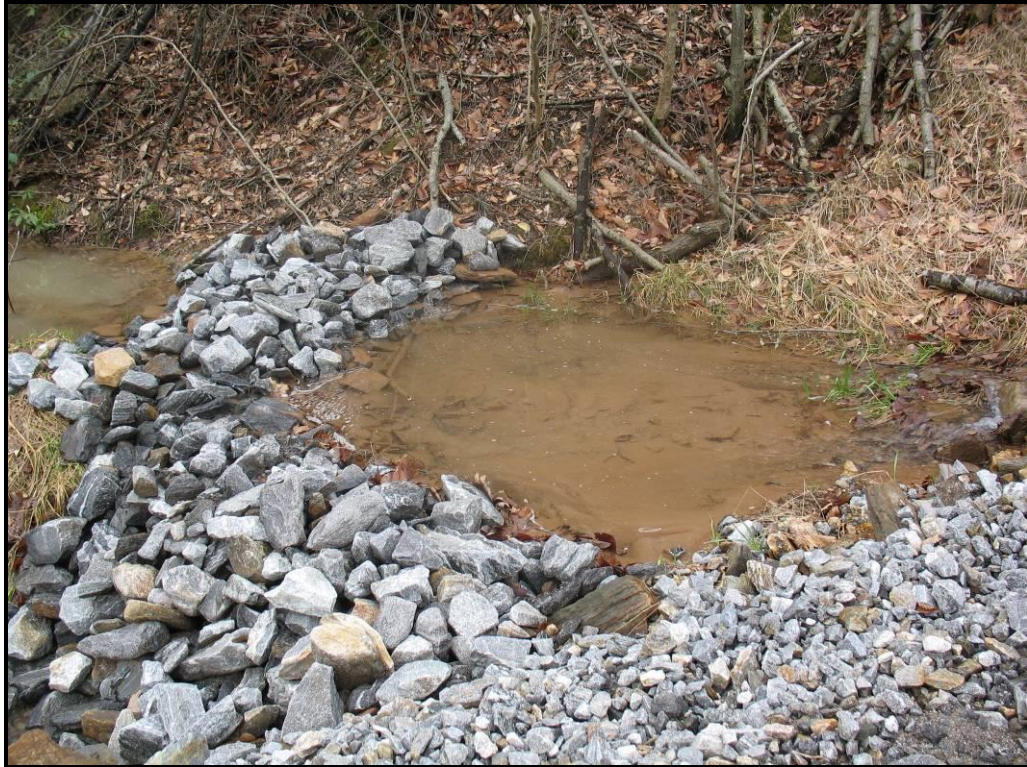
Stone check dam at construction site.
