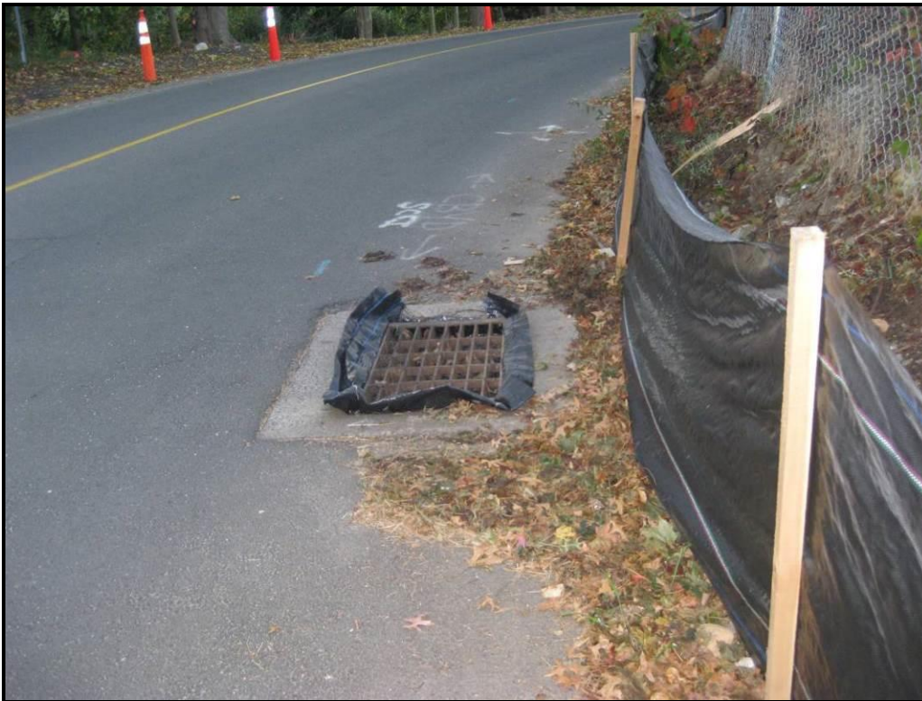
Catchbasin protected from sedimentation by filter fabric.
