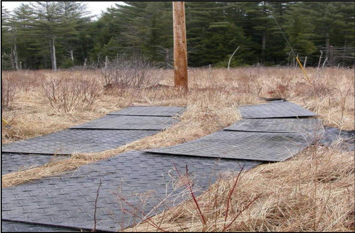
AlturnaMAT® tracks to utility pole in wetland.
