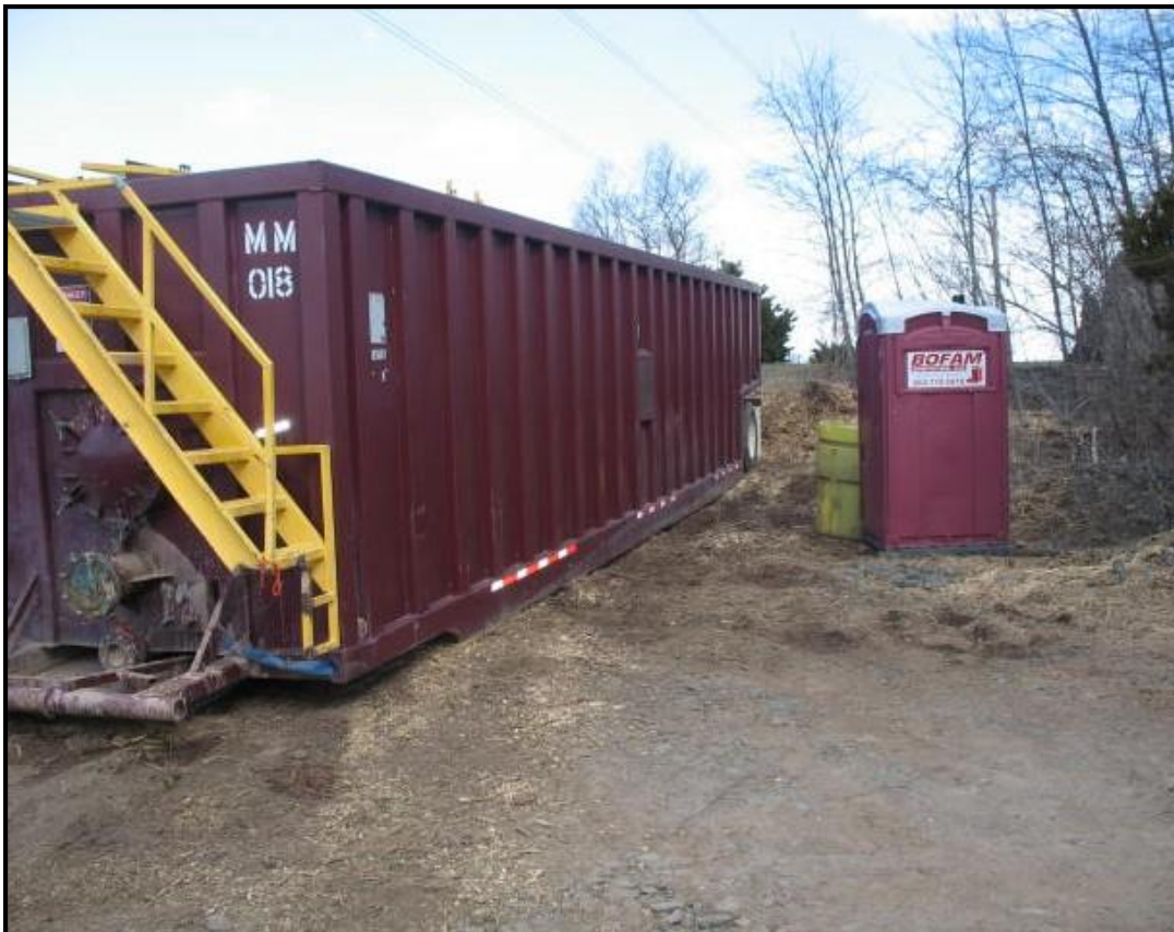
Frac tank on-site for dewatering activities.
