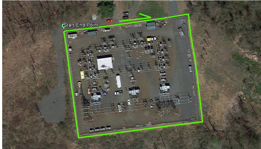
Newington Substation (Newington, CT)
