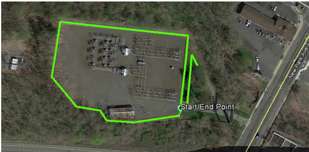
Southwest Hartford Substation (Hartford, CT)
