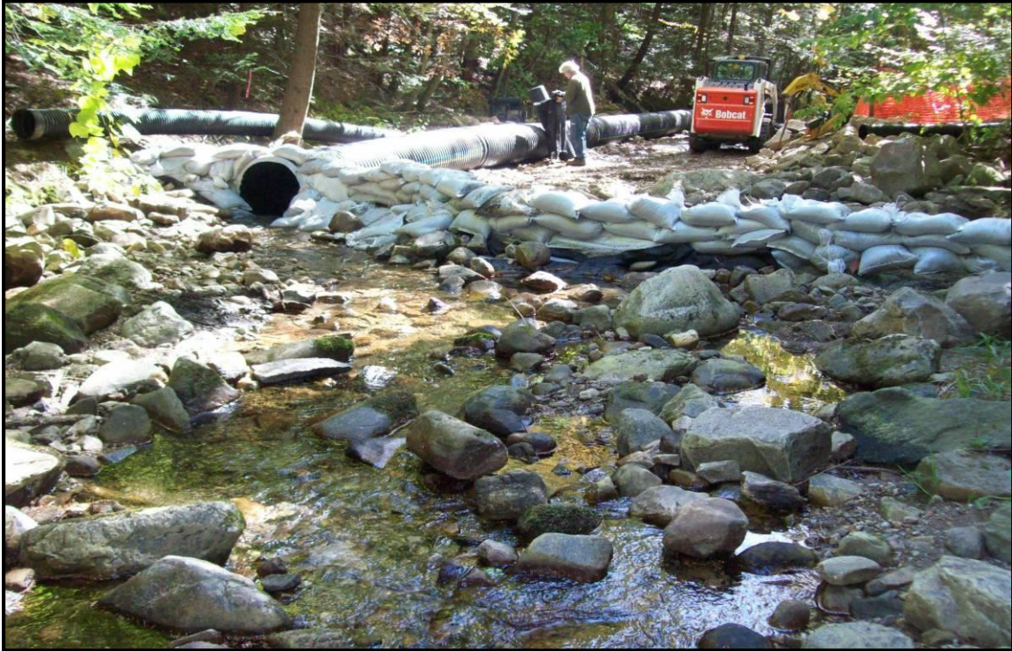
Sand bag coffer dam and streamflow gravity bypass.
