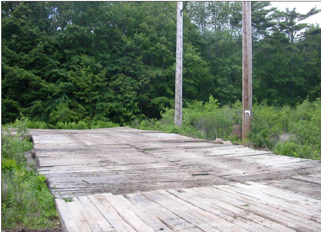
Construction mat wetland work-pad for de-energized work.
