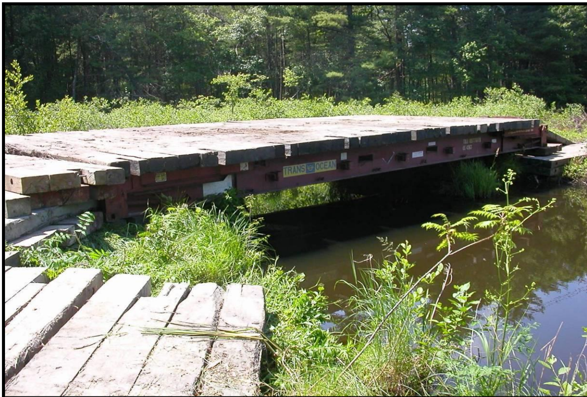
Rail car frame bridge crossing.
