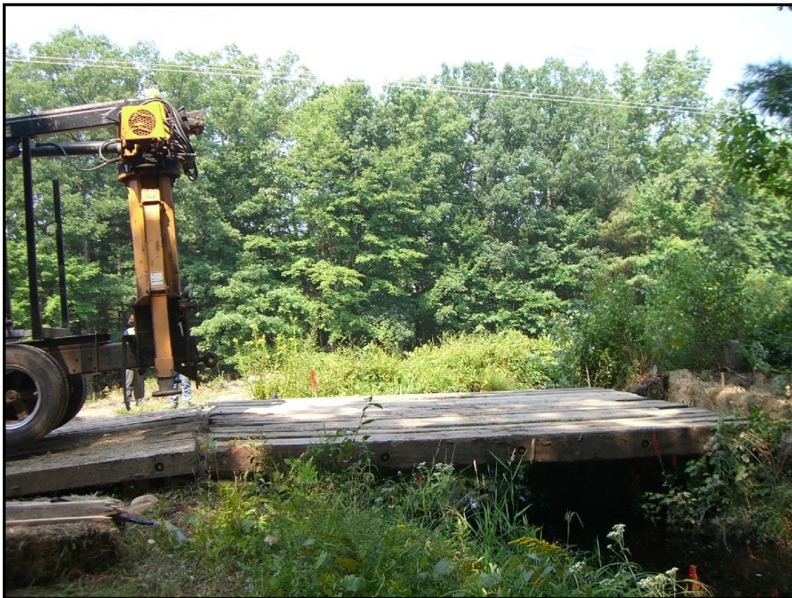
Construction mat bridge.
