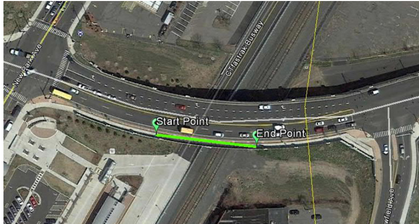
Flatbush Avenue (West Hartford, CT): Overhead Line Segment
