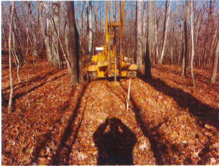
DRILLING TYPICAL PROBE
