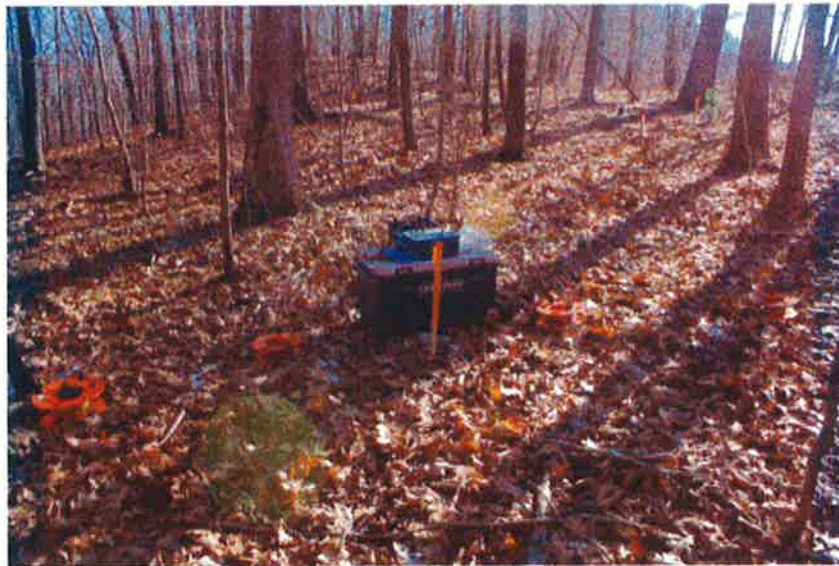
TYPICAL RESISTIVITY TESTING
