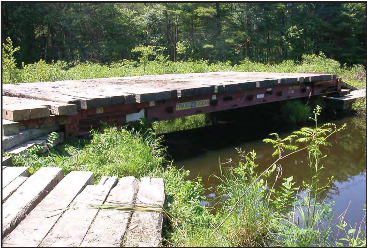
Rail car bridge crossing.
