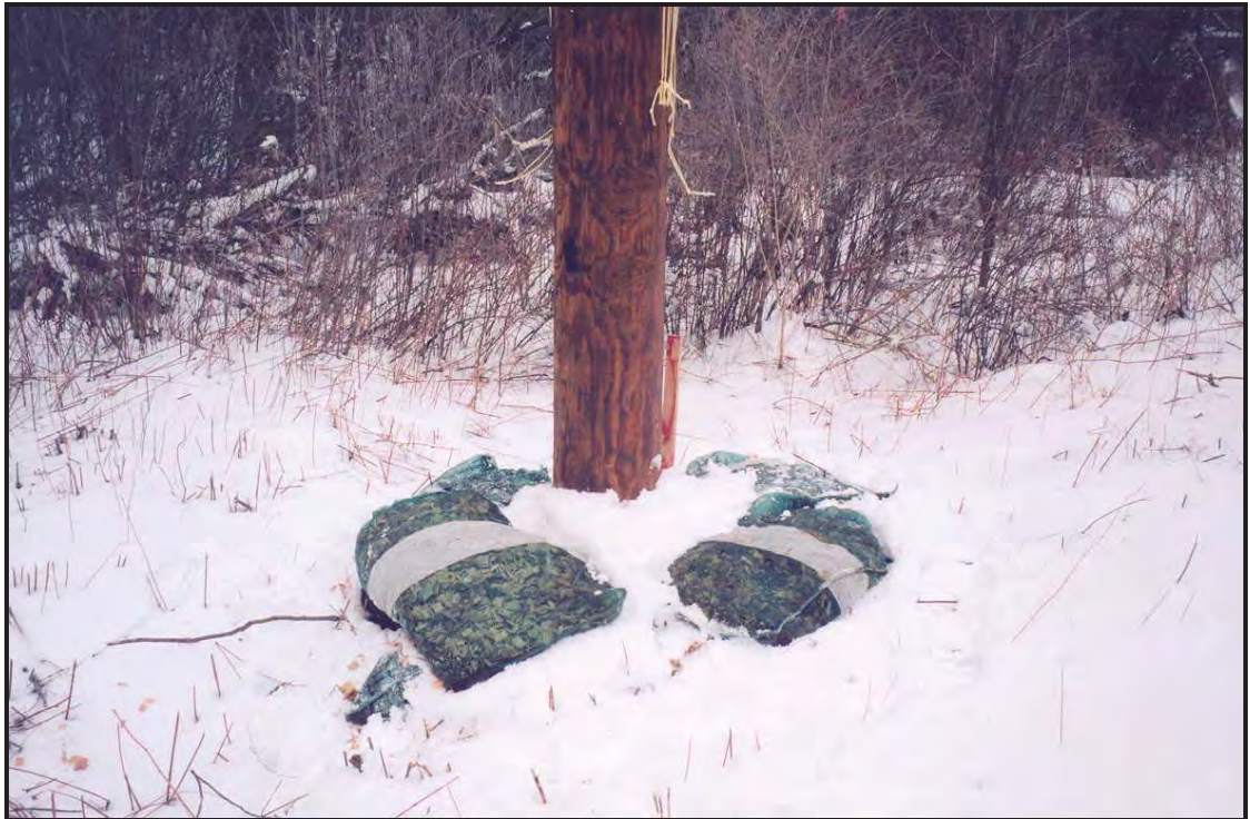
Wood chips in photo-degradable bags used to stabilize soils.
