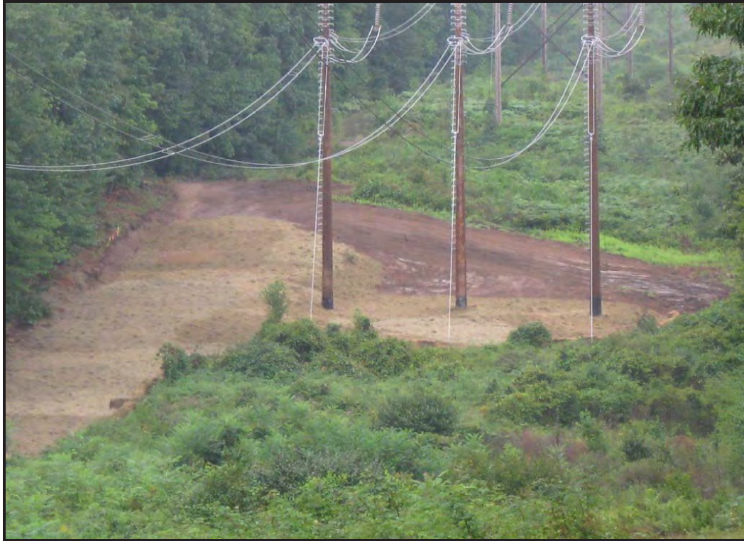
Loaming and seeding of recently disturbed right-of-way.
