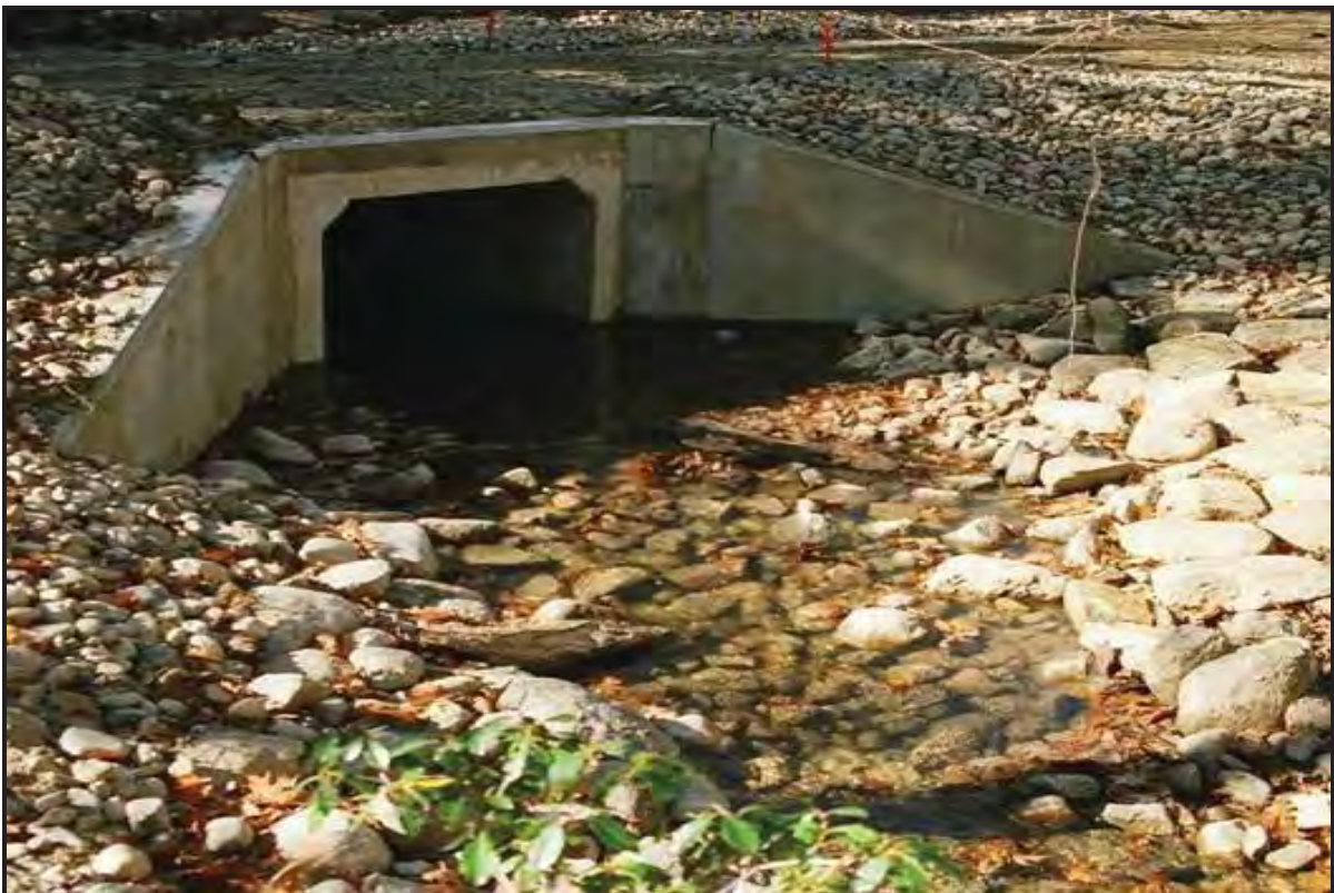
Embedded box culvert with wing walls.
