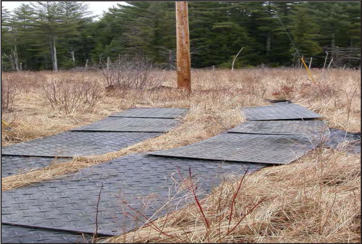
AlturnaMAT® tracks to utility pole in wetland.
