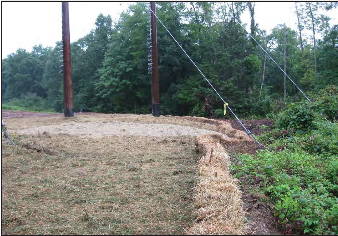
Typical view of light mulching atop unstable, seeded soils.
