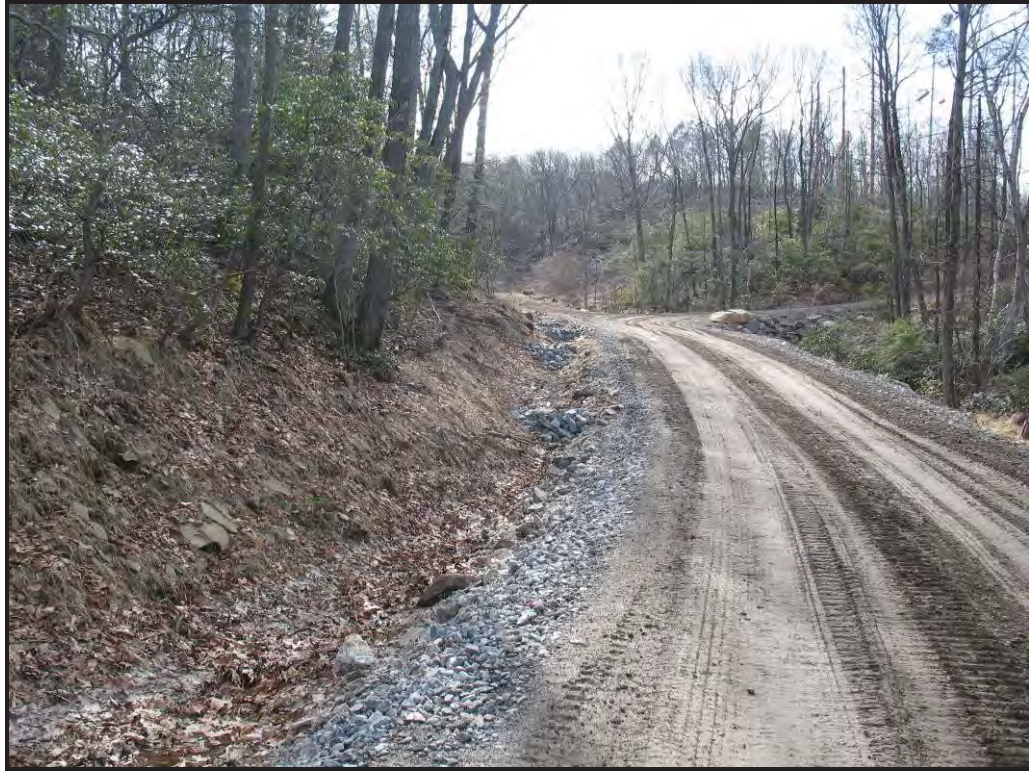
Stone check dams at construction site.
