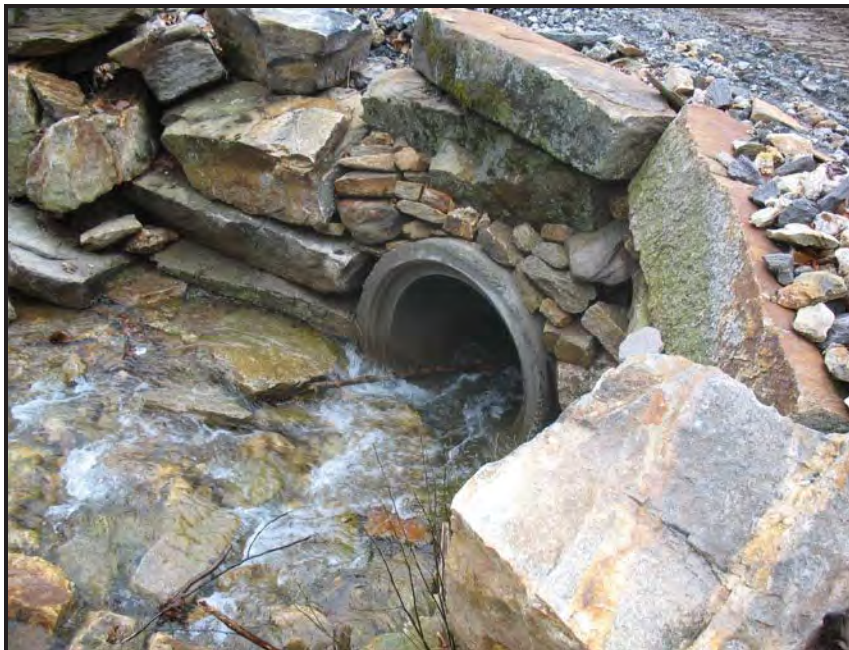
Culvert and riprap for stream crossing.
