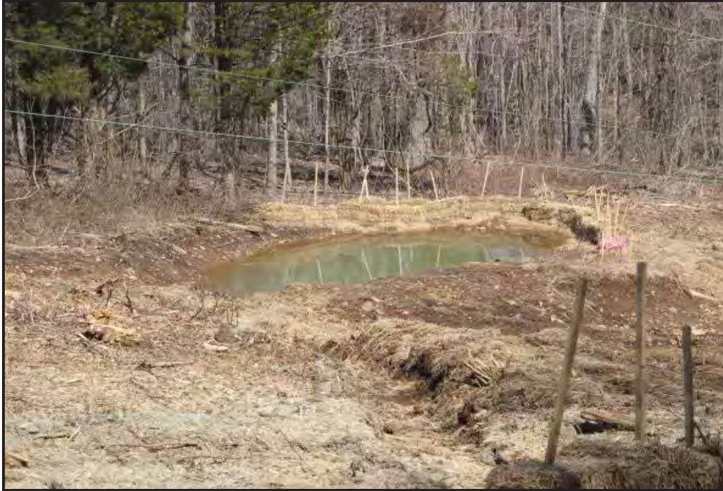
Sedimentation basin with haybale filters.
