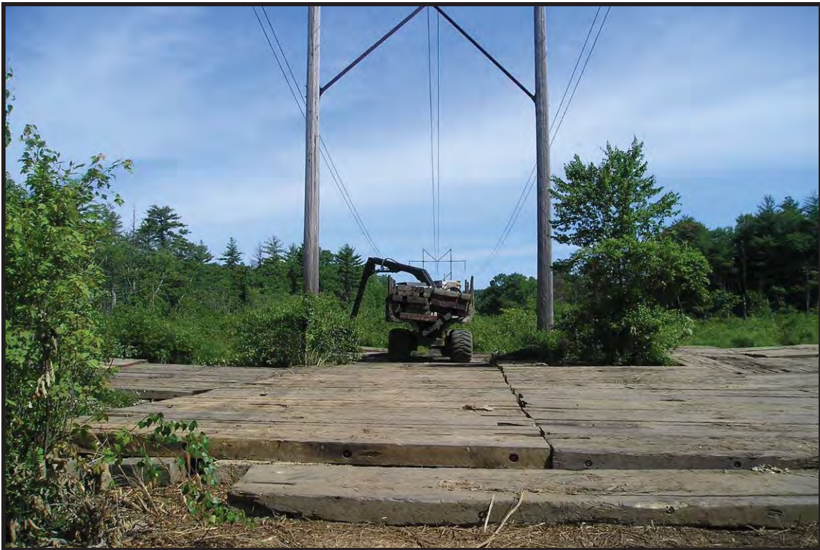
Timber mat wetland work platform.
