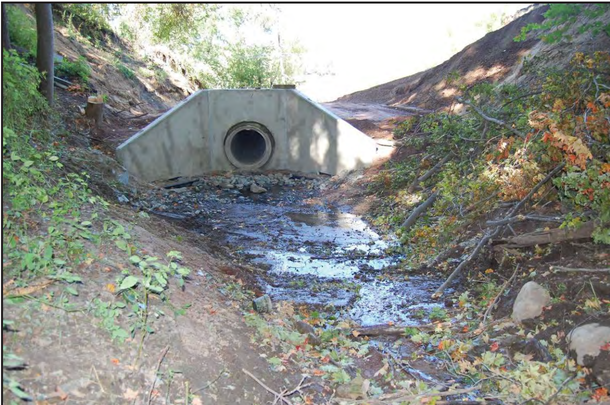
Installing a pipe culvert.
