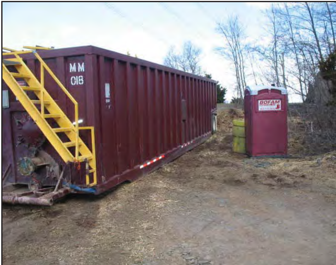
Frac tank on-site for dewatering activities.
