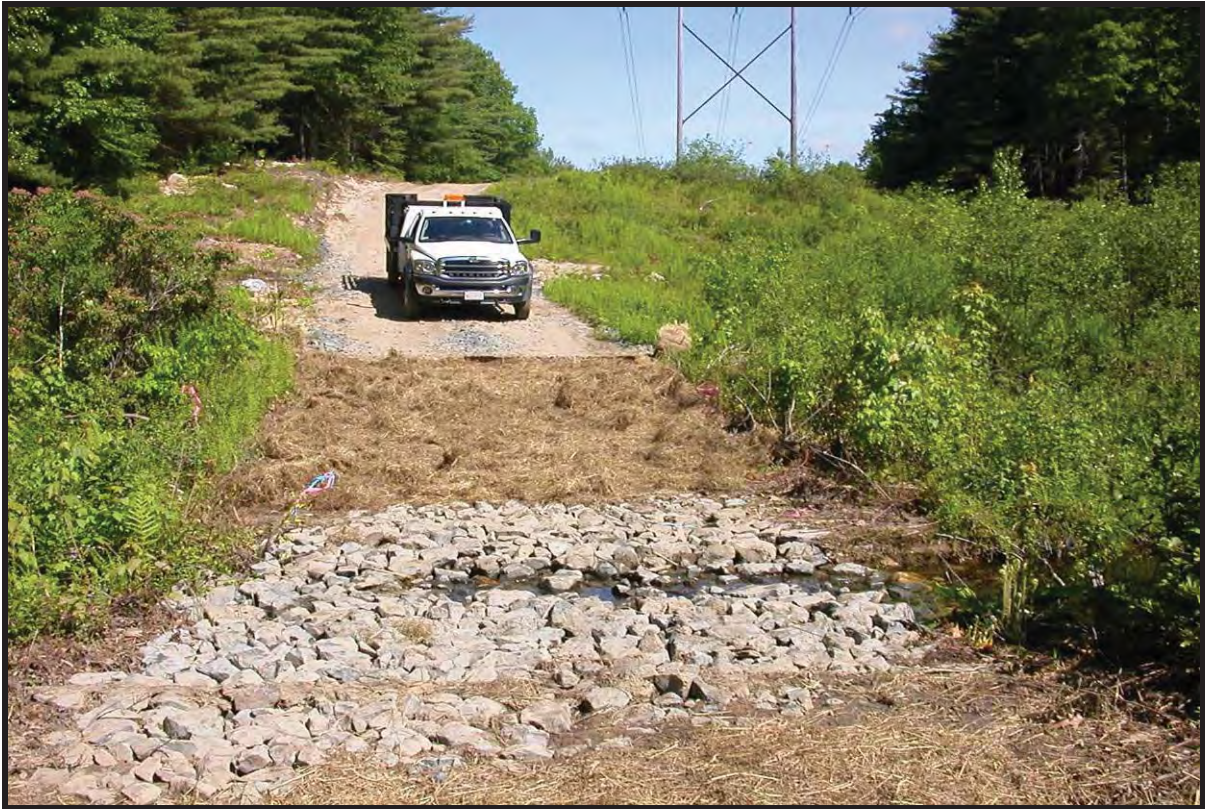
Intermittent stream crossing with angular stone.
