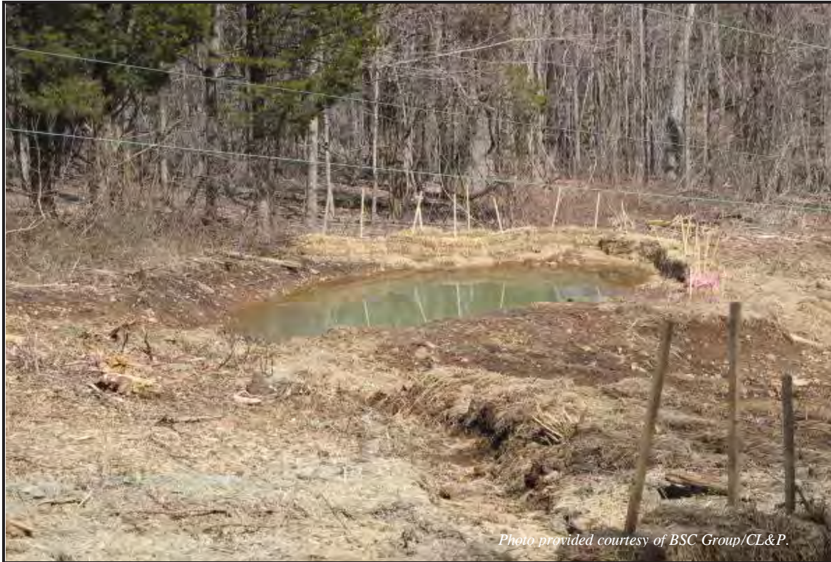
Sedimentation basin with haybale filters.
