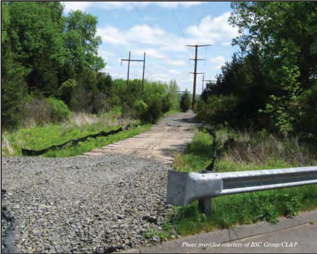
Construction entrance track pad.
