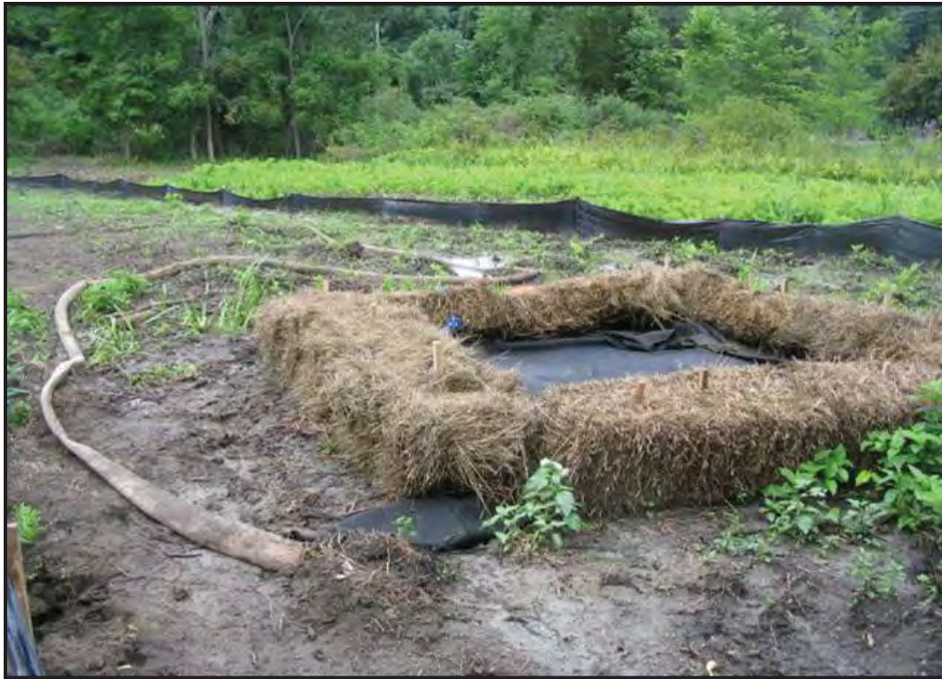
Dewatering to filter "sock" surrounded by haybales.
