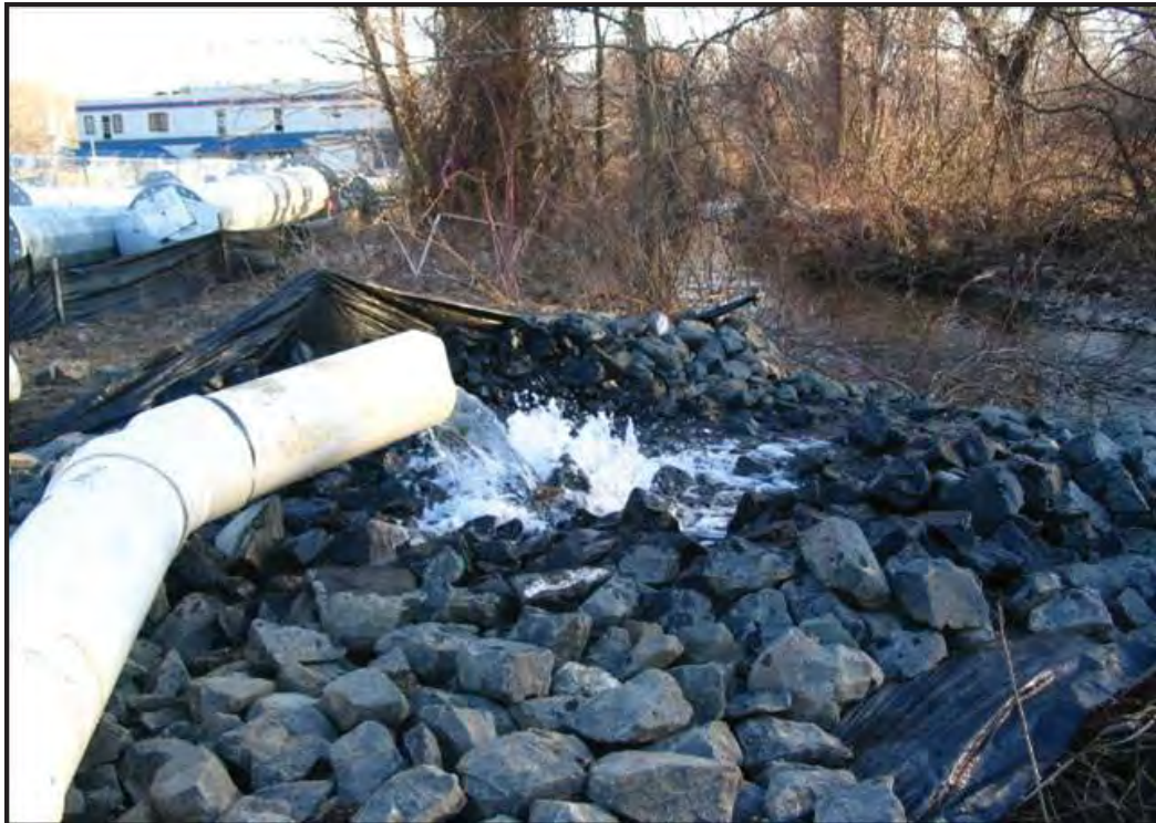
Riprap underlain by geotextile fabric
