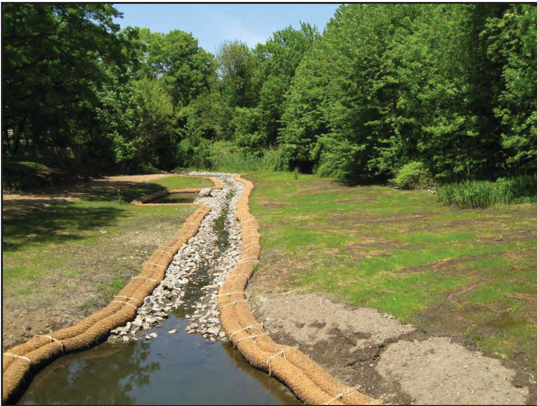
Coir logs used to restore a stream bed and banks.
