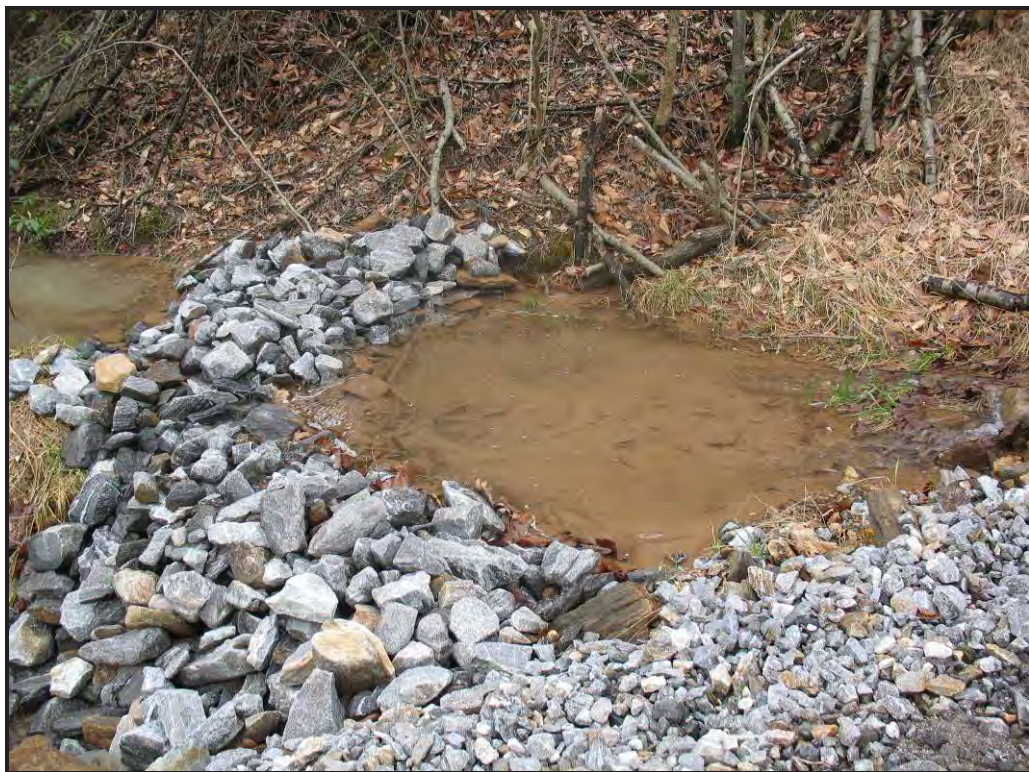
Stone check dam at construction site.
