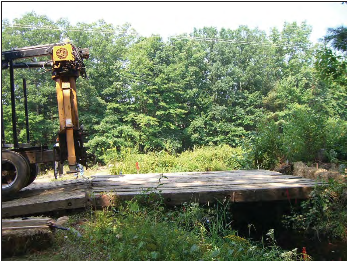
Timber mat bridge.
