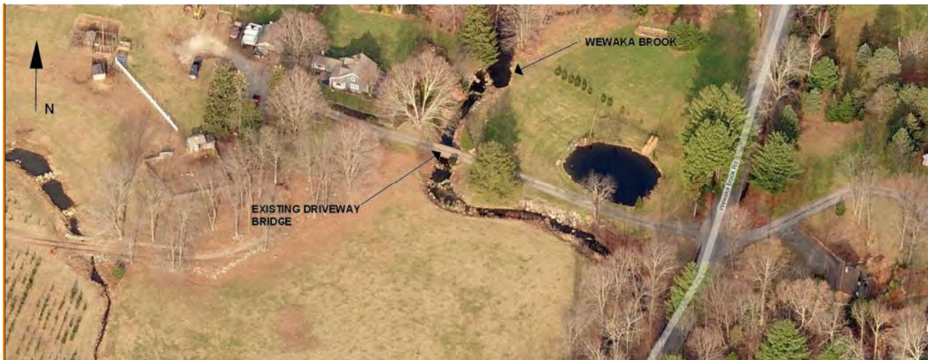
Figure 1 Aerial Image of existing bridge over Wewaka Brook
