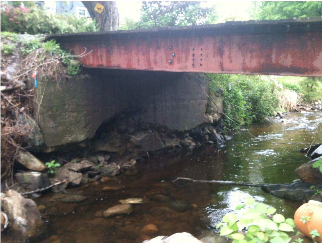
Photo 1: Existing Bridge Structure Across Wewaka Brook
