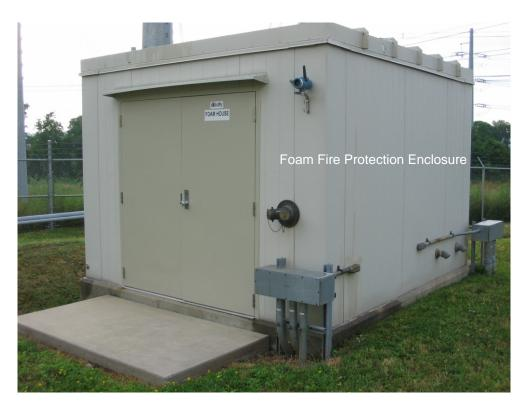
A normal environment will be maintained in the enclosures. Each enclosure will be inspected periodically and temperatures will be monitored continuously via wireless temperature probes.
