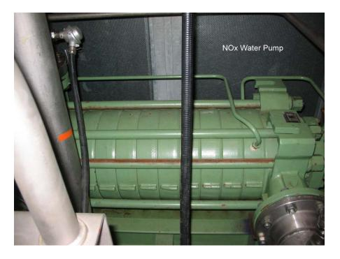
Pumps and piping will be emptied and drained and then stored in a dry condition, with the pumps being isolated electrically. Contactors and breakers will be racked out.
