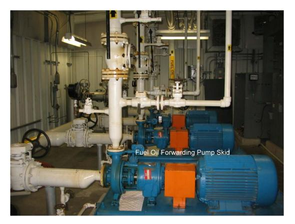
Pumps and piping will be emptied and drained and then stored in a dry condition, with the pumps being isolated electrically. Contactors and breakers will be racked out. Motor heaters will remain in service.
