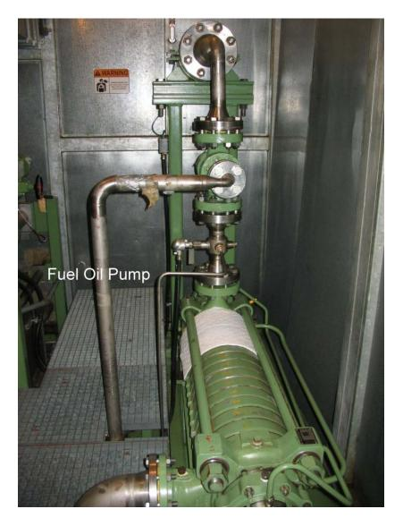
Pumps and piping will be emptied and drained and then stored in a dry condition, with the pumps being isolated electrically. Contactors and breakers will be racked out.
