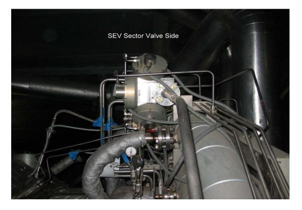
The trip shut-off valves and control valves associated with fuel oil combustion will be disassembled, preserved, and reassembled as per OEM recommendations. Sector and purge valves and all manual valves will be exercised routinely as part of the long term layup maintenance program. Valves and valve actuators will continue to be serviced as per OEM requirements.
