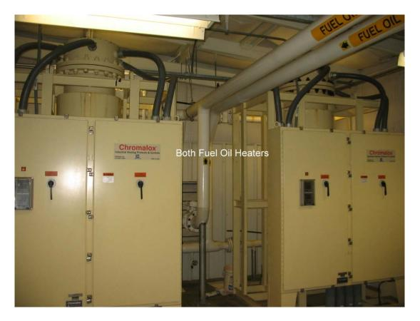
The fuel oil heaters will be emptied and stored in a dry condition and isolated electrically. Recommended OEM layup instructions will be followed.
