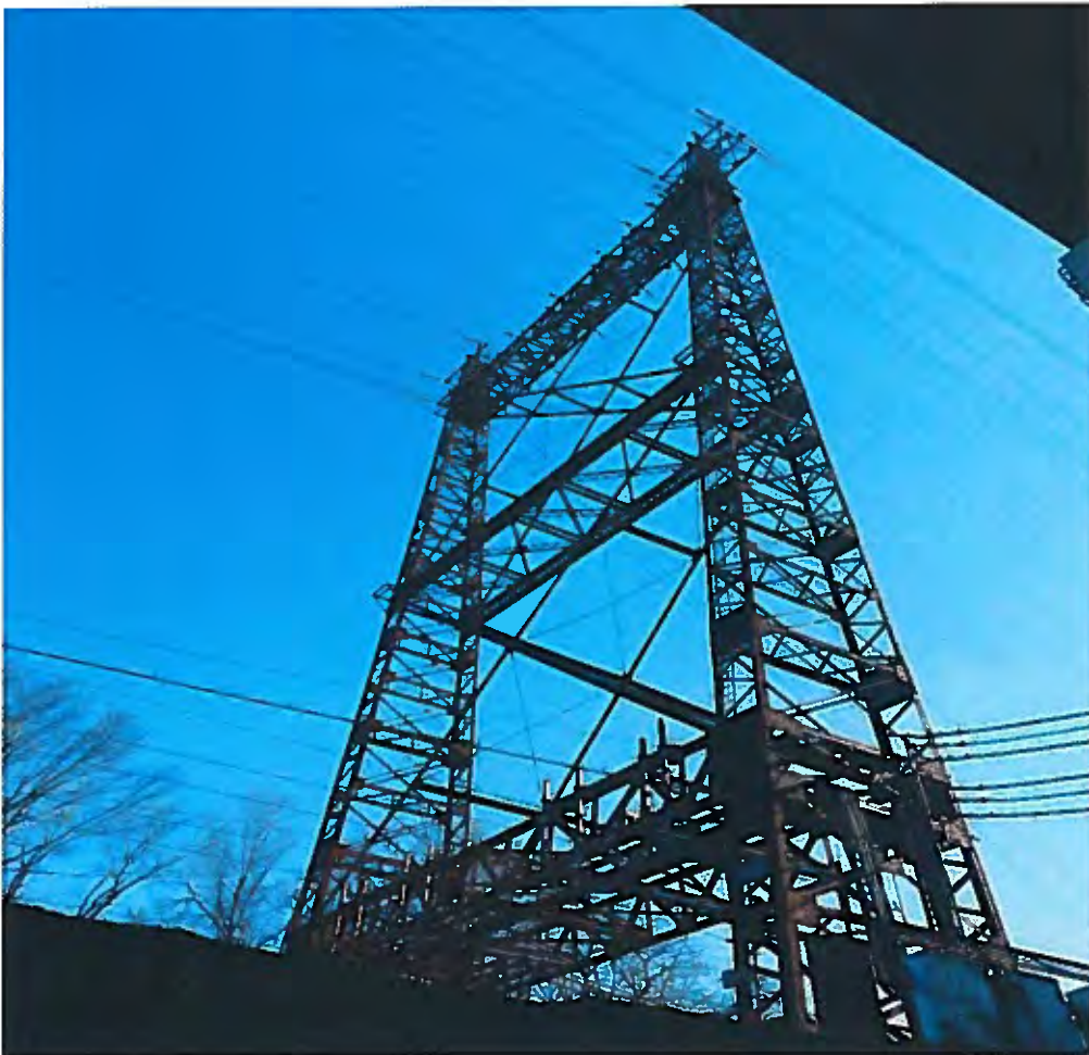
Figure A: Existing Structure
