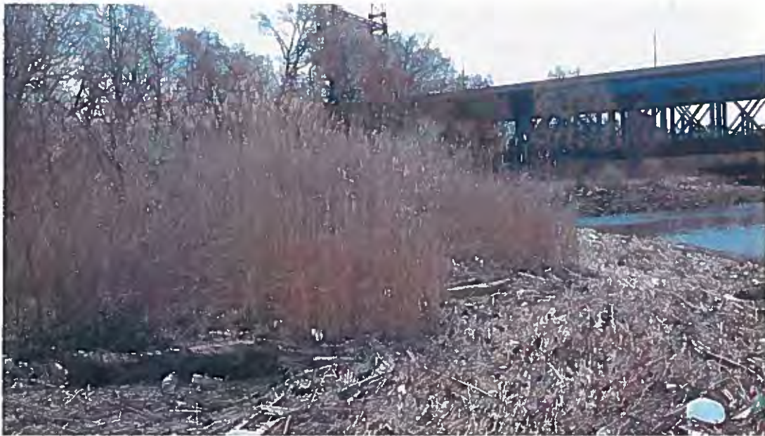
PHOTO 4: View of floodplain of watercourse 1 looking southeast.
