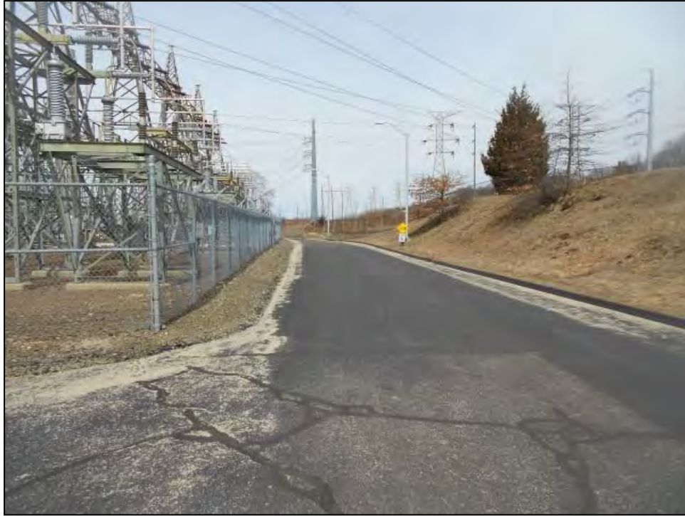
Photo 5. Overview photo of access to the proposed project area on the east side of the Housatonic River facing northwest.
