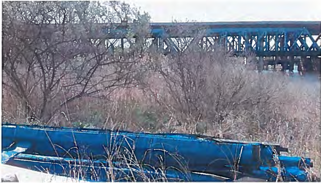
PHOTO 3: View of northern bench of water course 1 looking south.
