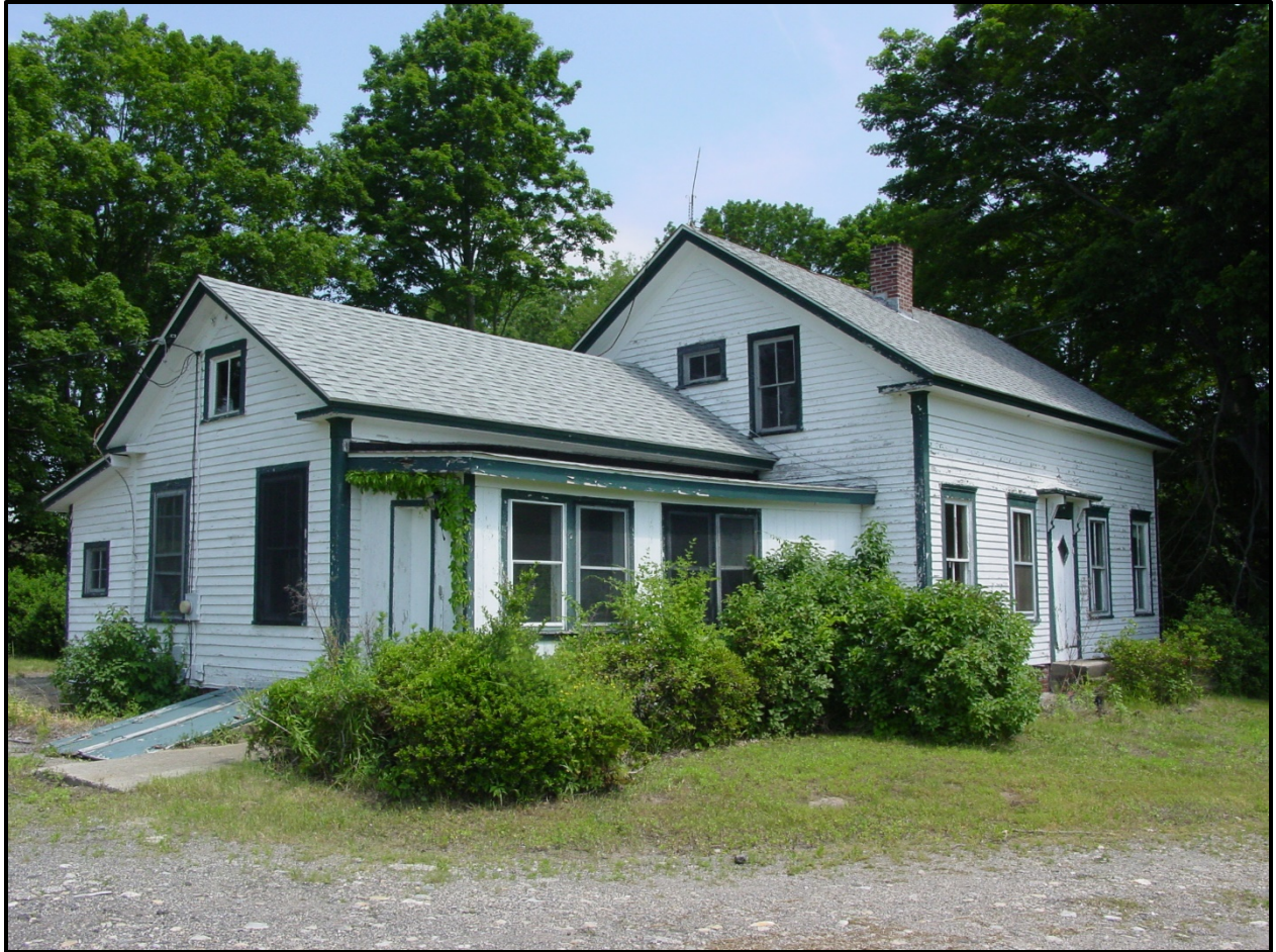
Photograph 9: House at 1 Williams Crossing, showing the partial return of the simple cornice across the gable ends.
