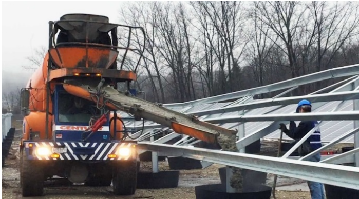
Utilizing concrete trucks to pour directly into tubs: 20 men install 1.64MW per week
