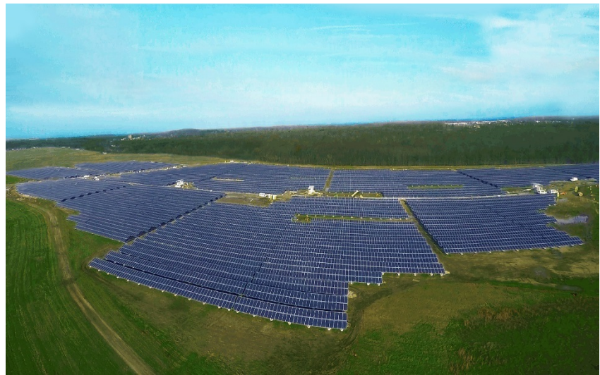
GameChange Pour-in-Place™ System 12.9 MW – New Jersey Landfill Site - Largest Superfund Site in the United States
