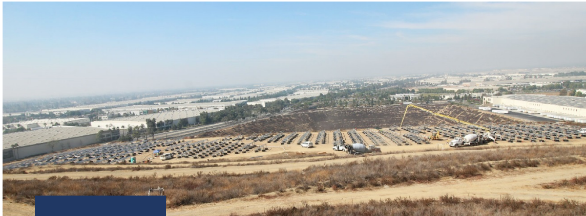
Utilizing concrete trucks to pour directly into tubs: 20 men install 1.64MW per week
