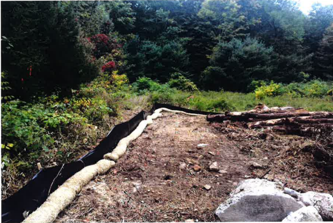
Photo 1: View of E&S perimeter controls looking southwest.
