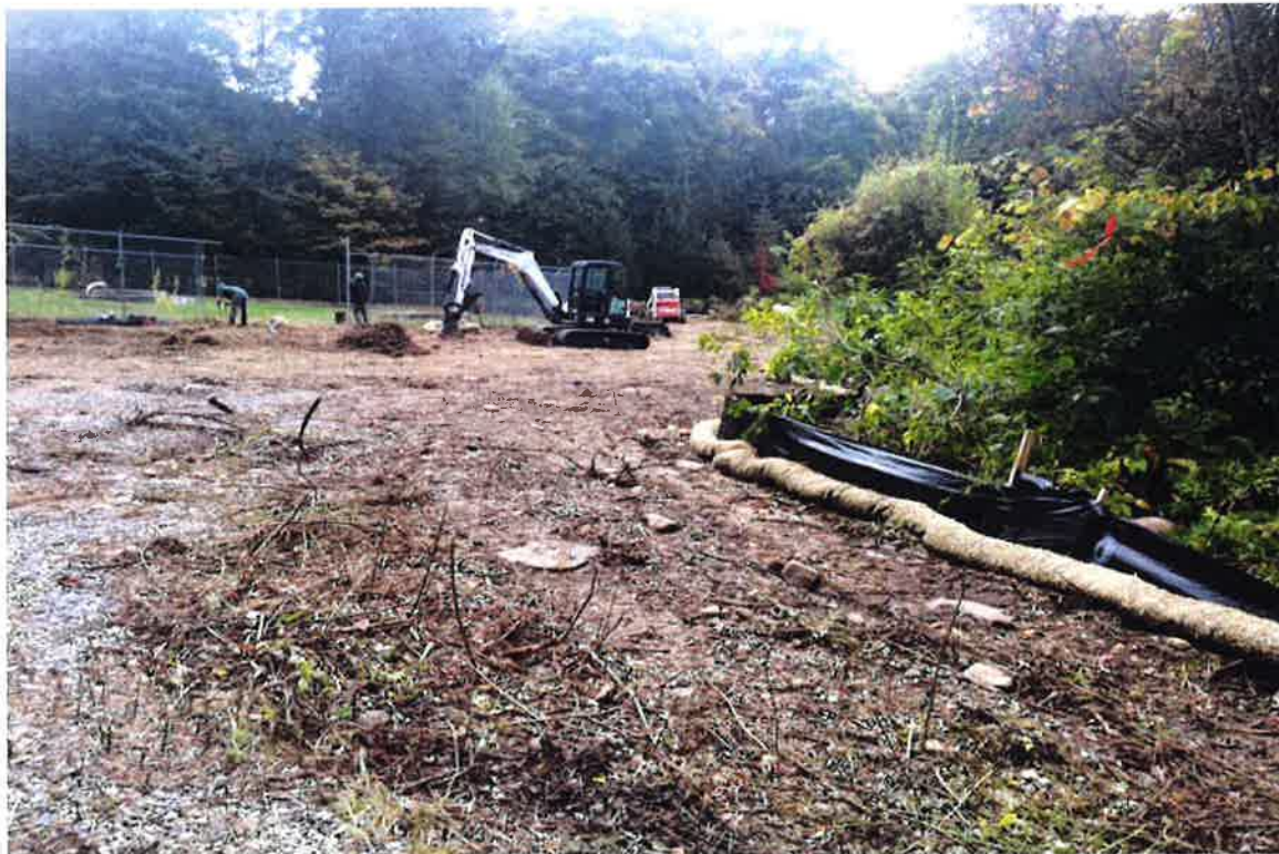
Photo 2: View of staging area looking south.
