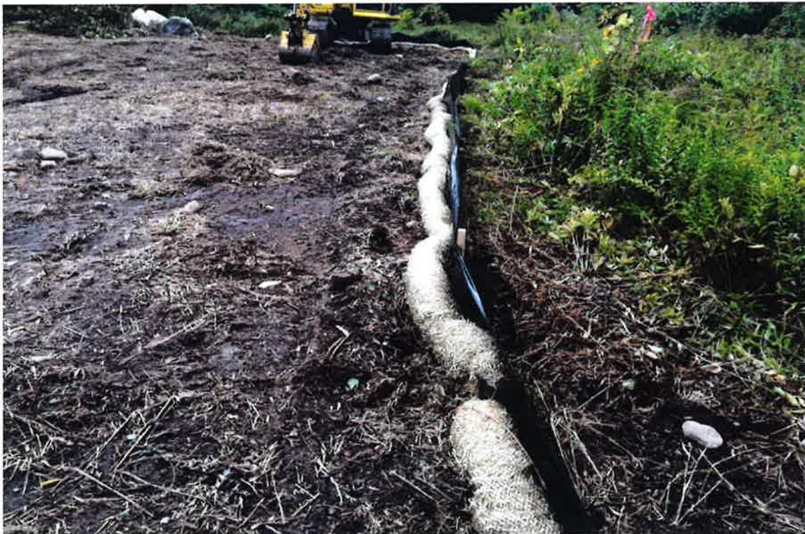
Photo 4: View of E&S perimeter controls looking east.
