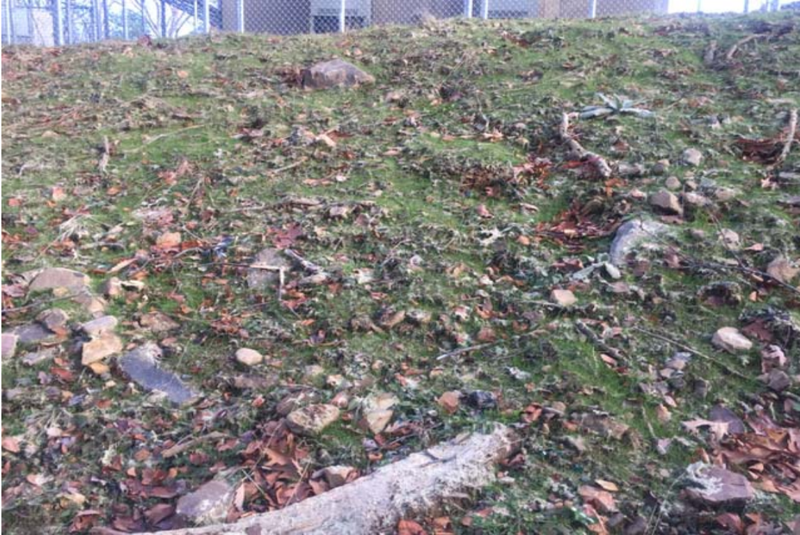
Photo 3: View of grass establishment on side slope looking east.
