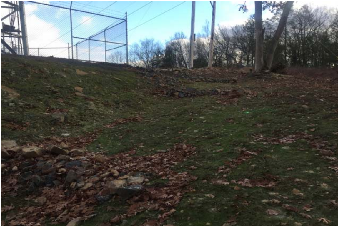
Photo 2: View of grass established in drainage swale and side slope looking south.
