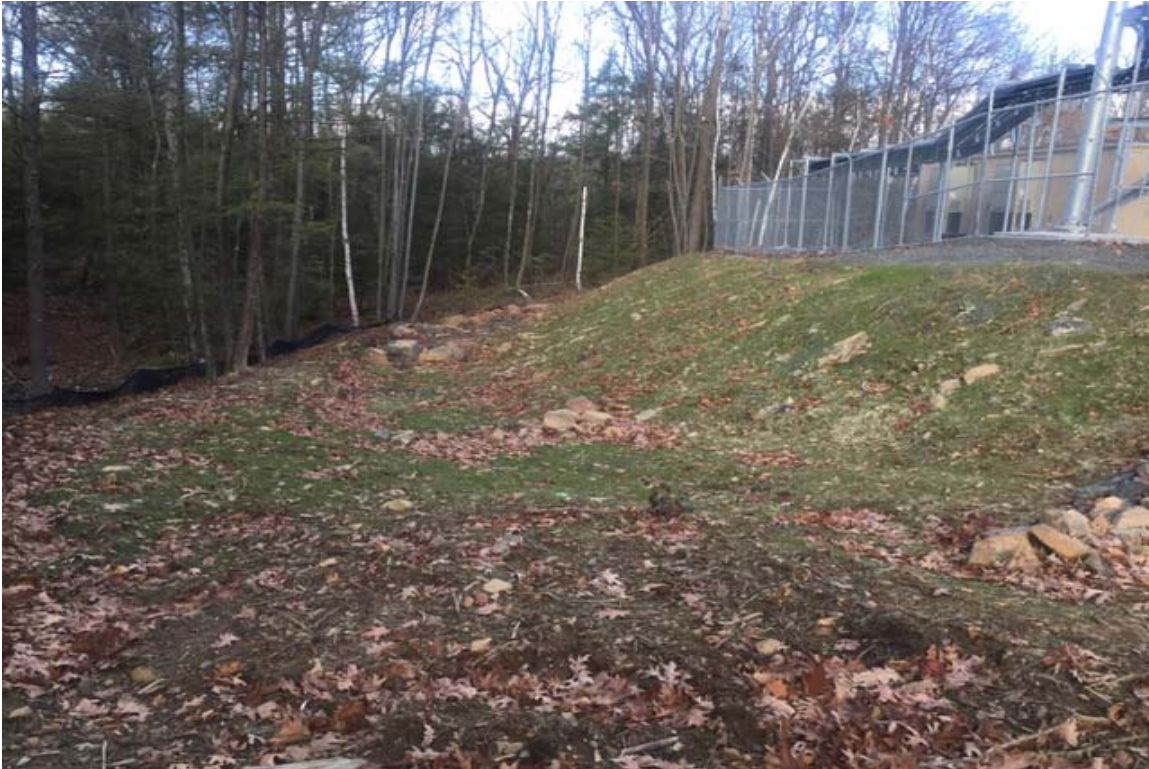
Photo 1: View of grass established in drainage swale and side slope looking north.
