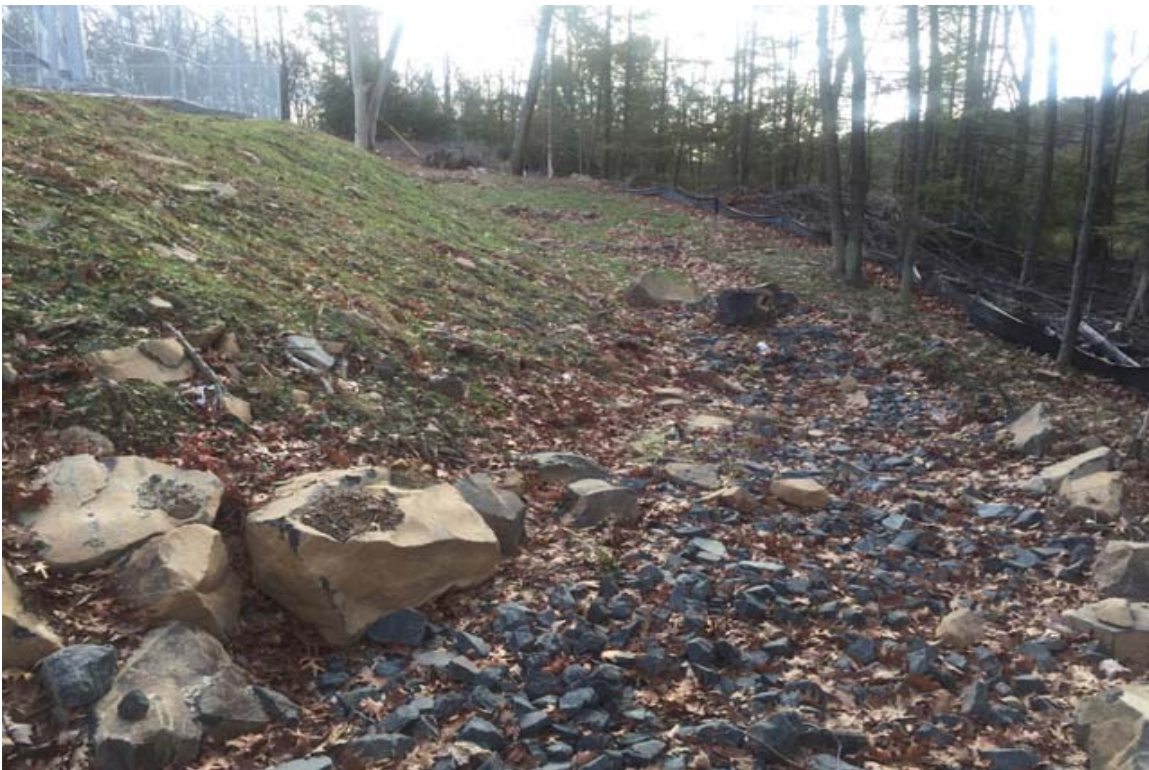
Photo 4: View of level spreader on side slope and drainage swale looking south.
