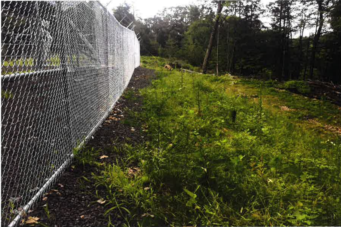
Photo 3: View of edge of southern compound side-slope looking west.
