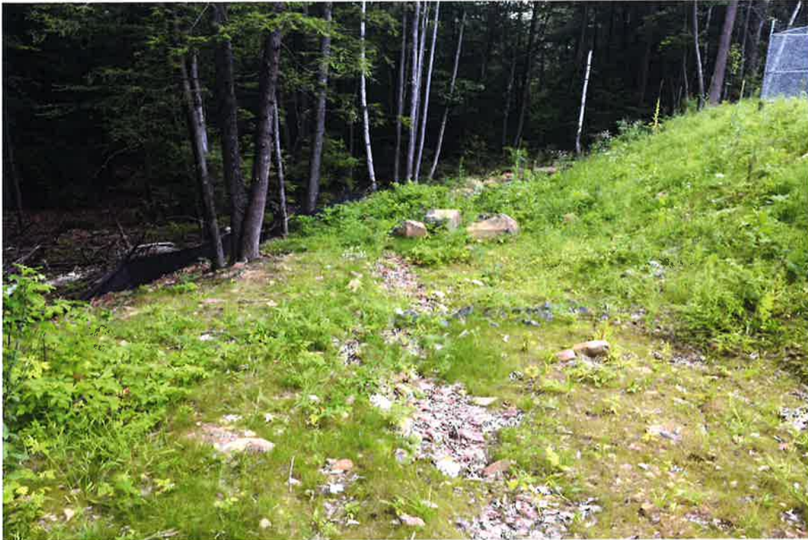
Photo 5: View of stabilized drainage swale and level spreader looking west.
