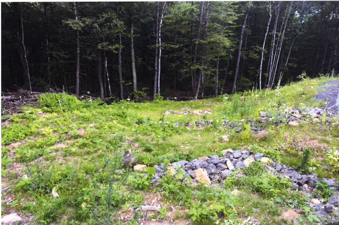
Photo 6: View of stabilized drainage swale looking west.
