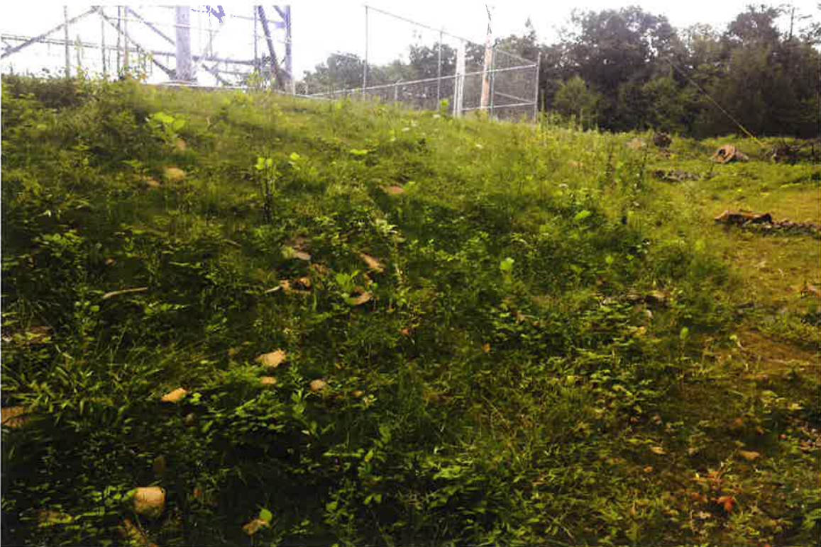
Photo 2: View of stabilized southern slope to compound looking north.
