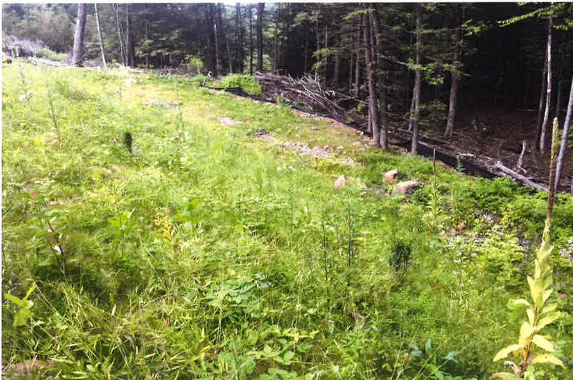
Photo 4: View of remaining silt fence along southern project boundary looking west.
