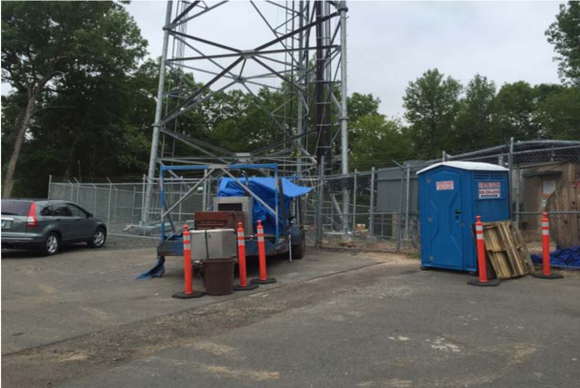
Photo 1: View of site under construction with new tower looking northwest.
