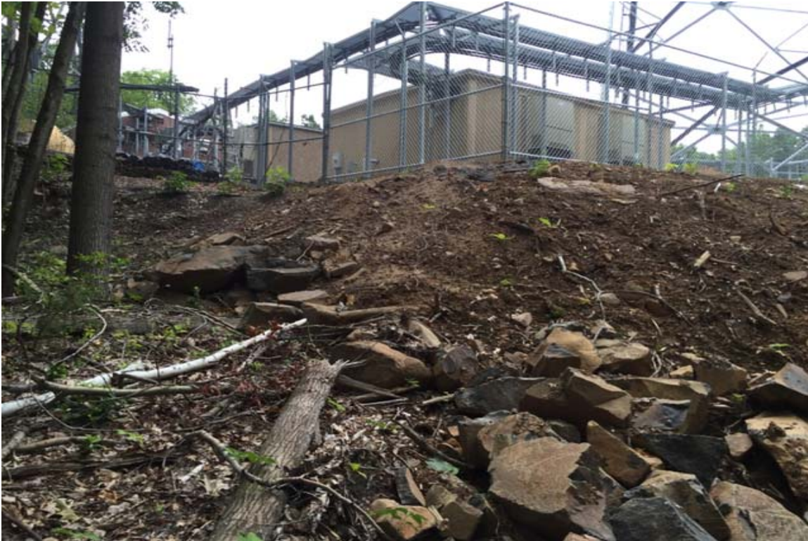
Photo 7: View of northwest corner of compound slope looking east – requires installation of erosion blanket and seeding.
