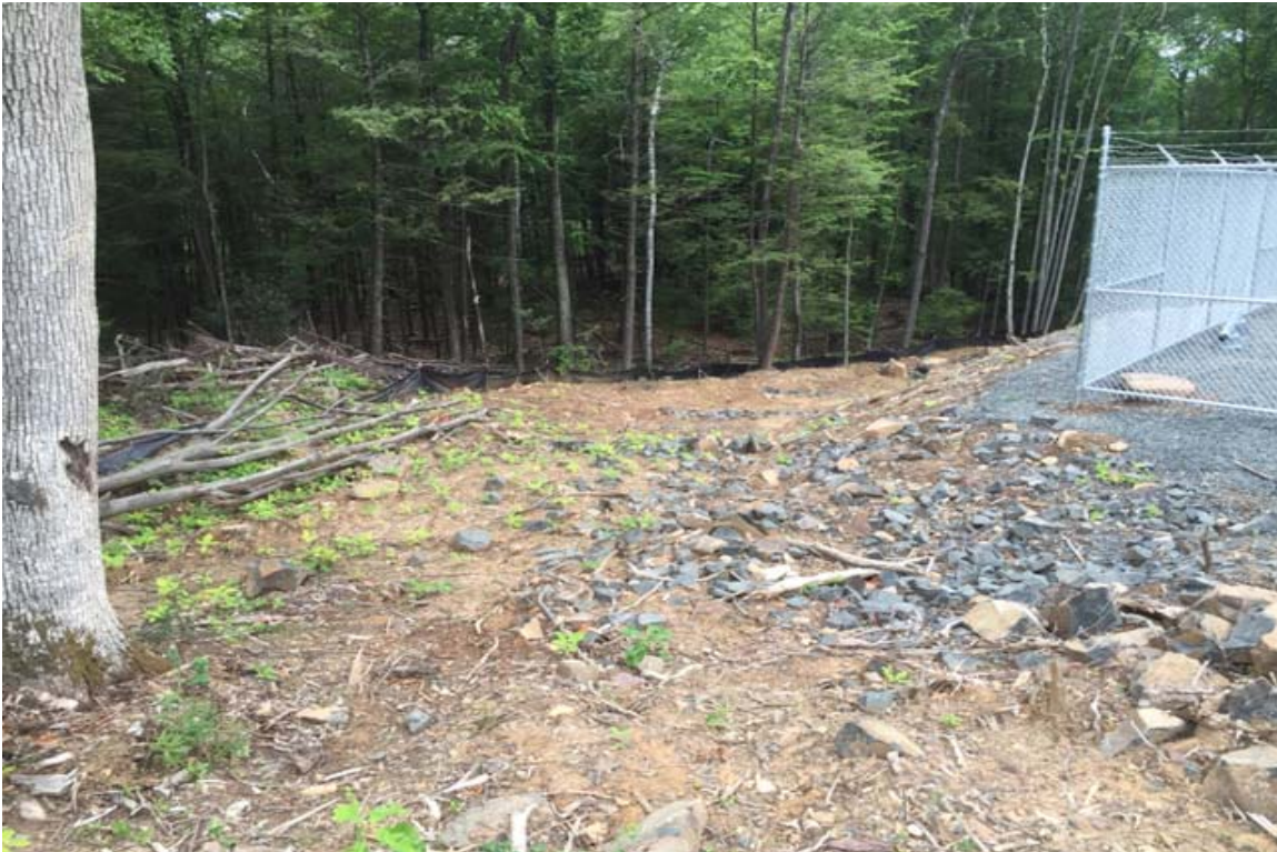
Photo 4: View of south end of drainage swale looking northwest.
