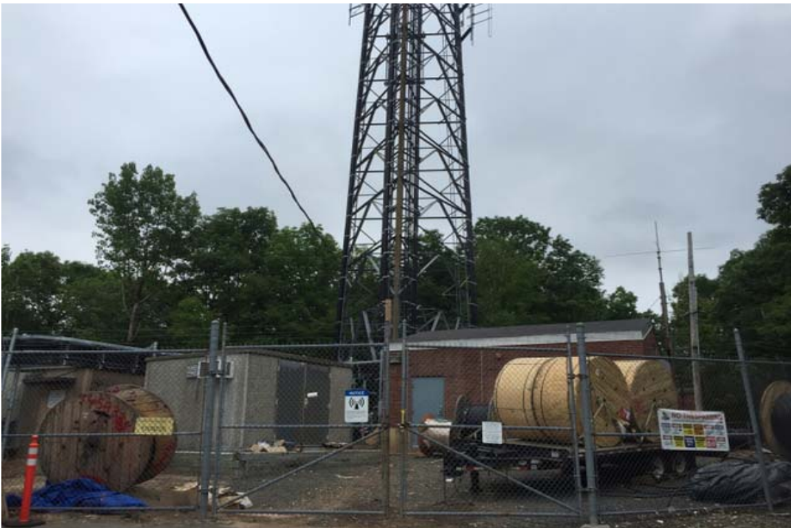
Photo 2: View of existing tower looking north.
