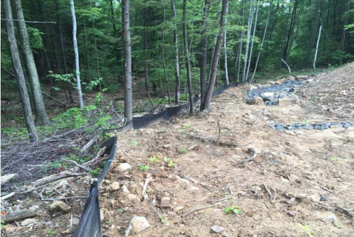
Photo 5: View of silt fence in good condition looking north.
