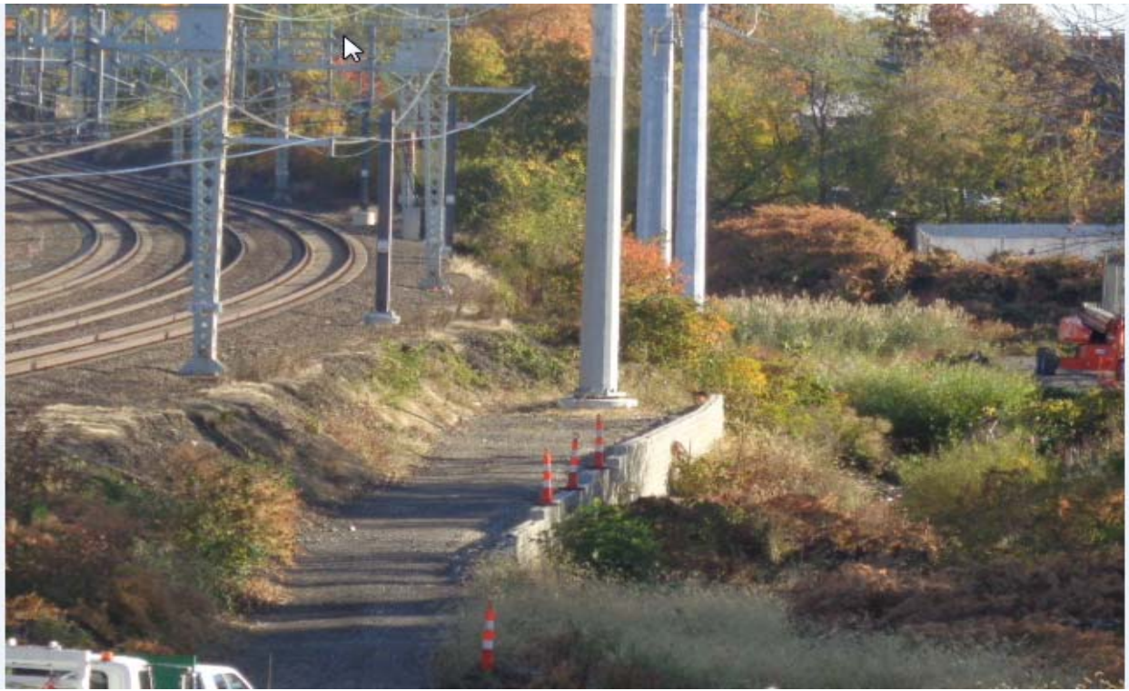
Retaining wall for Structure 886S
