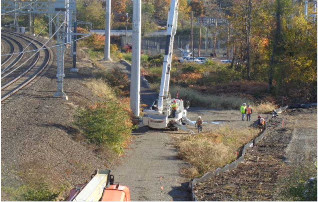
Work pad and access road for Structure(s) 884S, 885S and 886S
