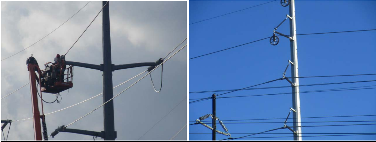
Installing jumpers at structure TP884S and clipping in conductor at 865.
