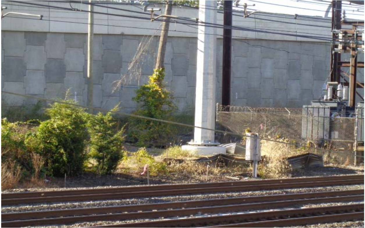
Work pad Structure 867S
