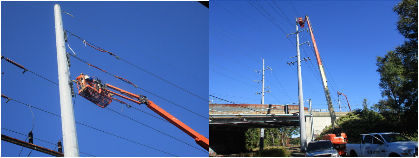
Pressing dead-ends at structure 864BSS and sagging OPGW at TP883S.
