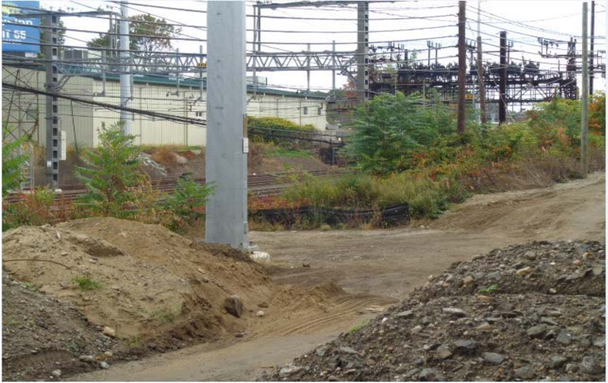
Structure 866S erosion and sediment controls
