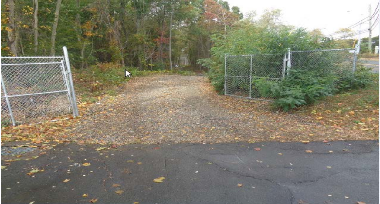
Access Gate and track pad at Structure(s) 882S and 883S
