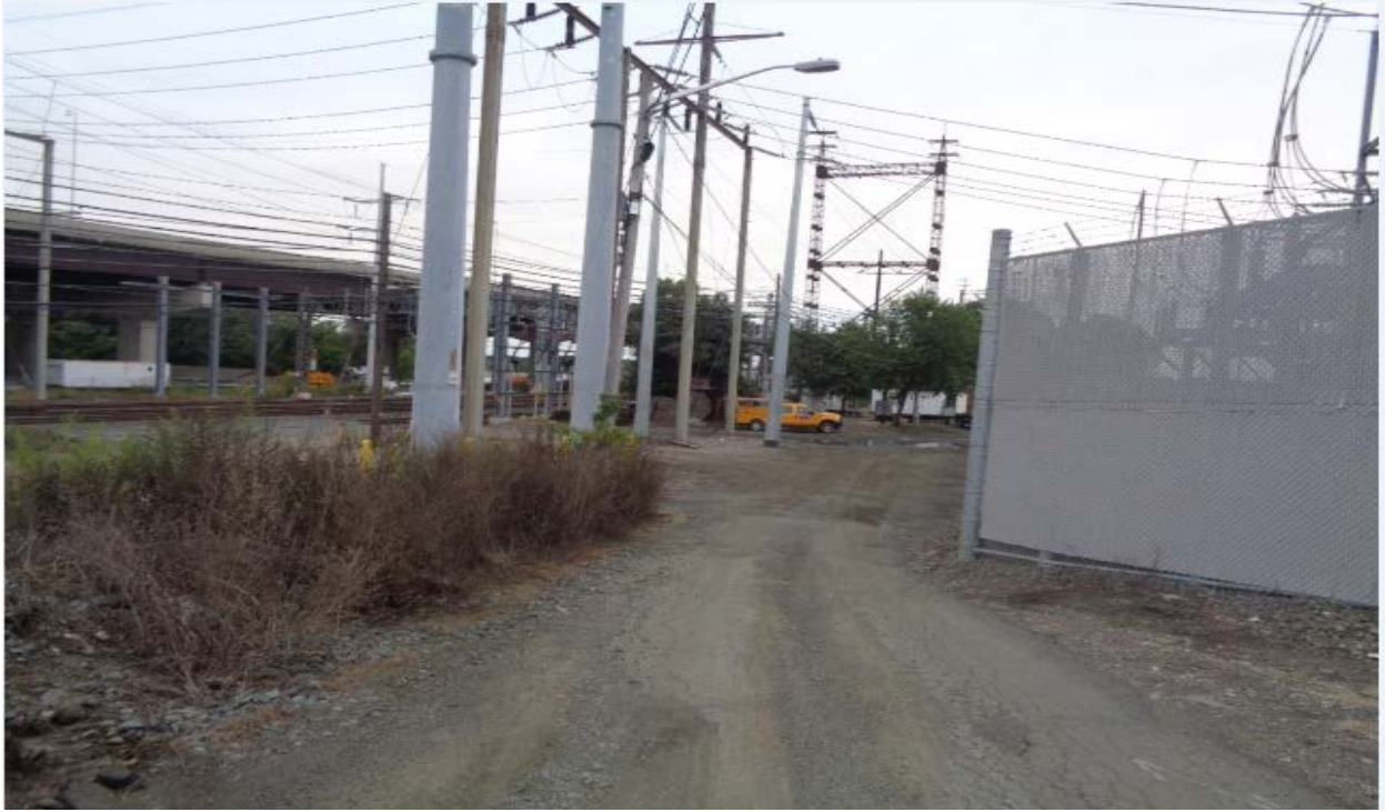
Structure 865S Access Road
