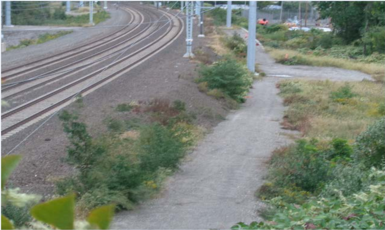
Access Road and Work Pad for Structure 886S
