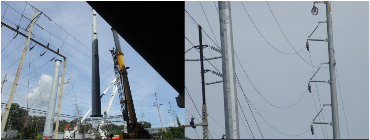
Setting structure 864BSS and installing ropes from structure 865S heading east.
