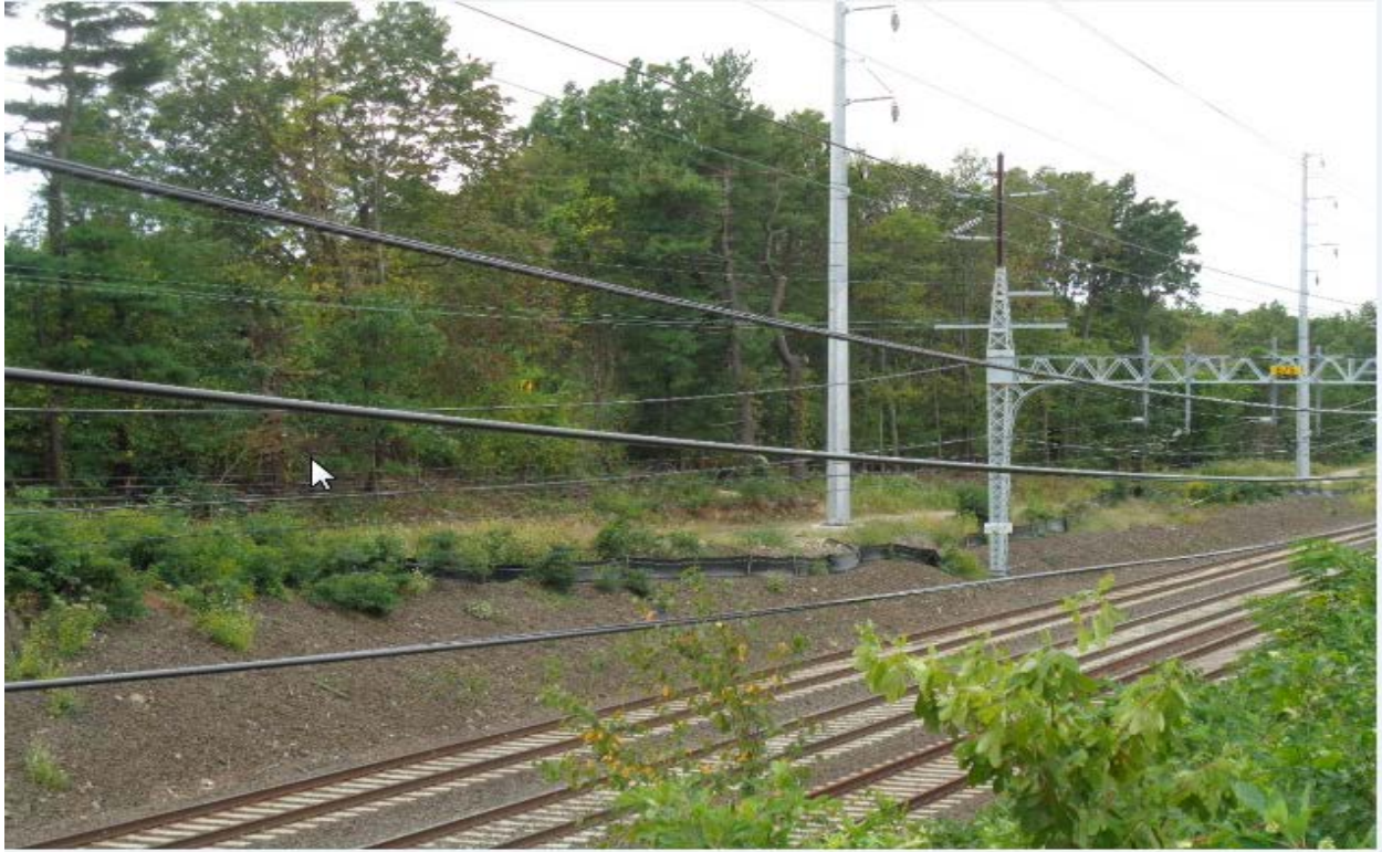
Access Road and Work Area(s) for Structures 873S & 874S
