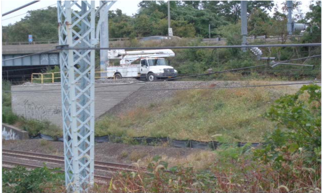
Work Area Structure878S
