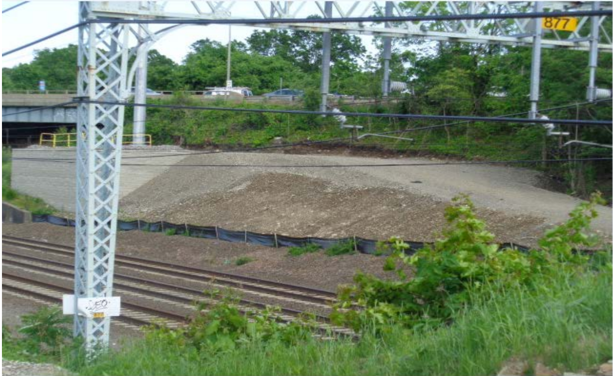
Retaining wall at Structure 878S
