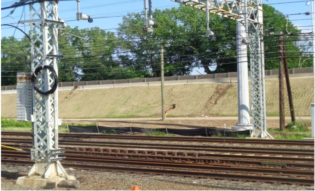
Work pad at Structure 868S
