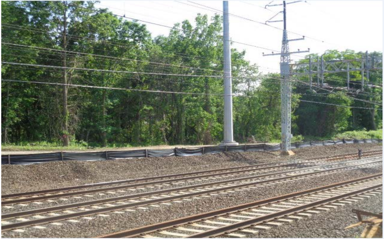
Access road and wok pad at Structure 872S
