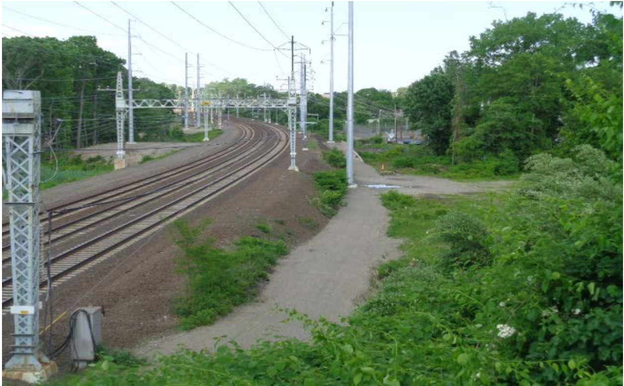
Access road(s) and work pad(s) for Structure(s) 884S and 885S
