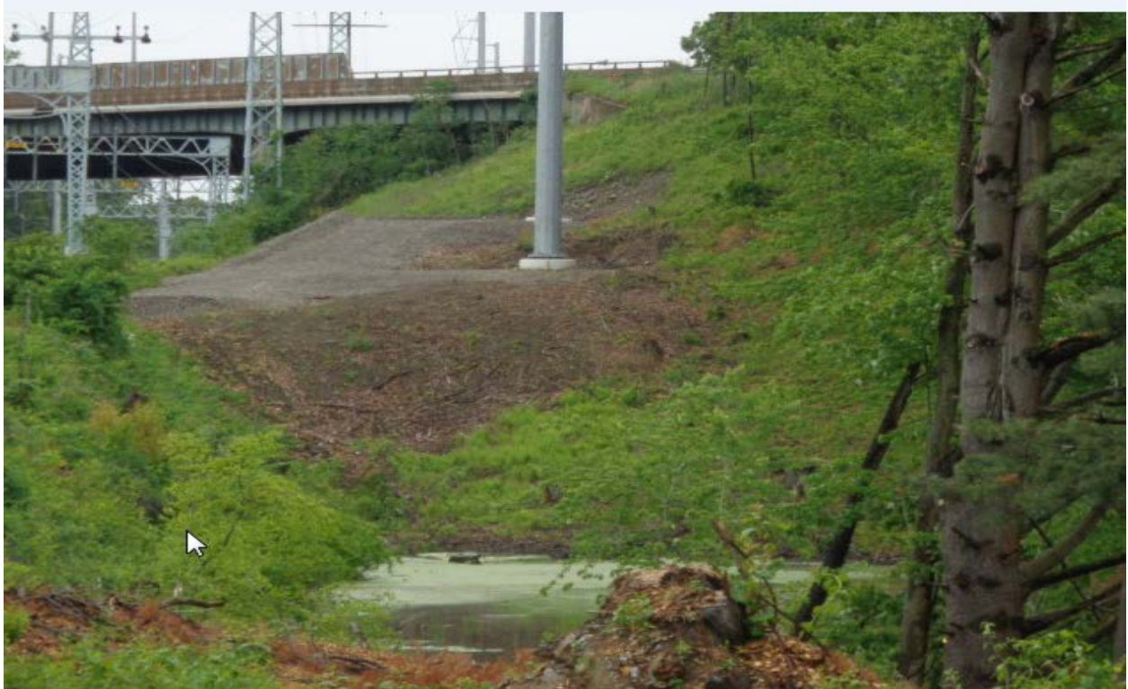
Structure 874S, Access Road, Work Pad and E&S Controls
