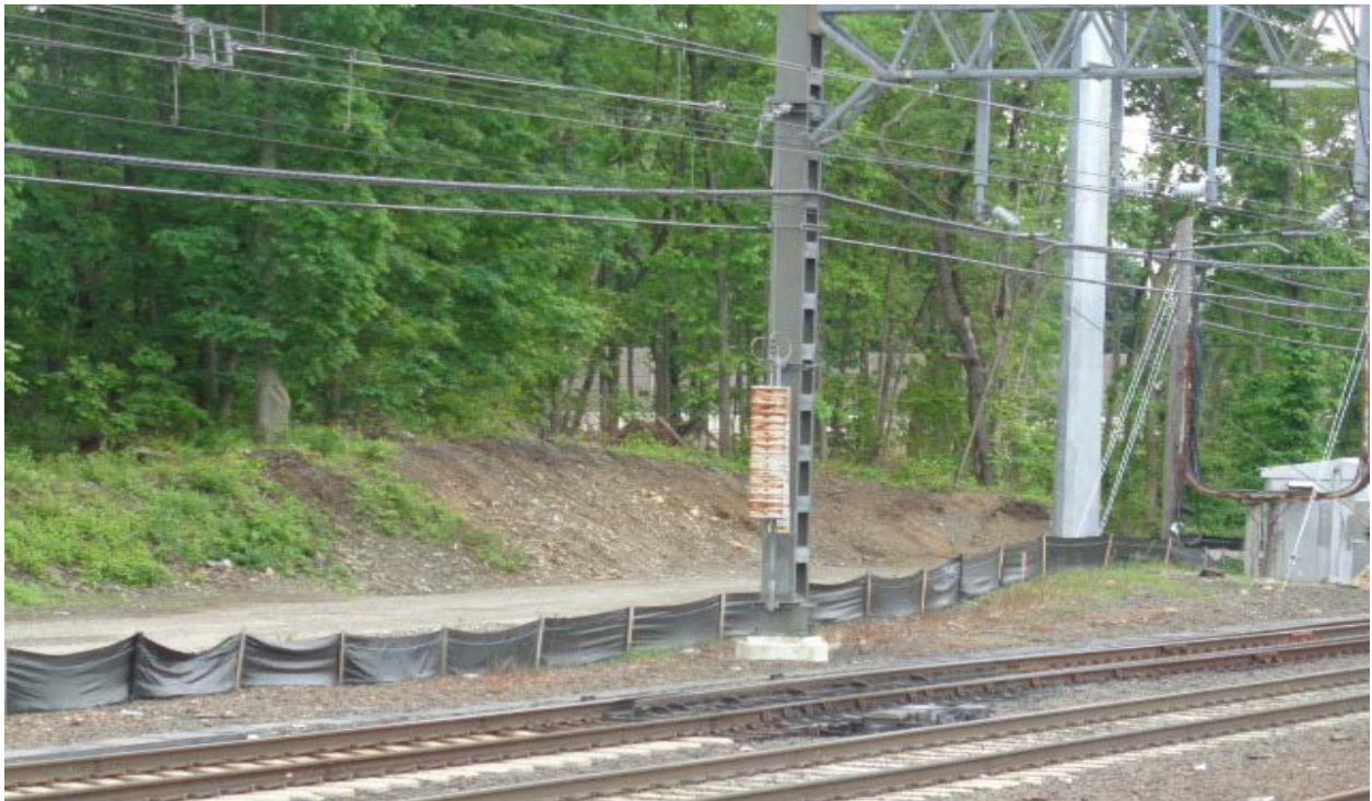
Structure 872S, Access Road, Work Pad and E&S Controls
