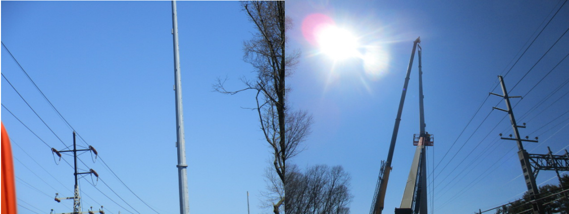
Structure 880S and setting structure 882S
