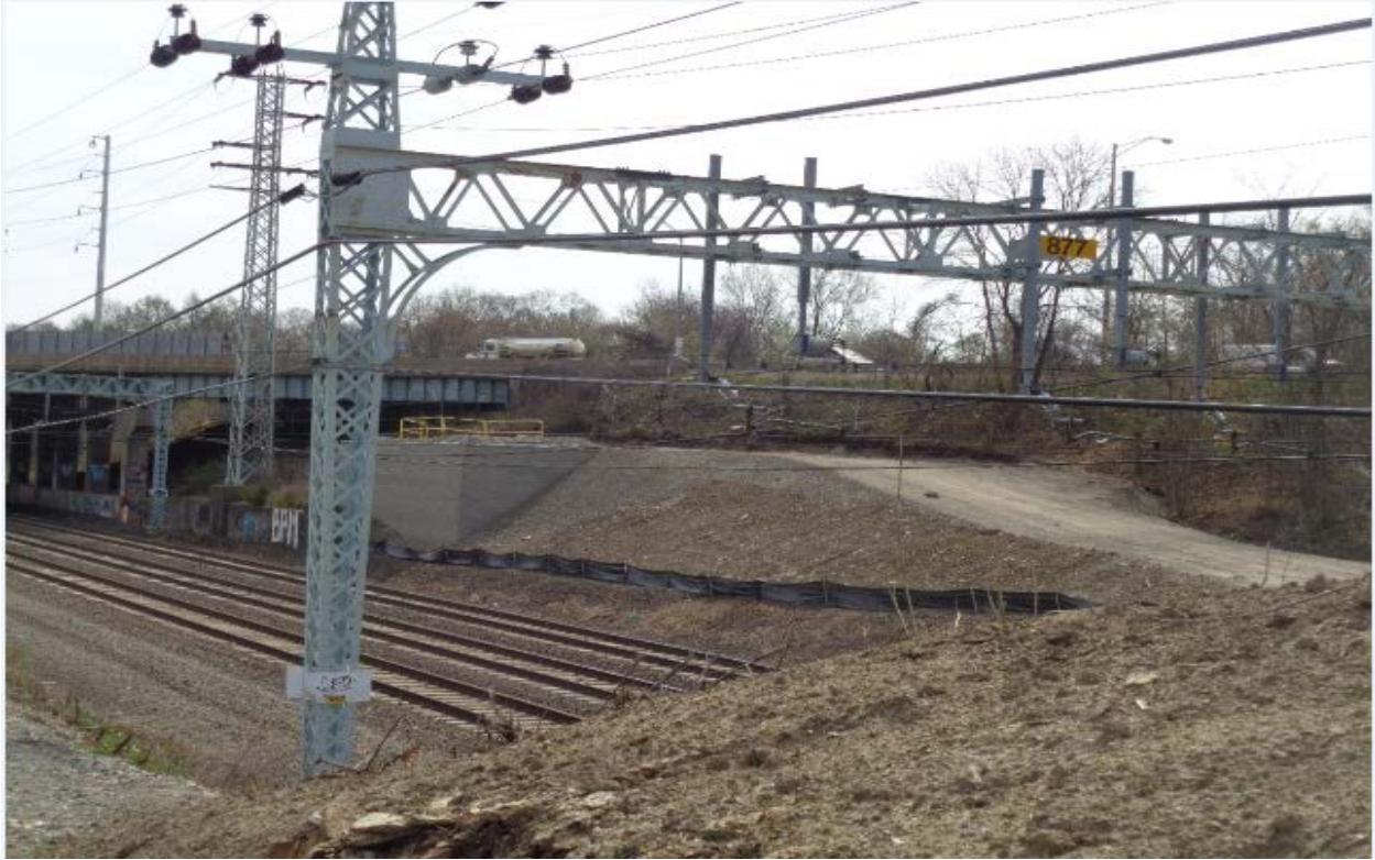
Structure 878S Work Area
