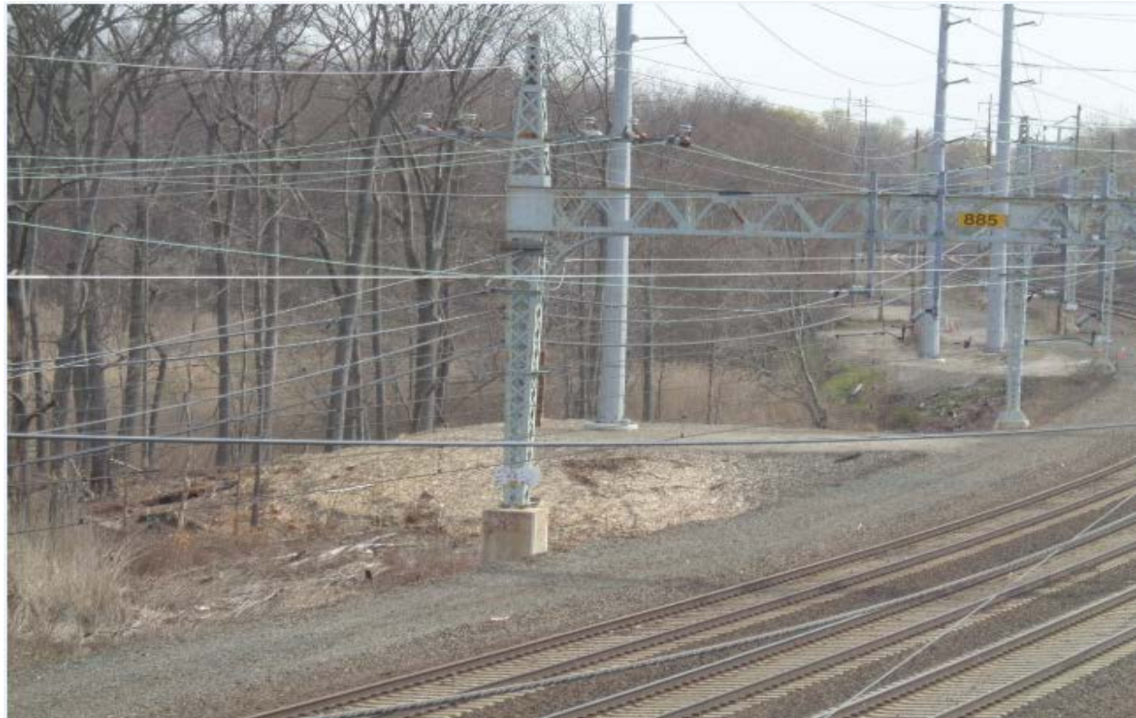
Structure 885S Work Area
