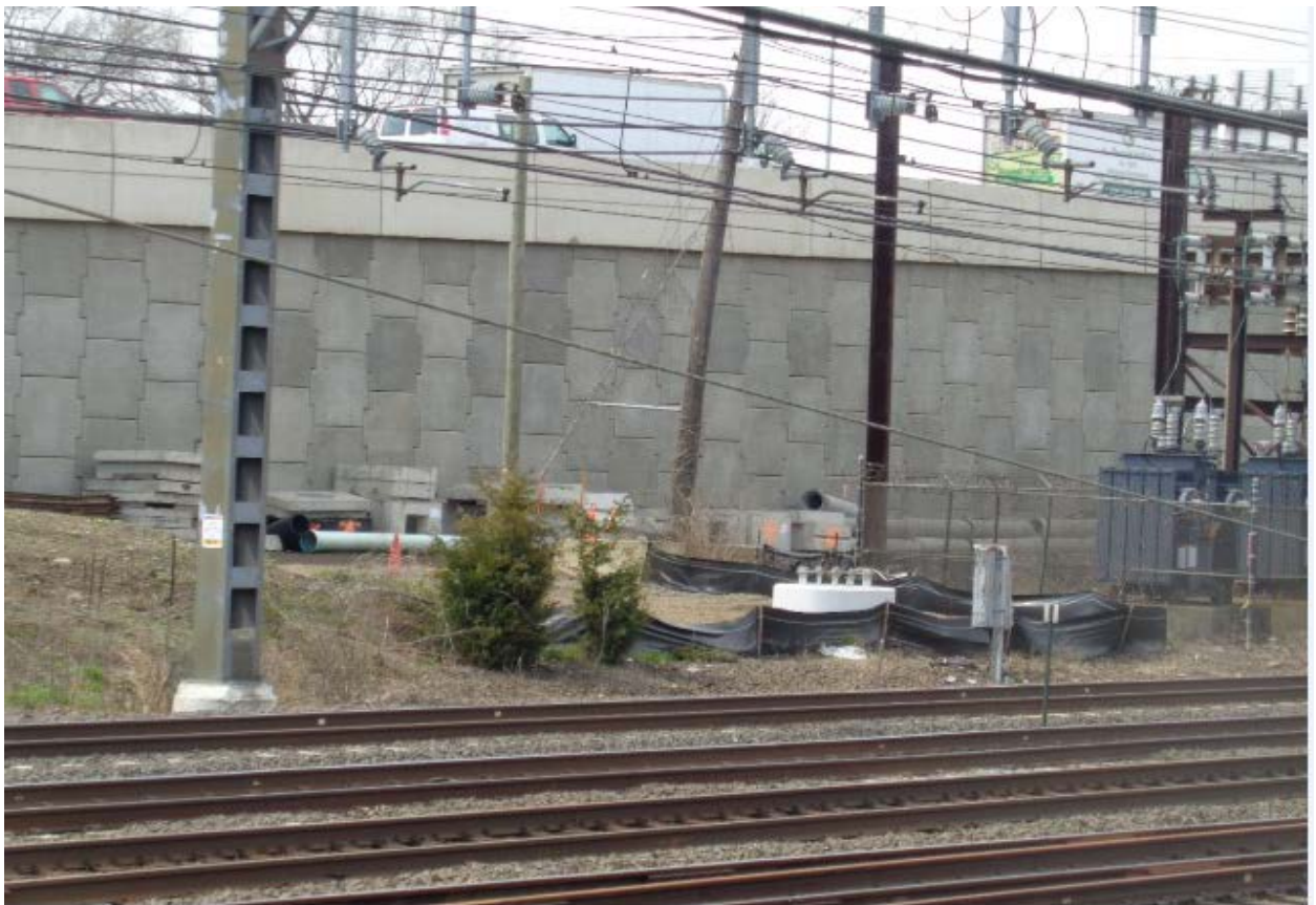
Work pad Structure 867S
