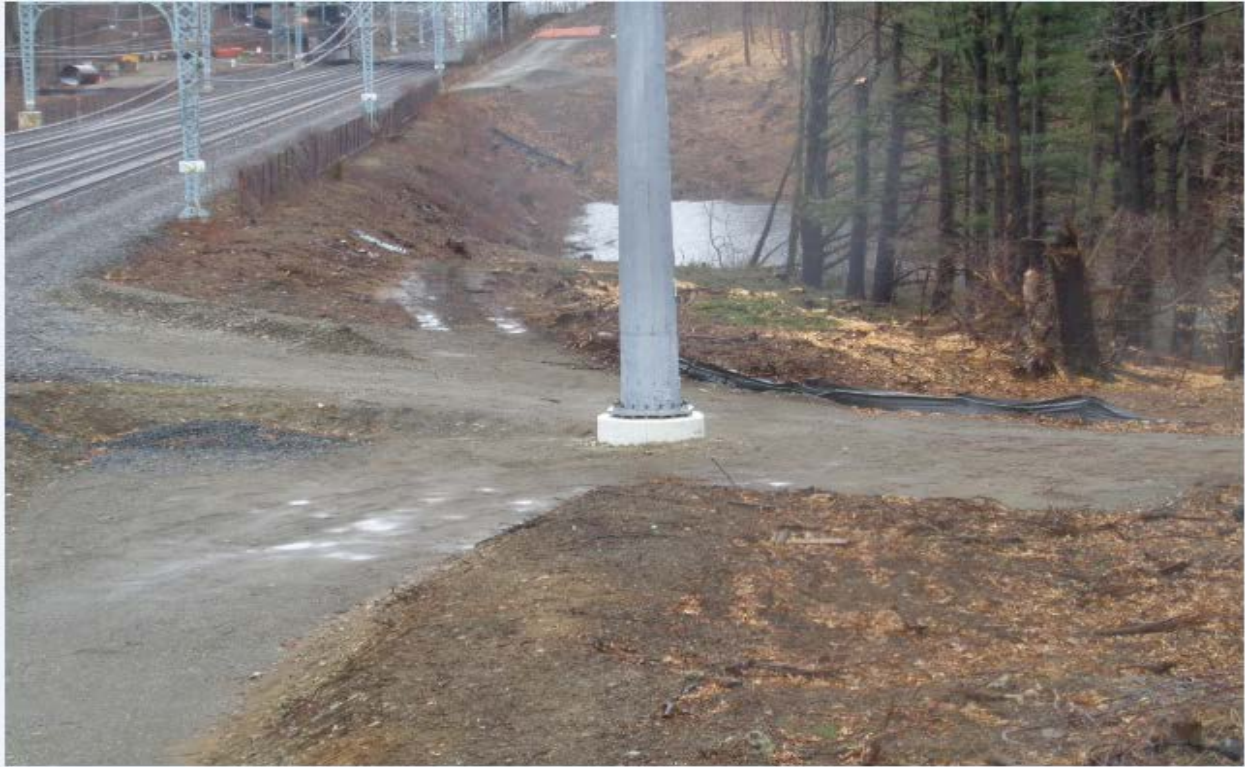
Work area for Structure(s) 882N, 883N and 884N
