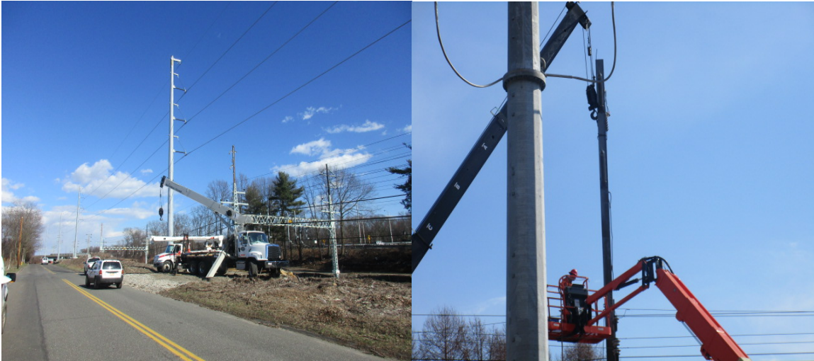
Bonnet removals at Rowe Ave. and Schoolhouse Rd.
