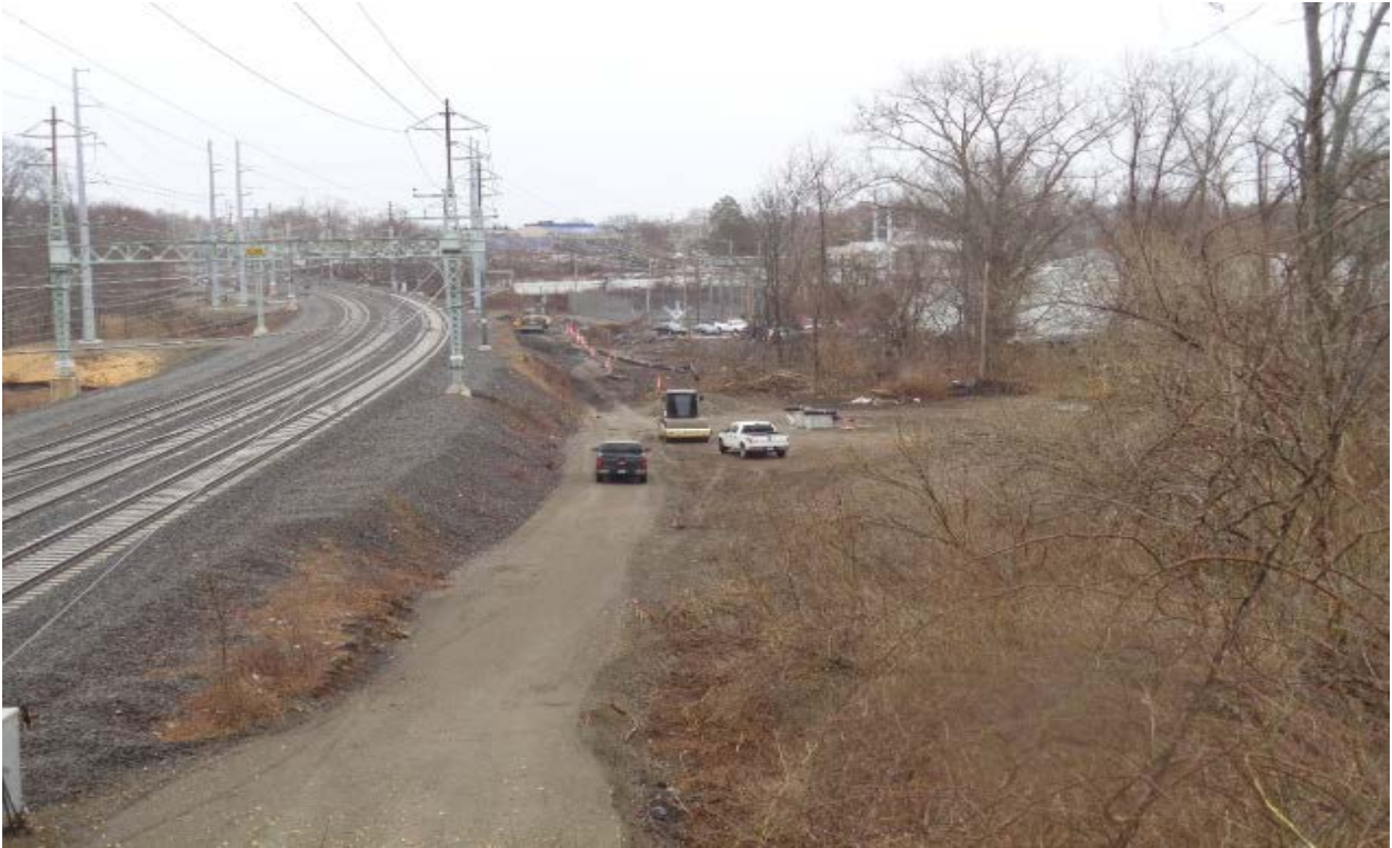
Access Road and Work-pad for Structure(s) 886S & 885S
