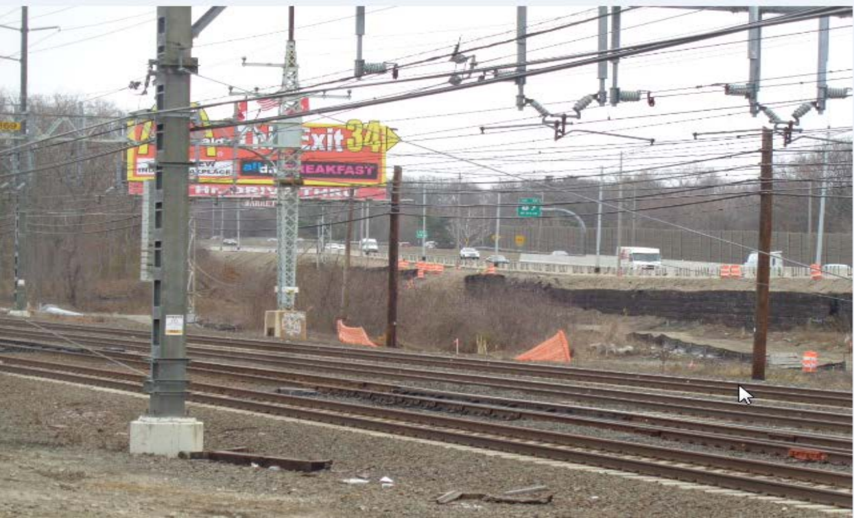
Structure 869S access road
