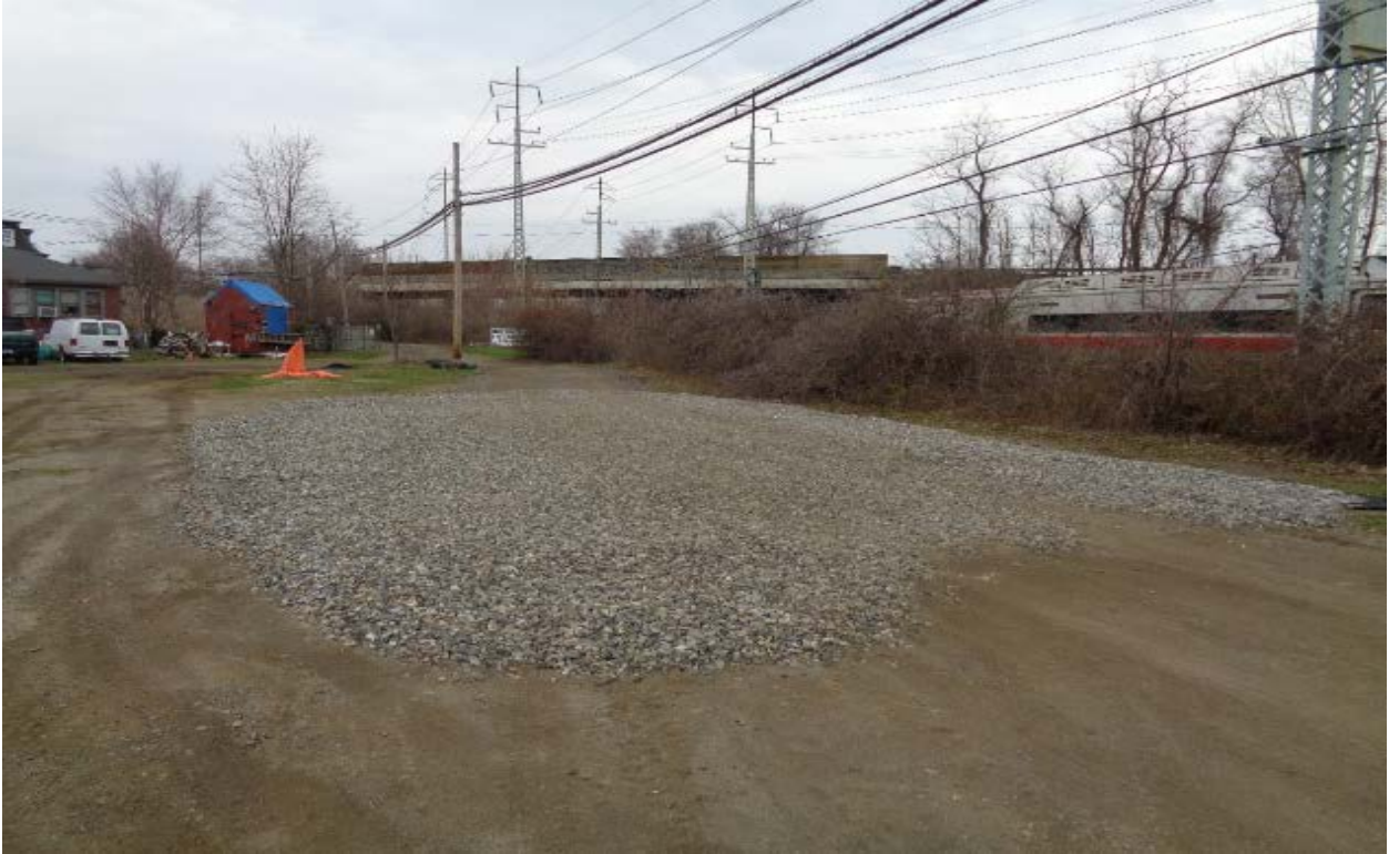
Track-pad for Structure 887N
