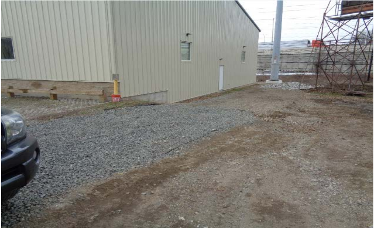
Structure 867N track-pad and access road
