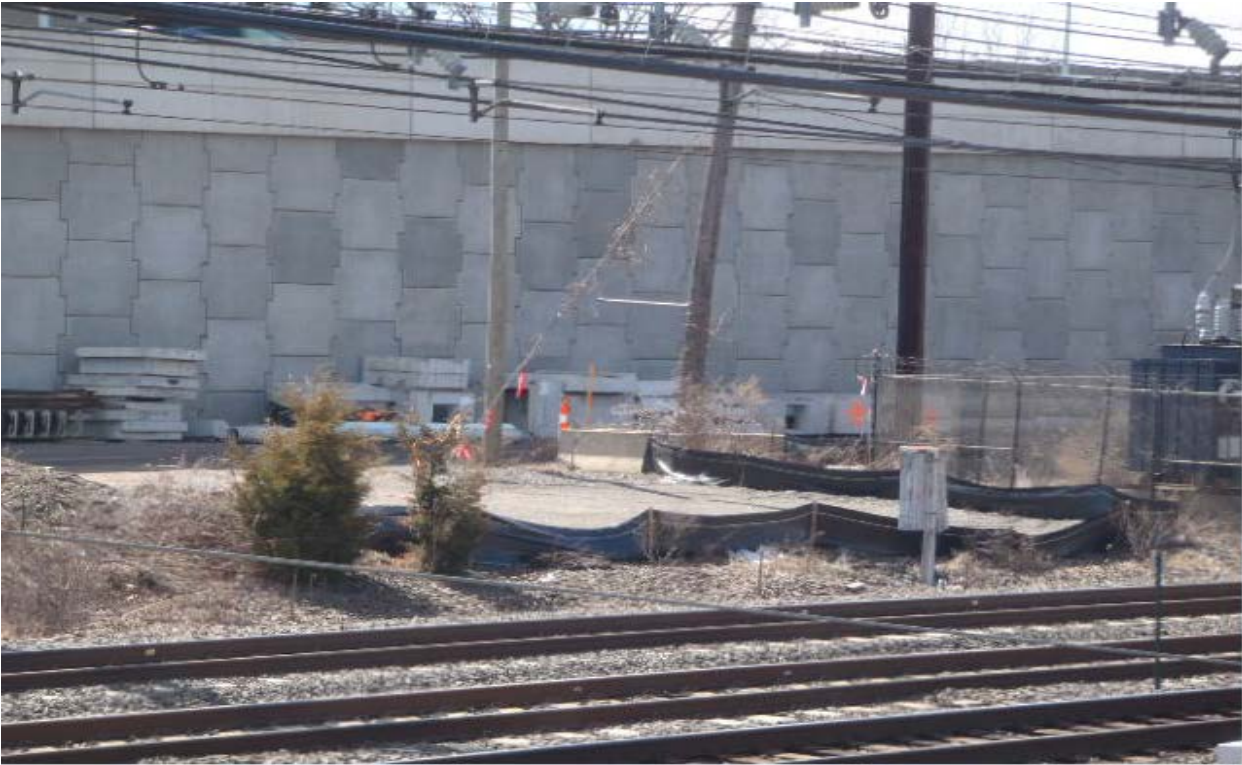
Work pad at Structure 867S
