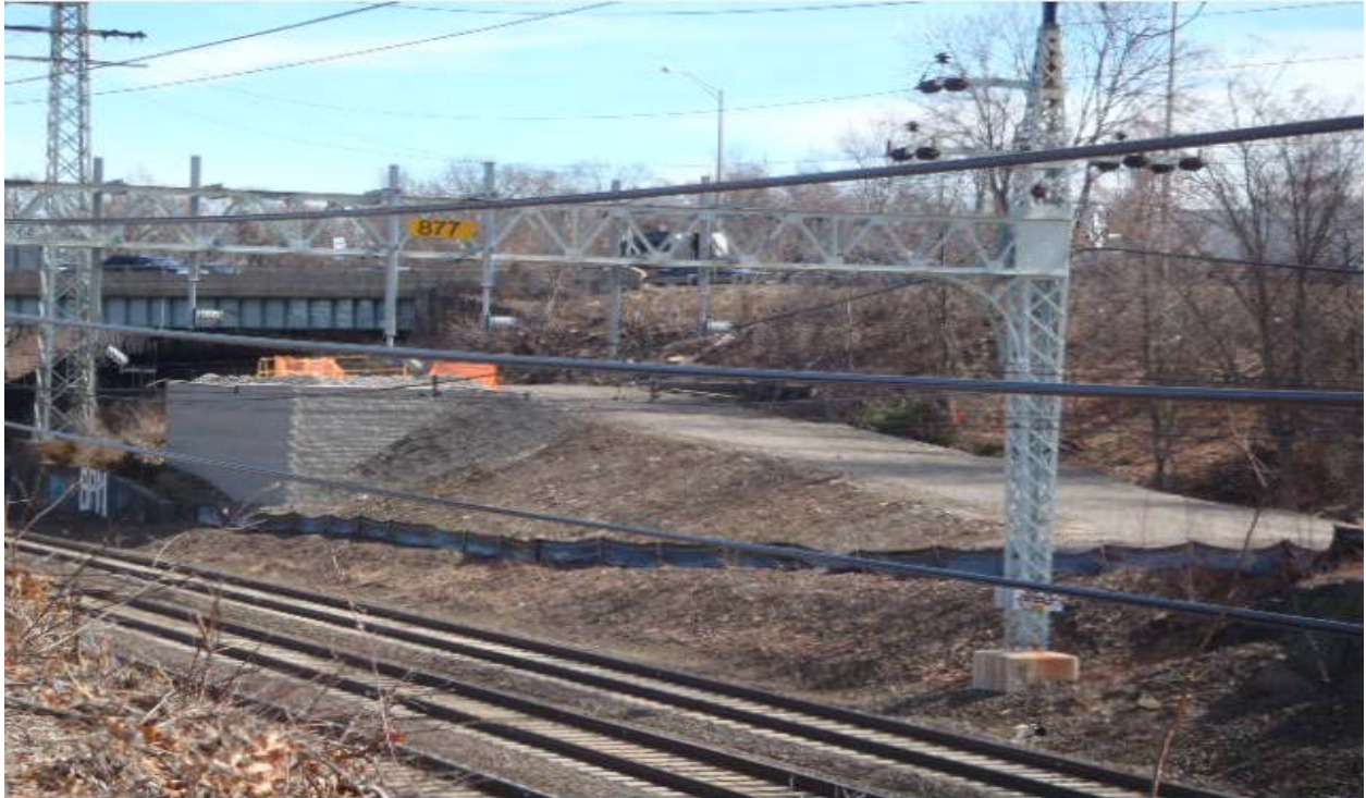
Retaining wall 875S
