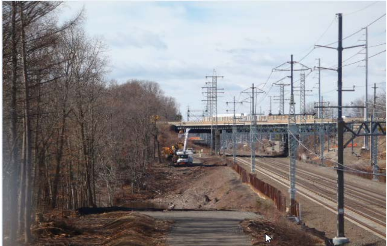
Access road and work pad for Structure(s) 879S and 880S
