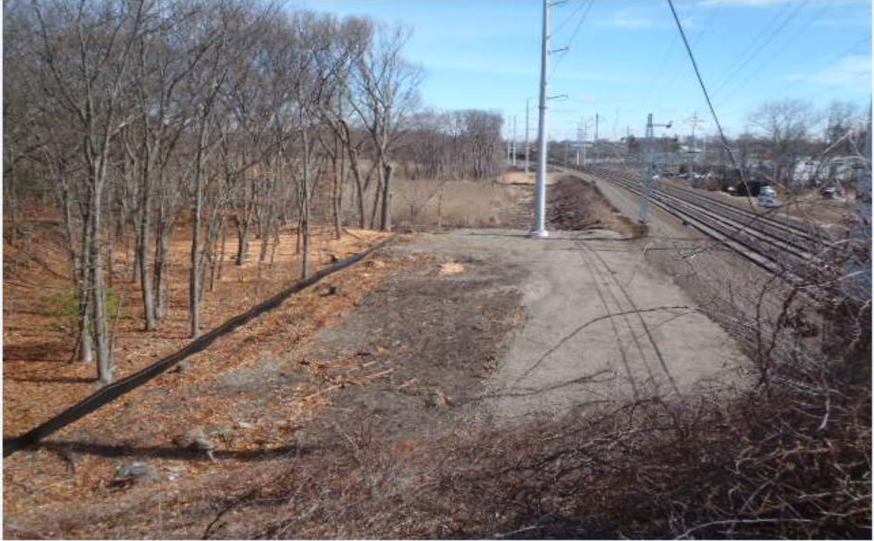
Work pad and erosion and sediment controls at Structure 884N
