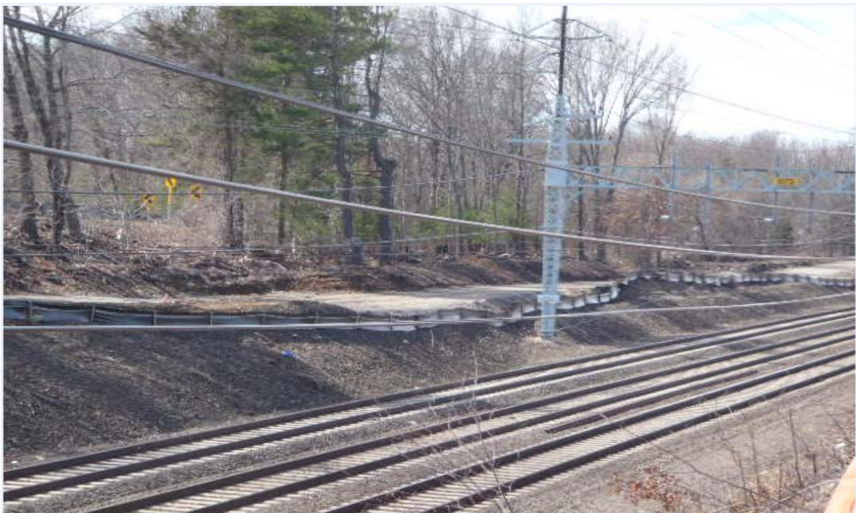
Access road Structure(s) 873S, 874S and 875S
