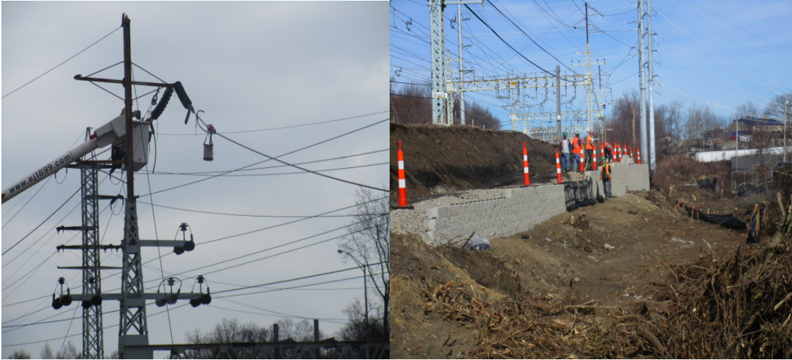
Conductor removal along Rowe Ave., retaining wall being installed at 886S
