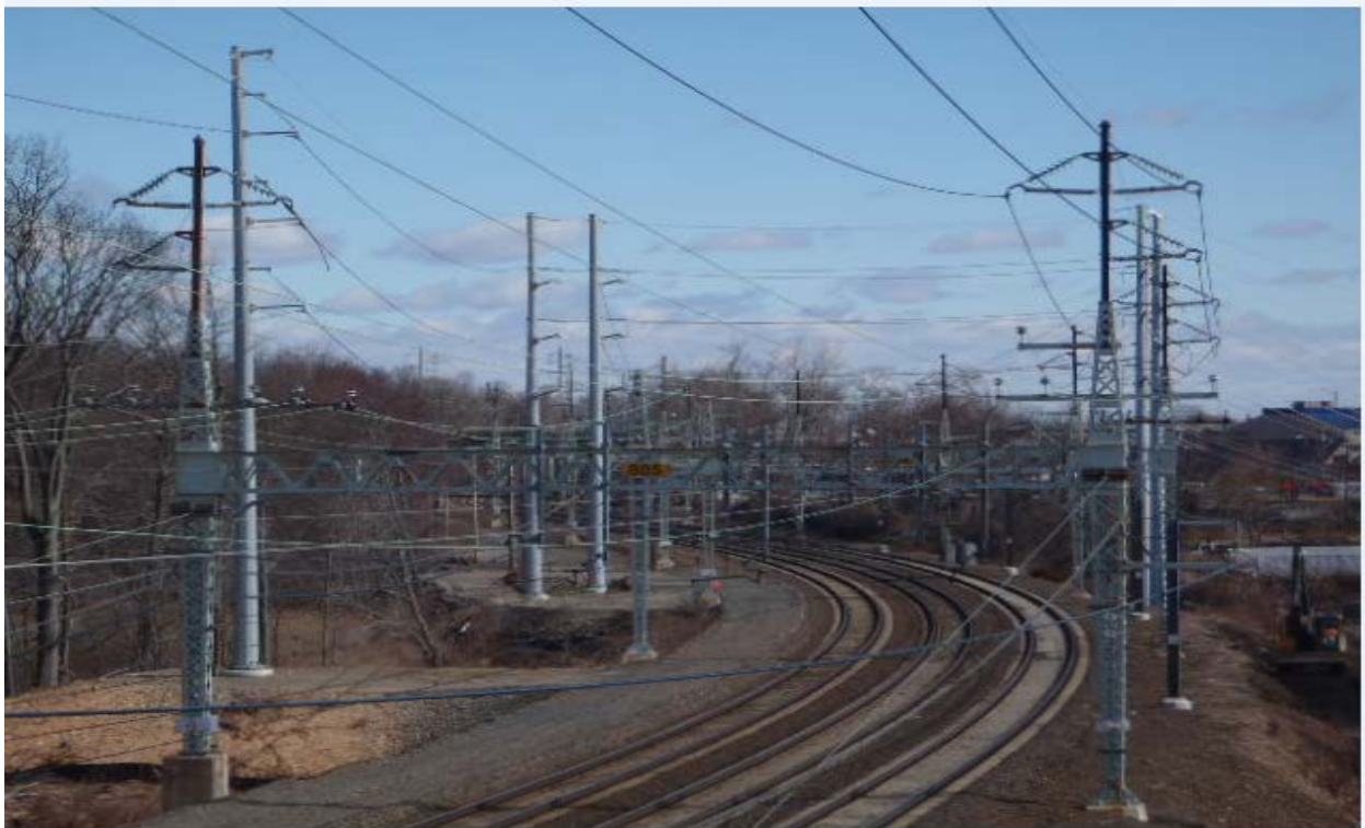
Work area(s) 886N and 887N
