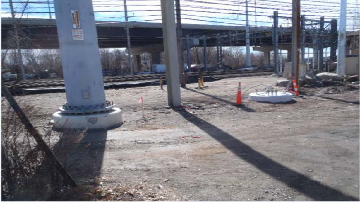
Structure 865N & 866N
