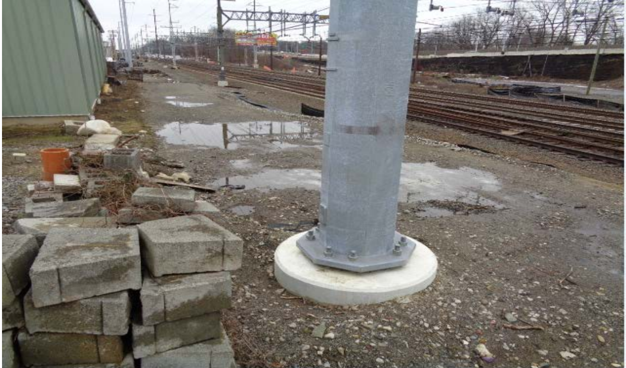
Access road at Structure 868N
