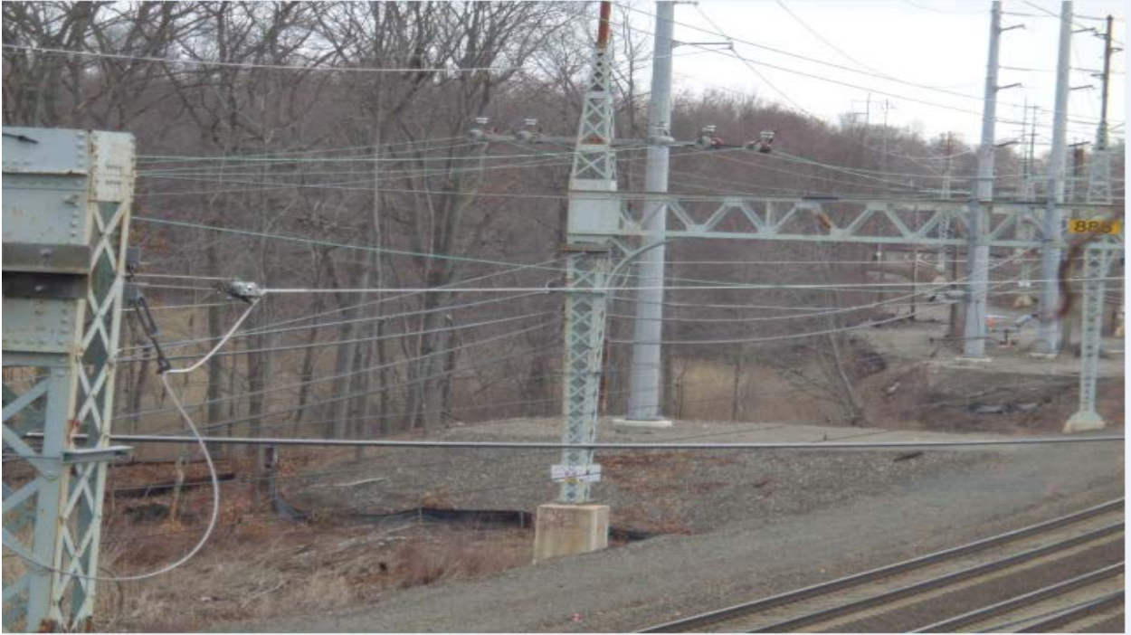
Work pad for Structure 886N
