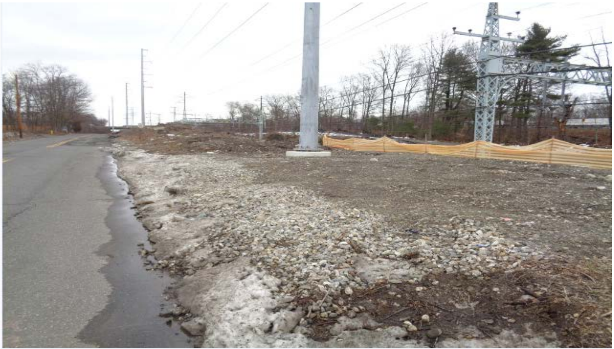
Structure 875N work pad
