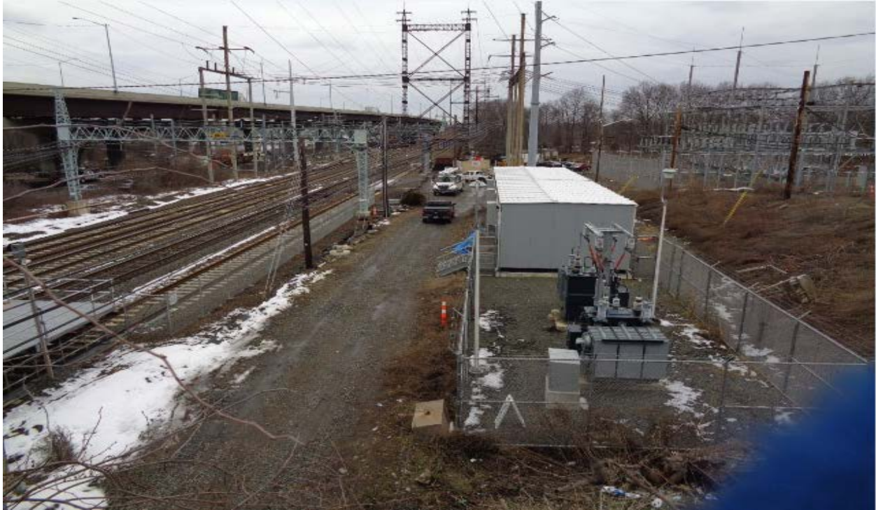
Structure 865N Electrical Work
