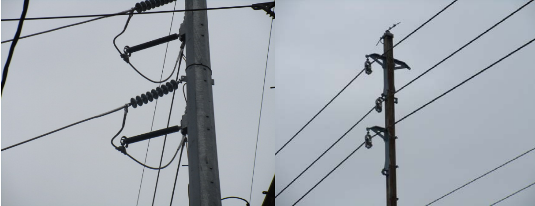
Jumpers installed at 865N, hardware and static wire removed
