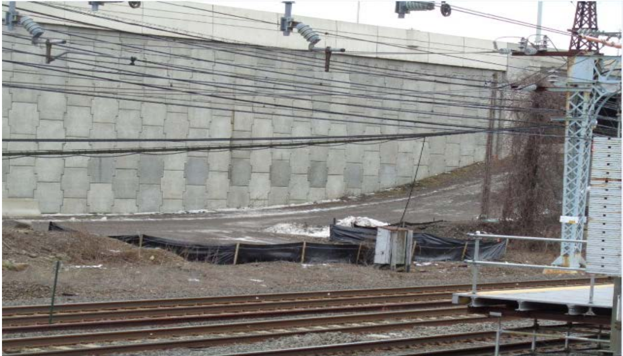
Erosion and sediment controls and work pad at Structure 866S
