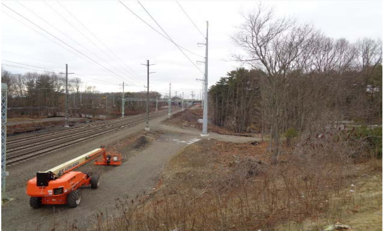
Access road and work pad for Structure 882N
