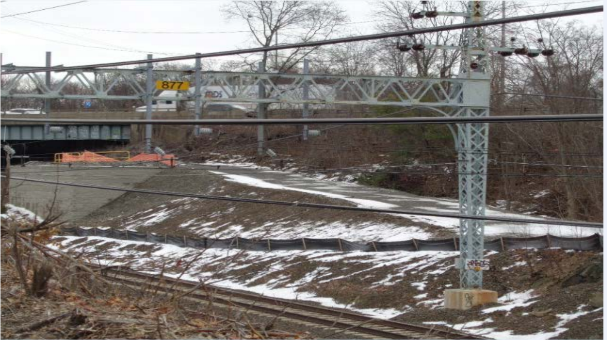
Structure 877S work pad, retaining wall
