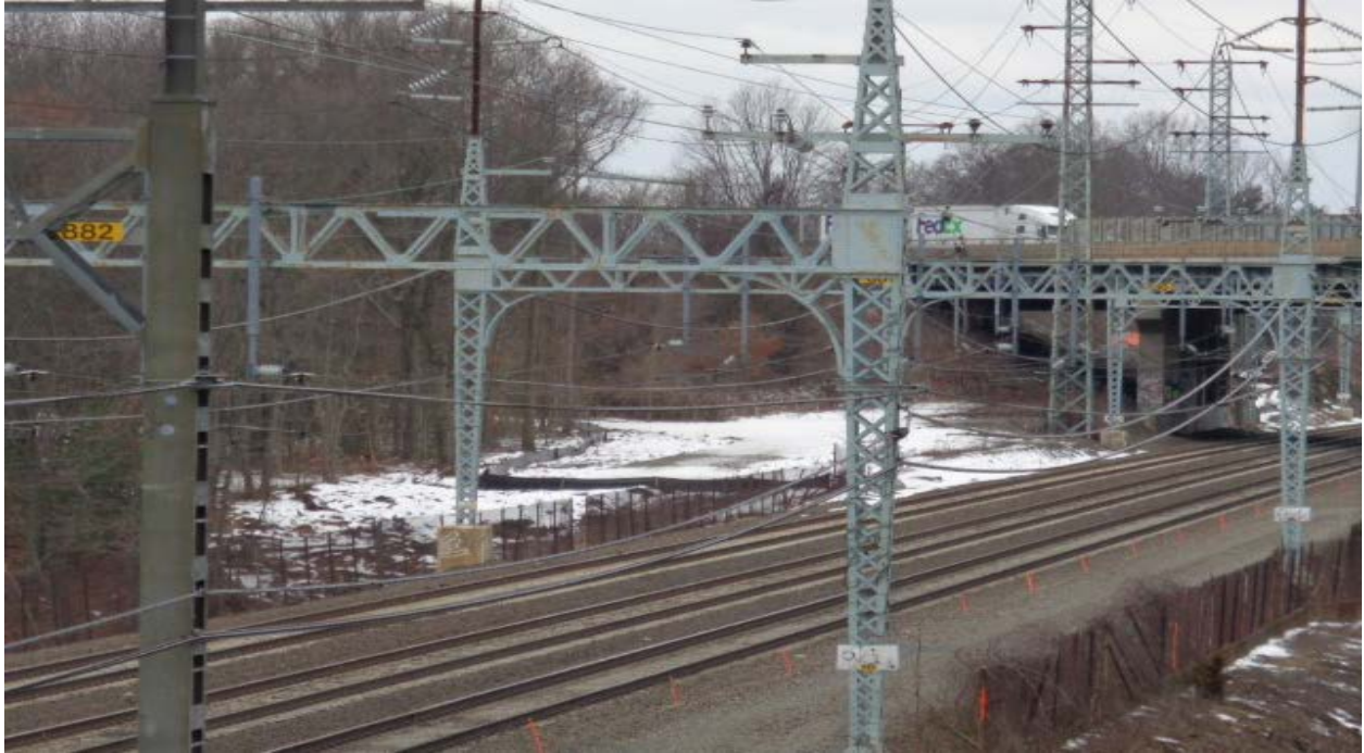
Work pad Structure 881S
