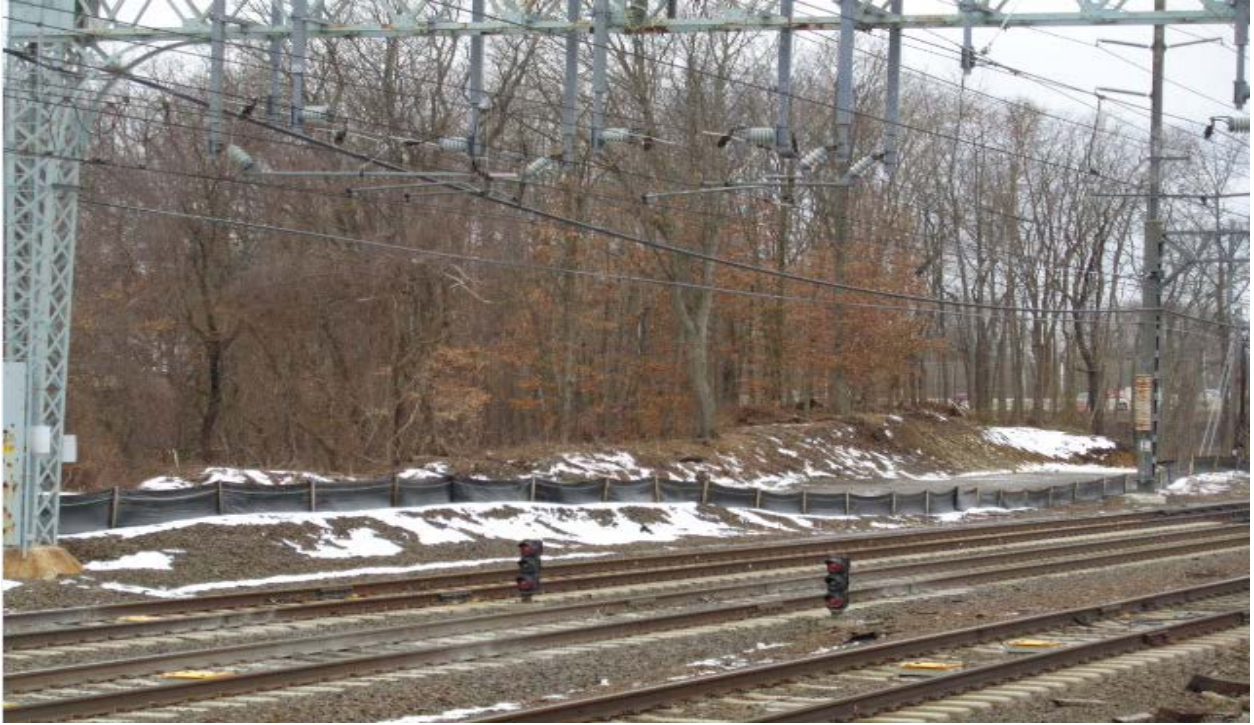
Access road and erosion and sediment controls between 871S and 872S
