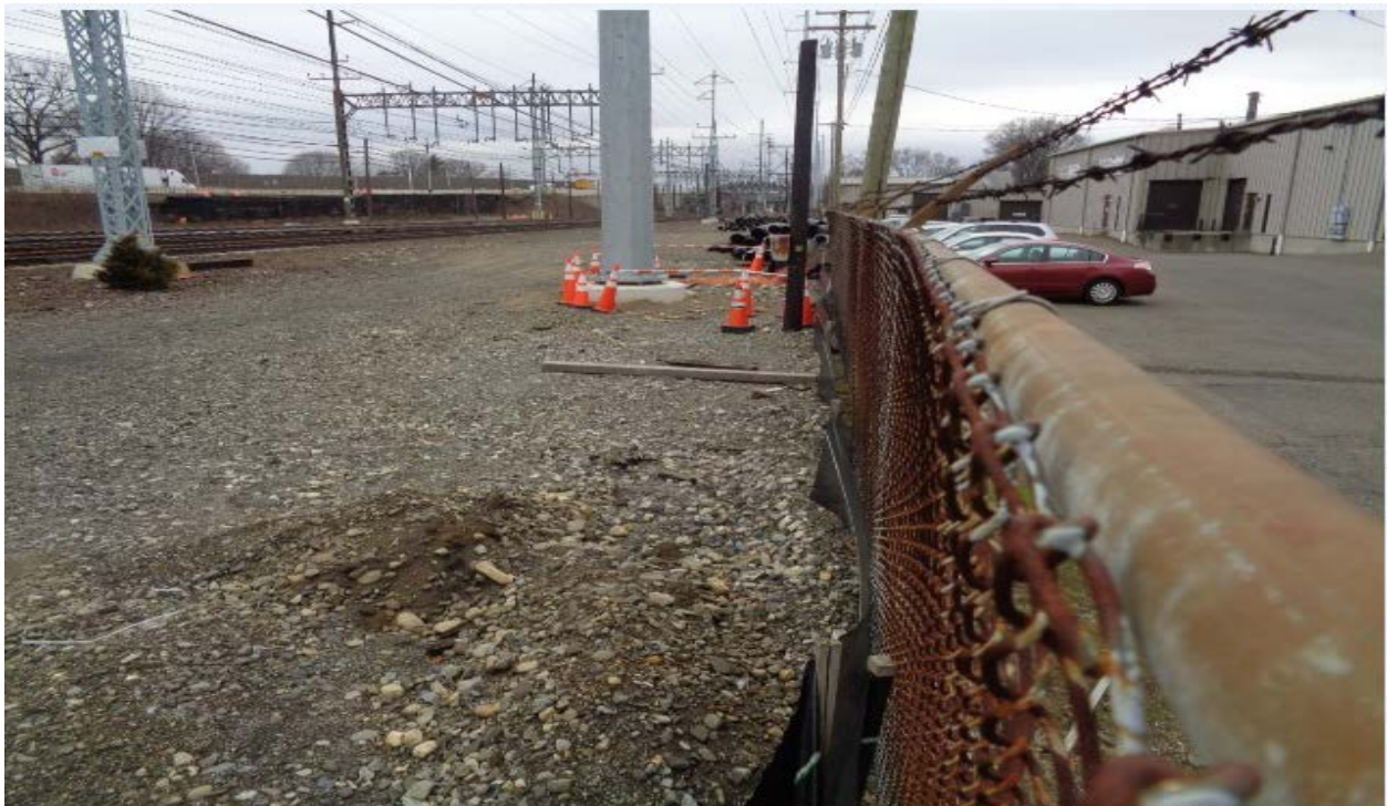
Access road and erosion and sediment controls at Structure 870N
