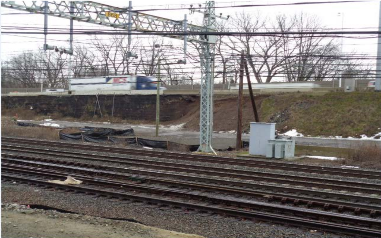
Work pad at Structure 868S
