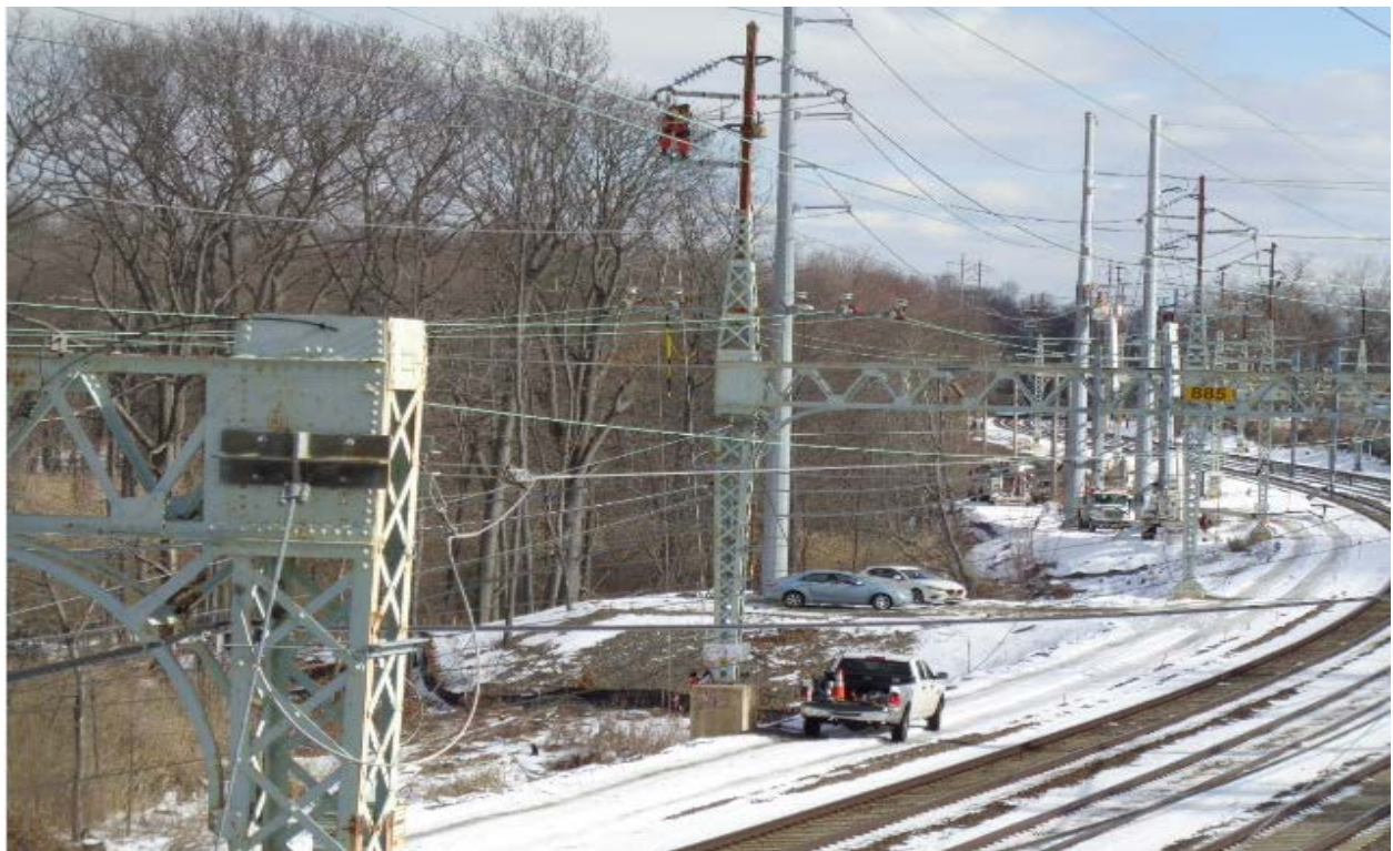
Structure(s) 885N & 886N Work pads
