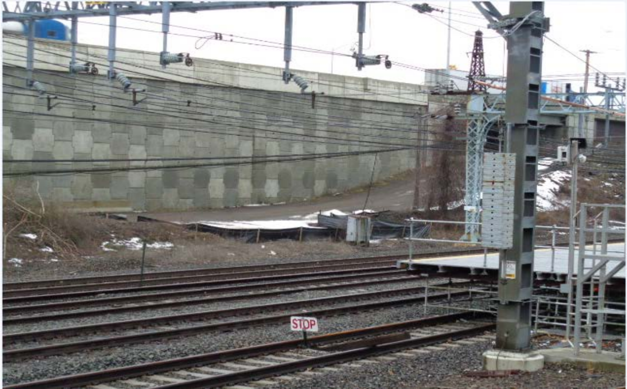
Erosion and sedimentation controls along access road for 866S
