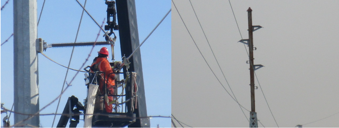
Clipping conductor at structure 879N, exiting conductor and hardware removed
