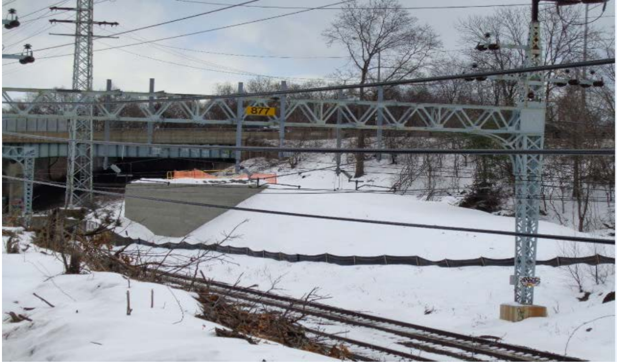
Structure 877S retaining wall and erosion and sediment controls
