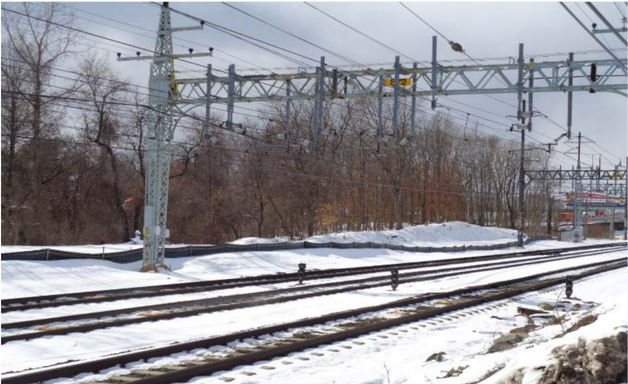
Access road, work pad and erosion and sediment controls for Structure(s) 871S & 872S
