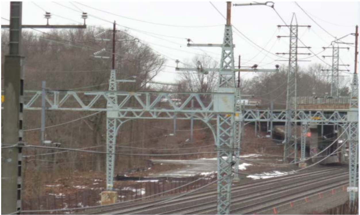
Structure 879S Work pad
