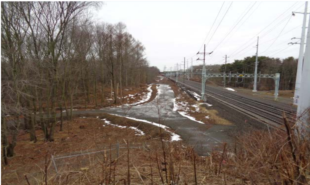
Access road and work pad construction at Structure(s) 882S & 883S
