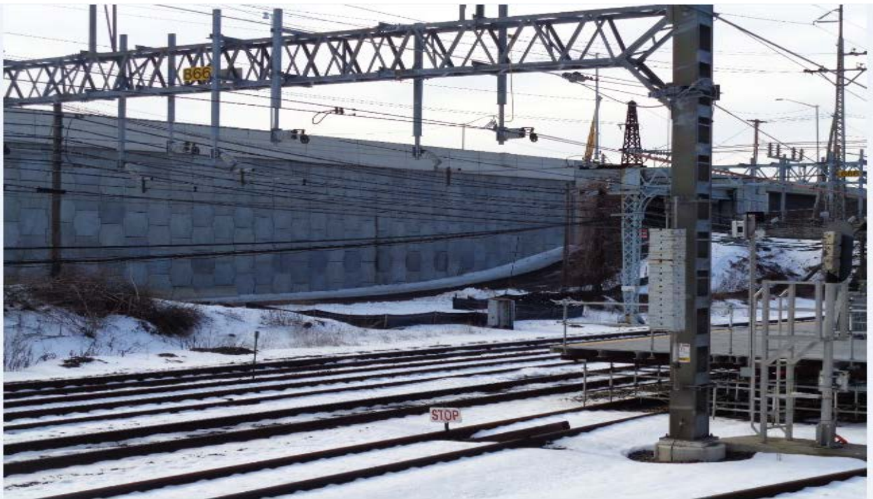
Structure 866S sediment and erosion controls
