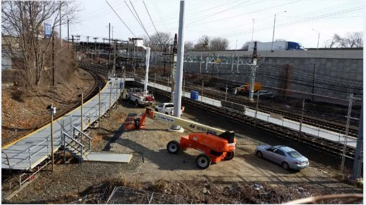
Stringing at Structure 866N
