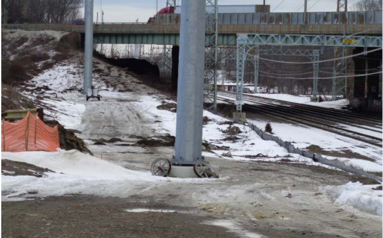
Access road Structure 877N-878N
