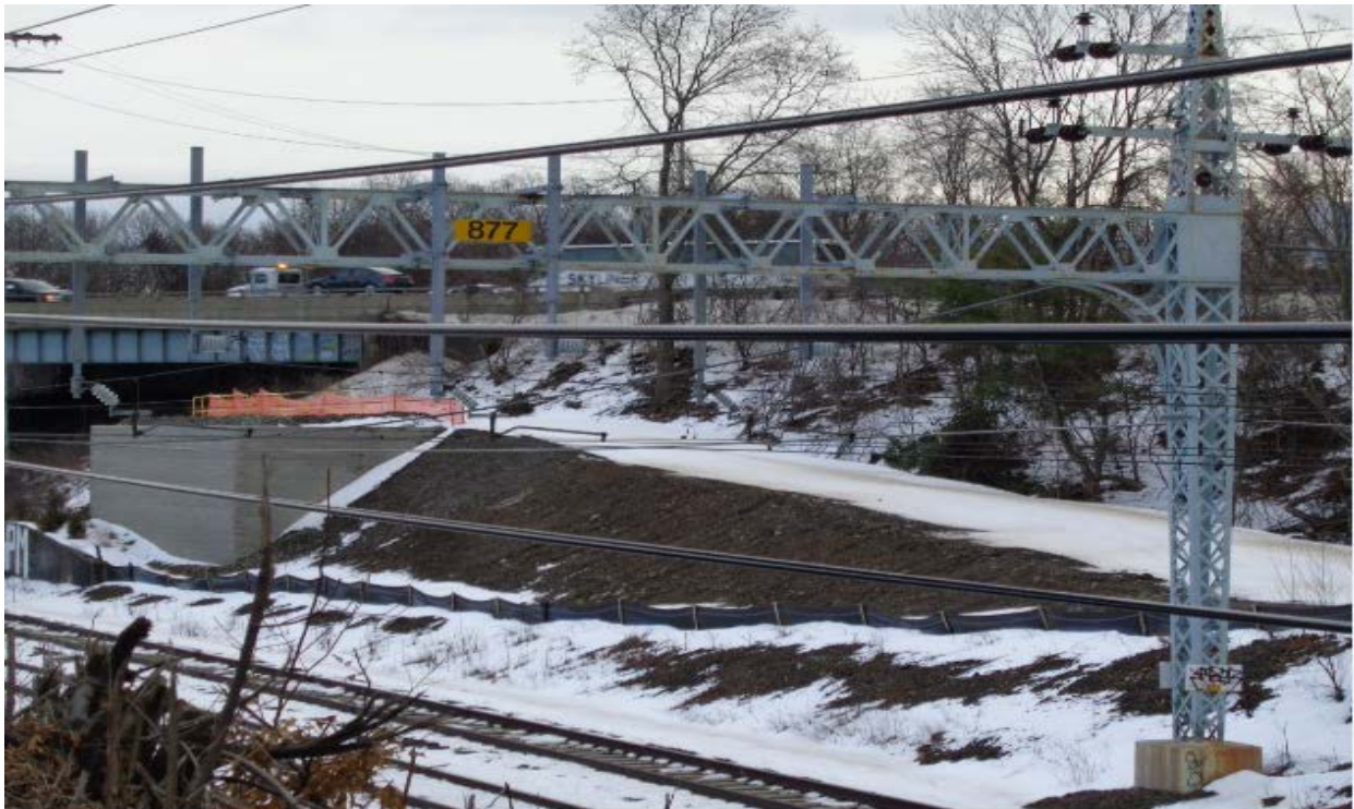
Structure 877S access road, work pad, sediment and erosion controls
