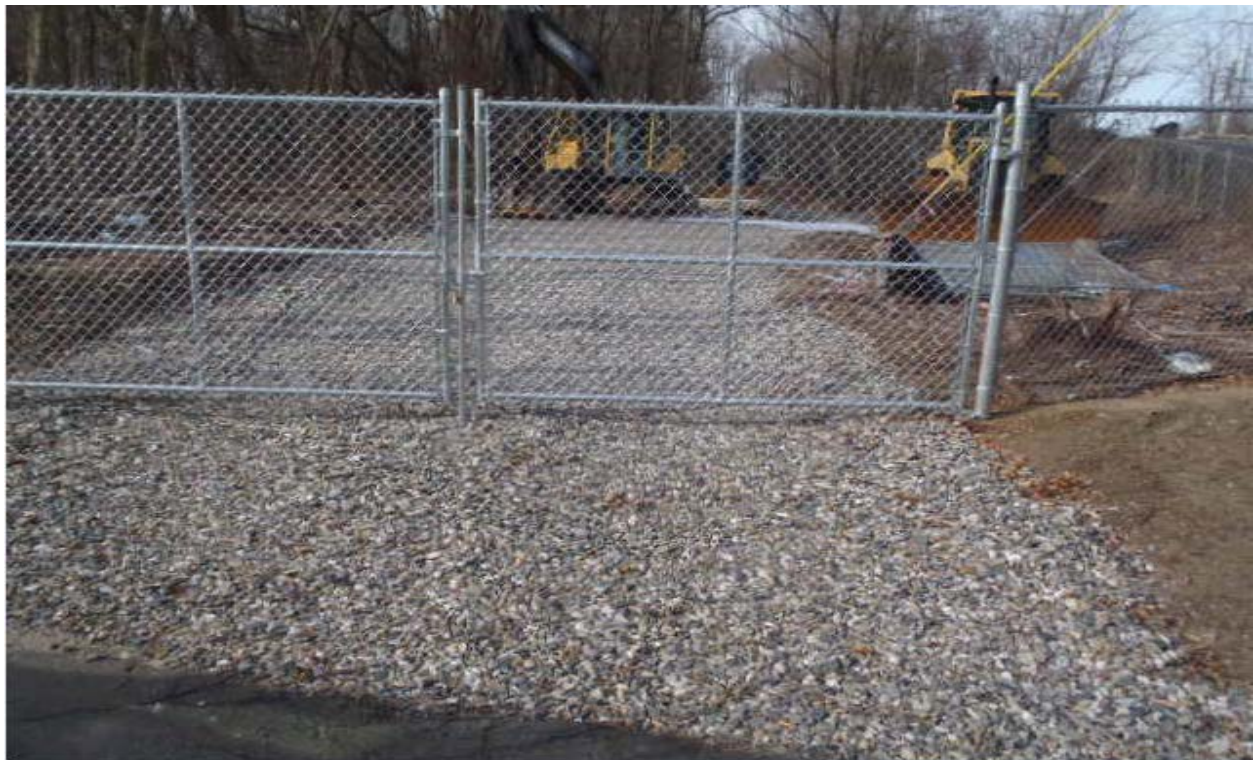
Access road entrance at Structure 882S and 883S
