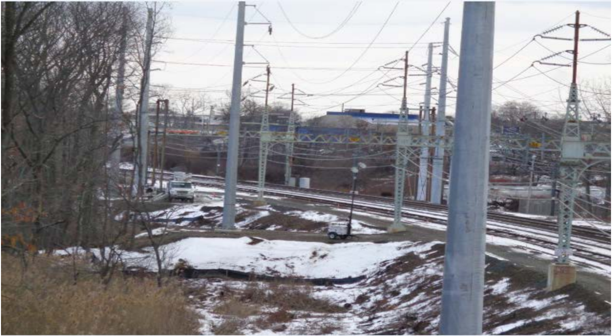
Structure 886N work pad and sediment and erosion controls
