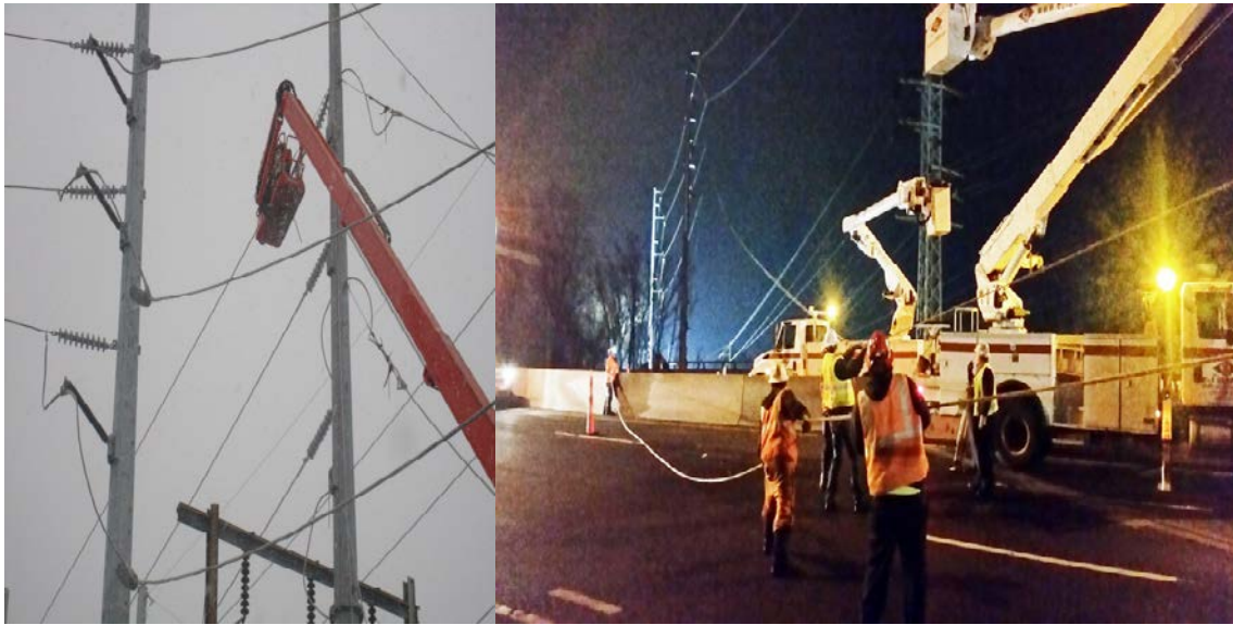
Conductors installed across the 4-tracks and rope installation across I-95
