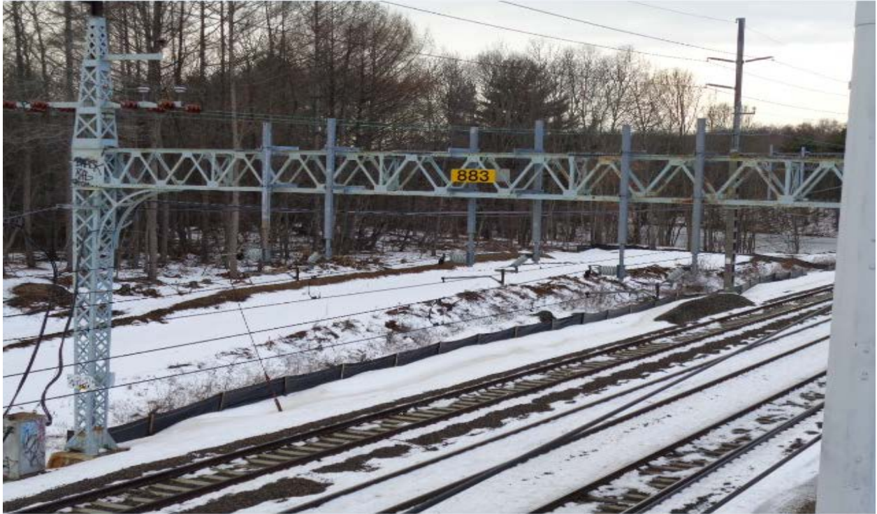
Structure 882S and 883S access road, sediment and erosion controls
