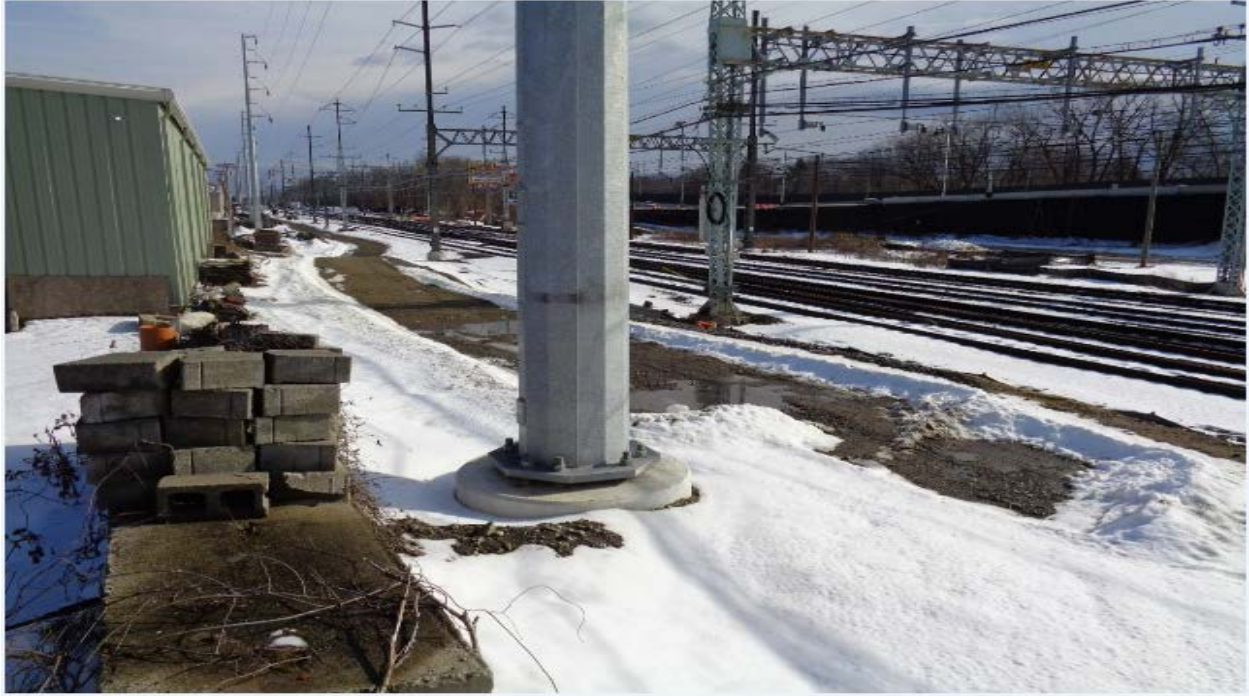
Structure 868N access road
