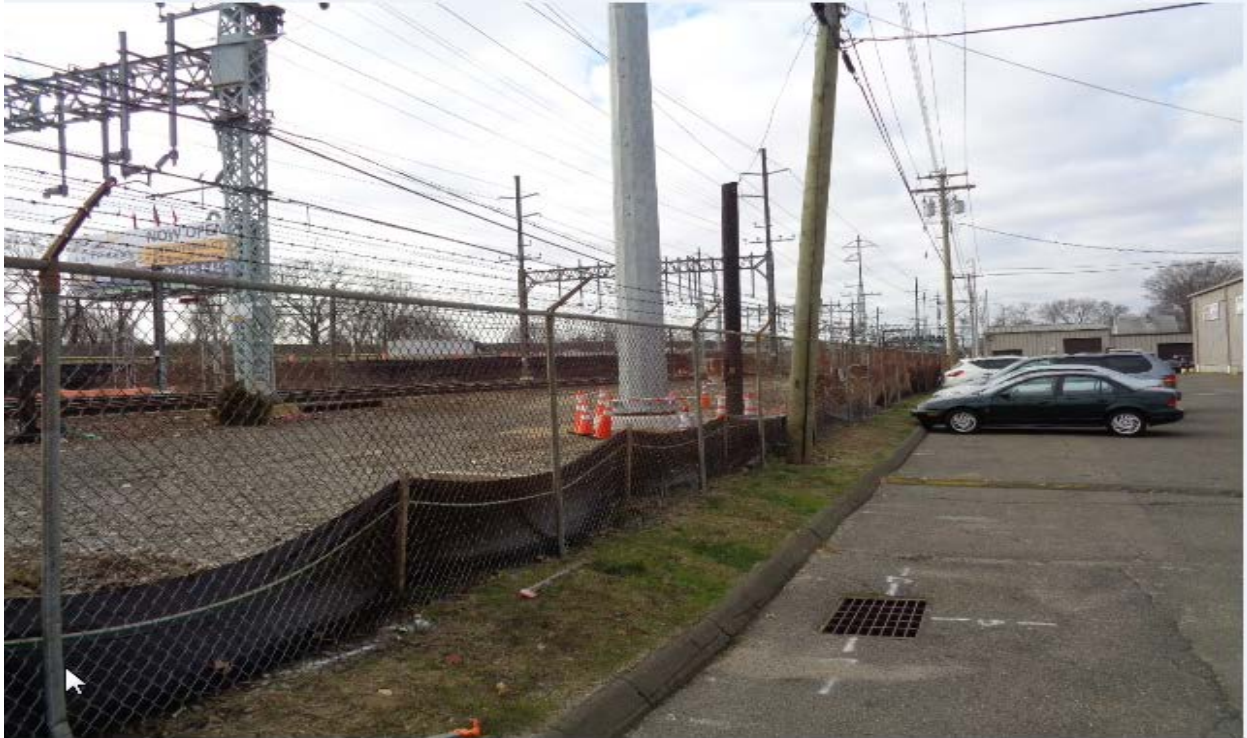
Erosion and Sediment controls at Structure 870N
