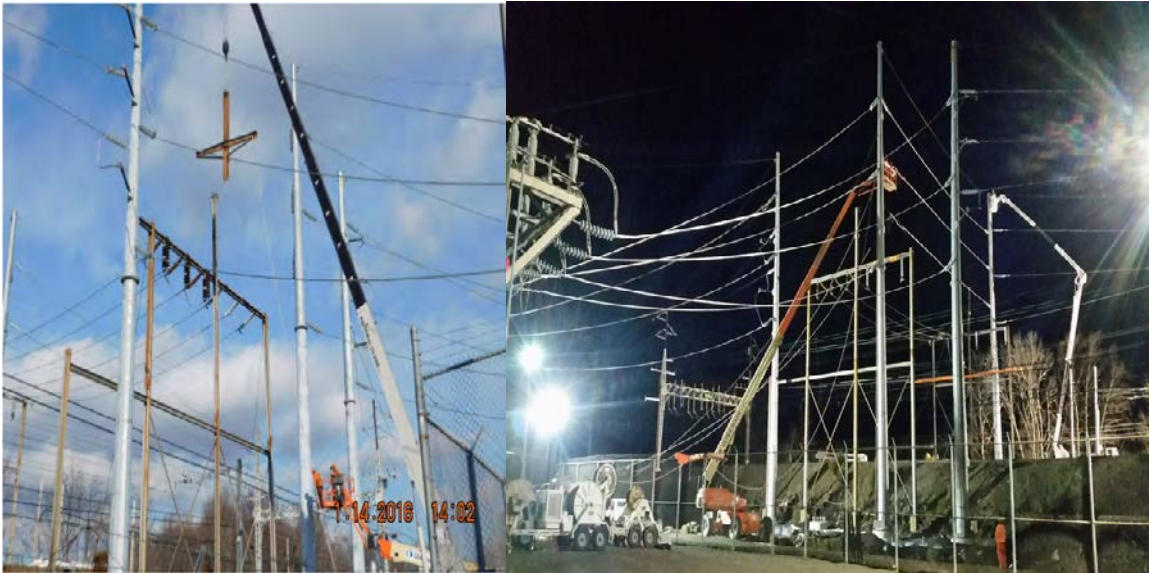
'H' frame structure removal and 4-track crossing to install conductors
