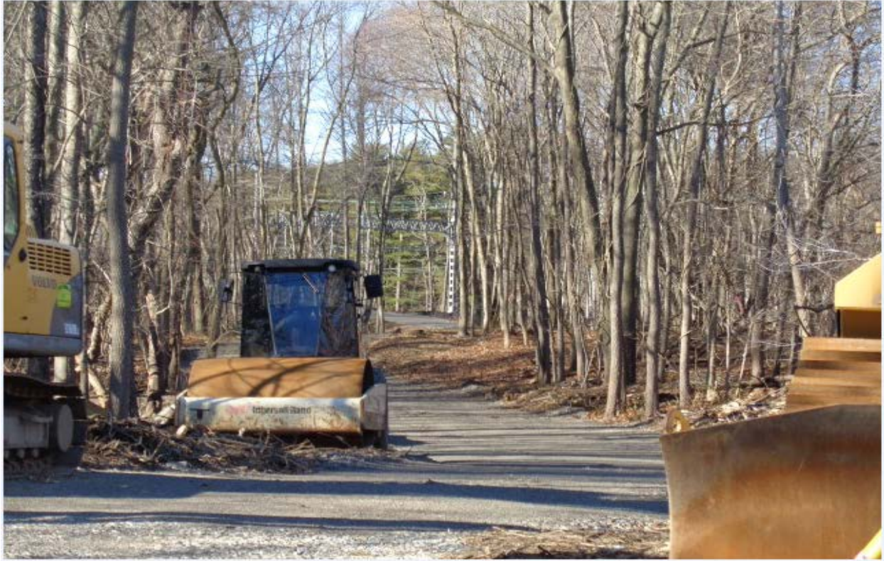
Access road for Structure 882S & 883S
