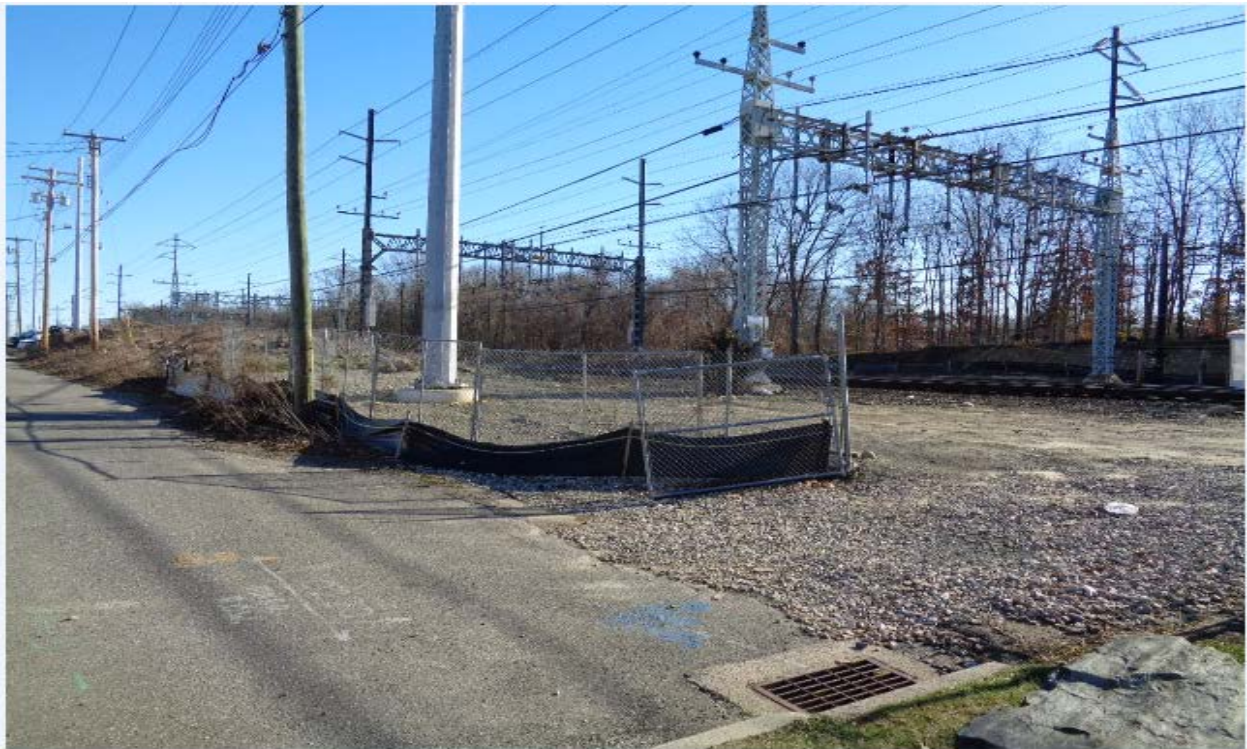
Access gate to Structure 871N
