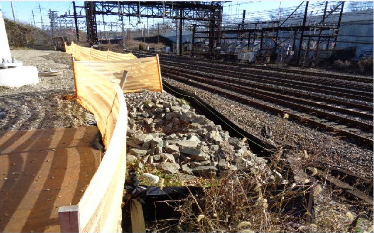
Erosion and Sediment controls at Structure 867N
