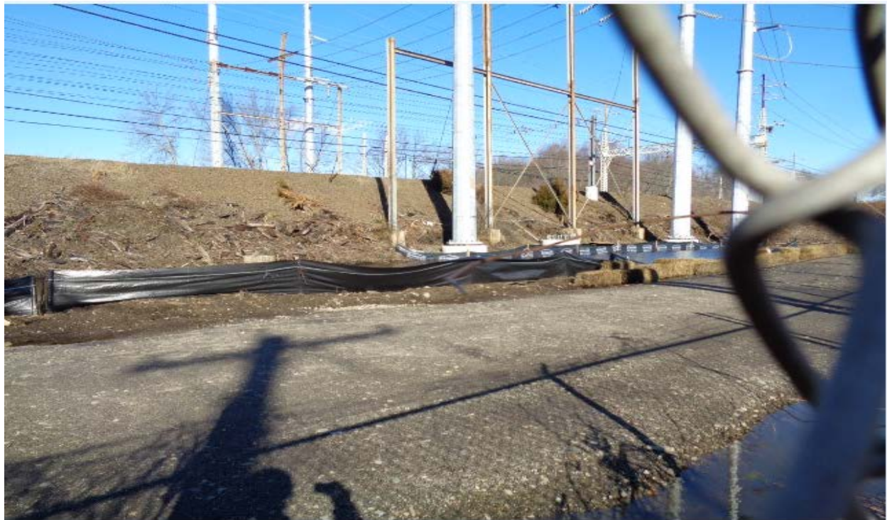
Erosion & Sediment Controls at Structure 887S
