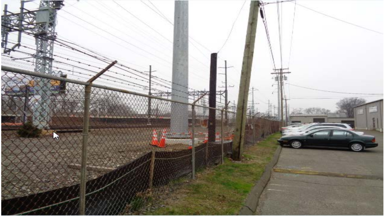
Structure 870N Sediment and Erosion Controls
