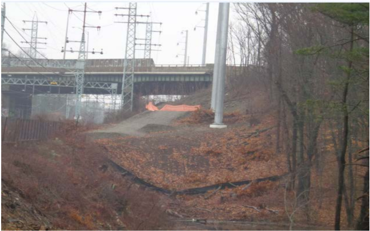
Structure 879N Sediment and Erosion Controls
