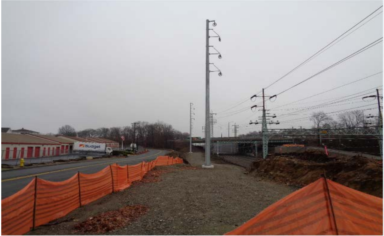
Structure(s) 876N and 877N
