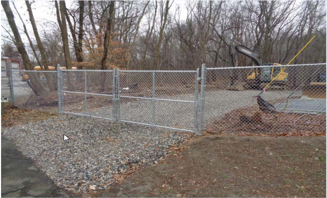
Structure 882S/883S access road with track pad
