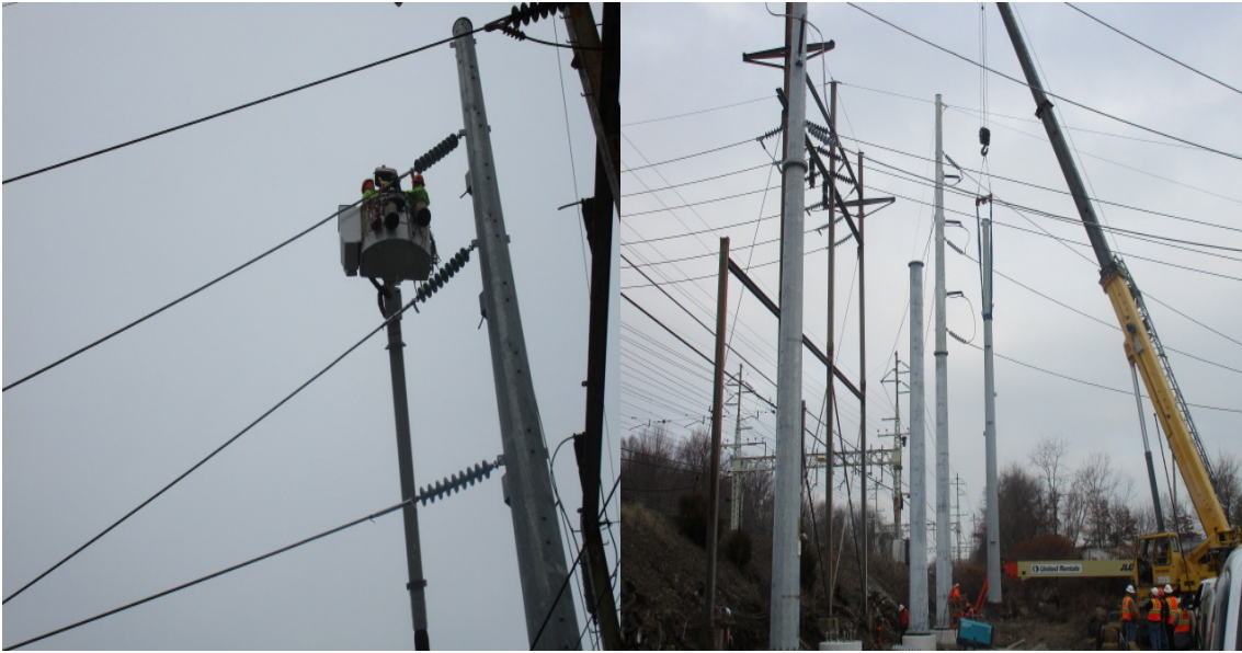
Installation of new conductor and setting of structure 887BNS
