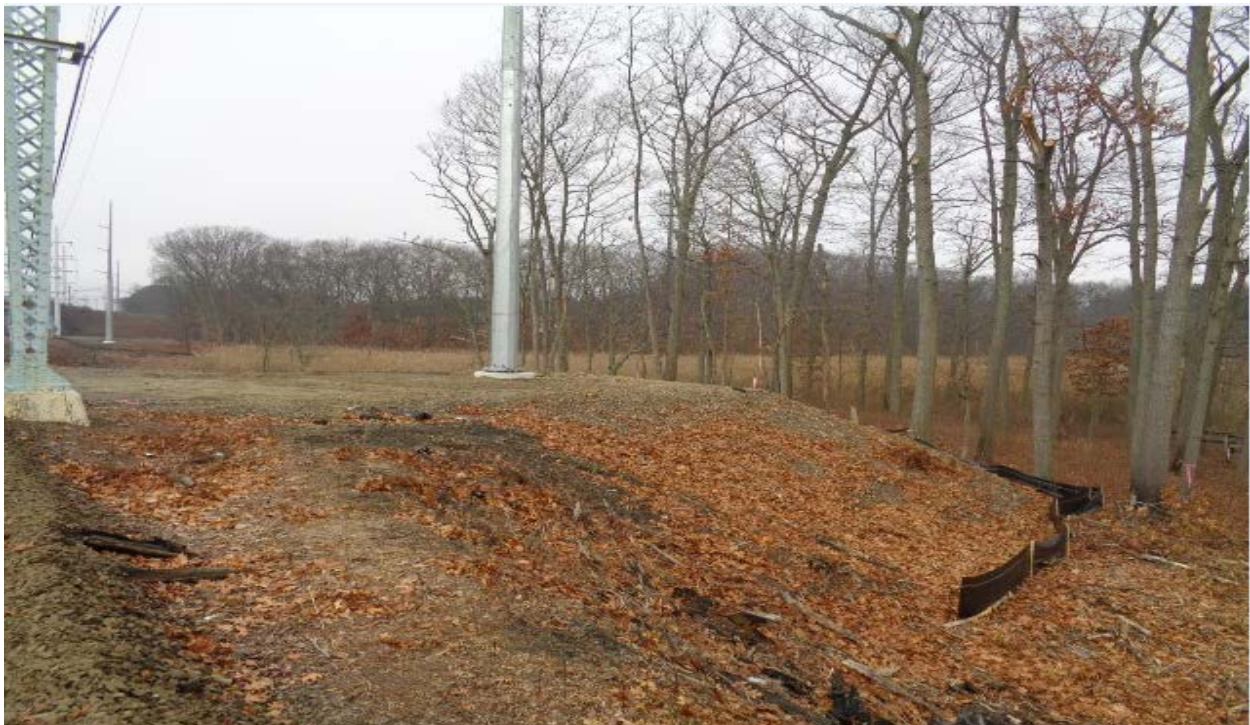
Structure 886N work pad with E&S controls
