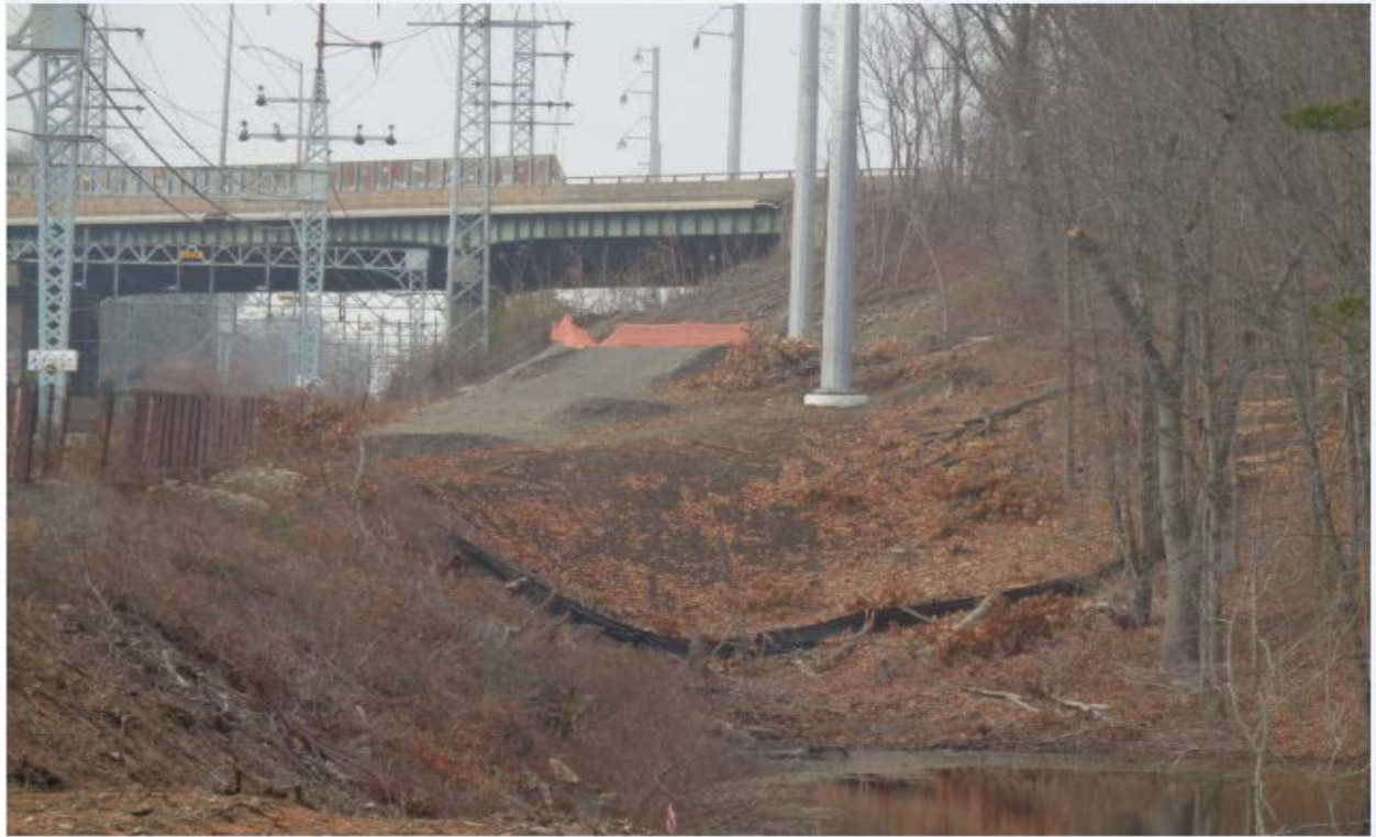
Structure 879N E&S controls
