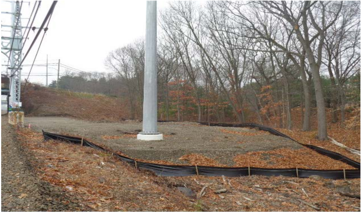
Structure 884N work pad with E&S controls
