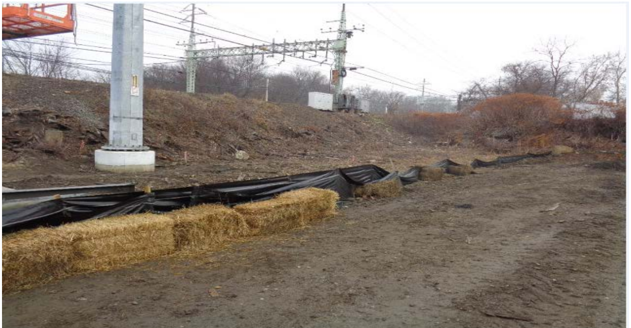
Structure 887S work area with E&S controls
