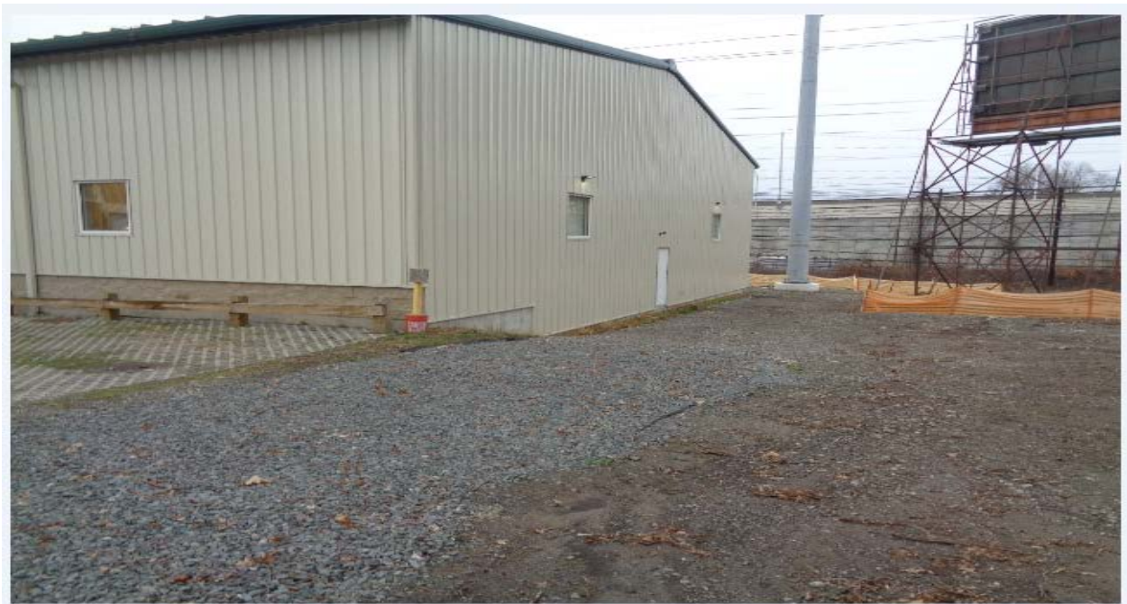
Structure 867N track pad
