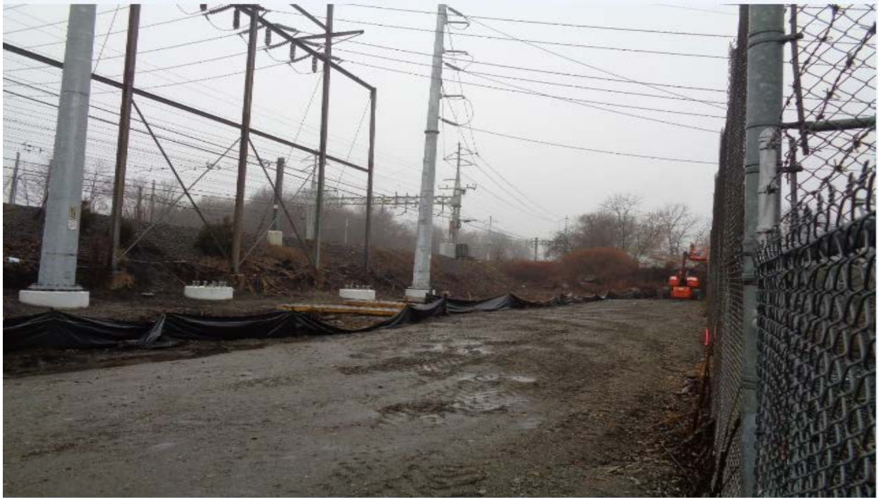
Structure 887S swamp mats and E&S Controls
