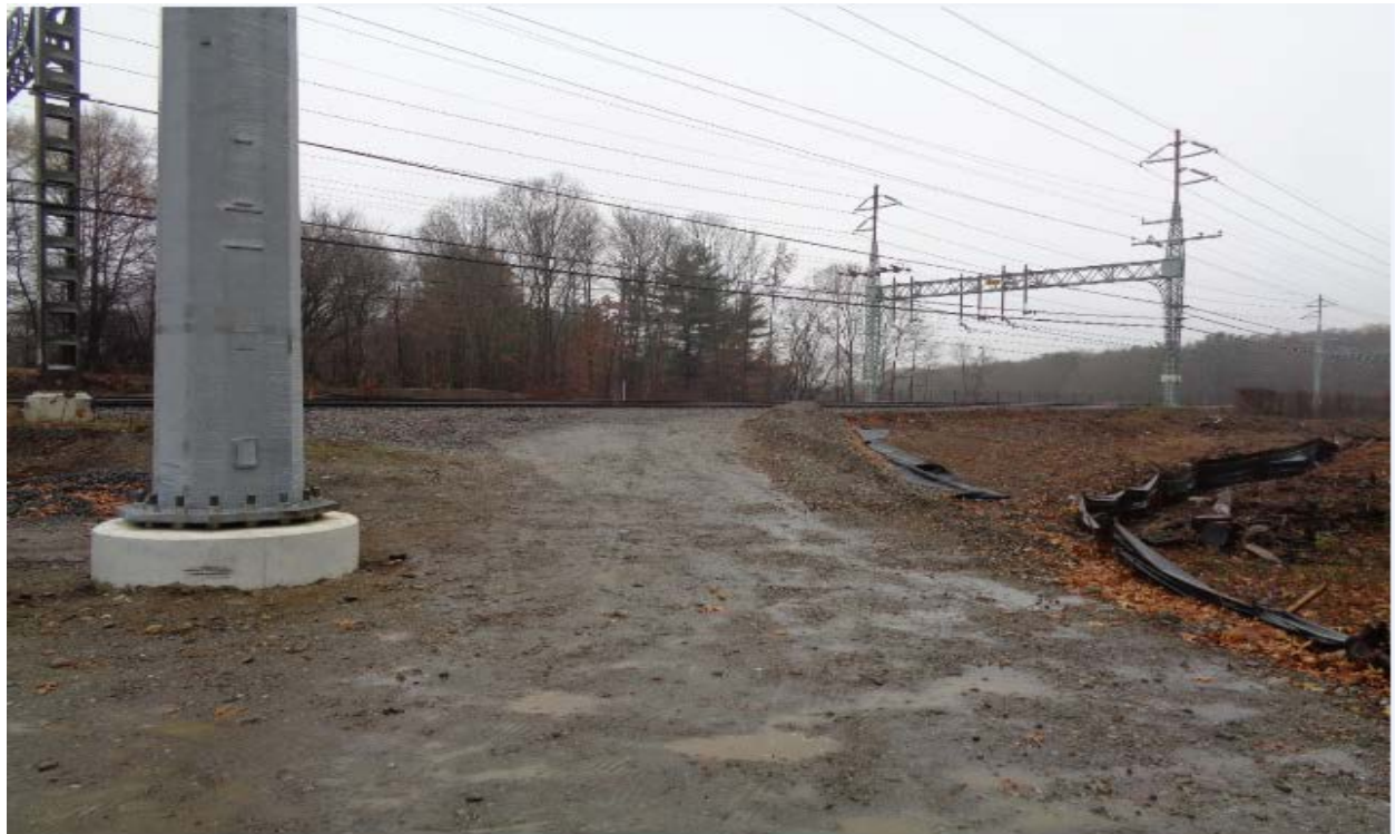
Structure 883N access road and E&S Controls
