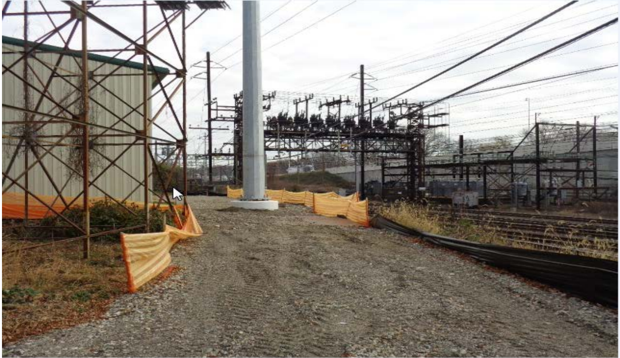
Access Road Structure 867N
