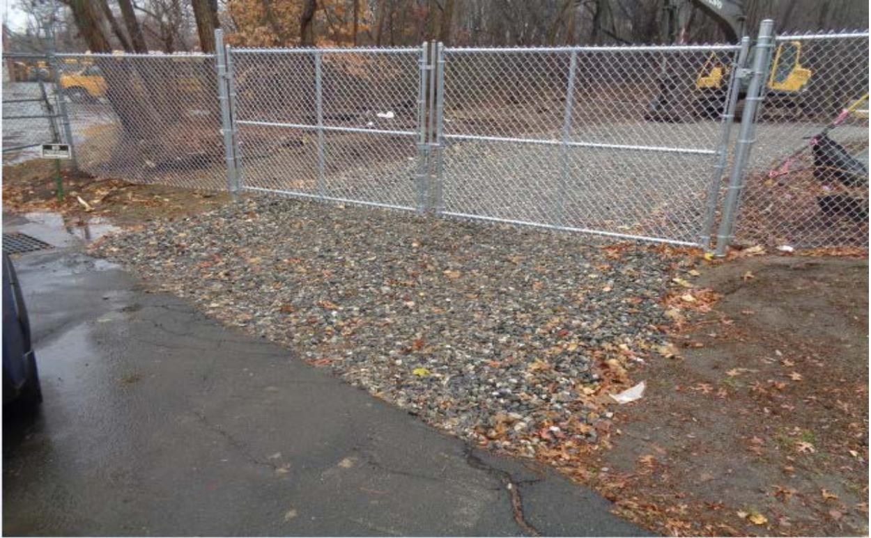
Track Pad for Structure(s) 882S and 883S
