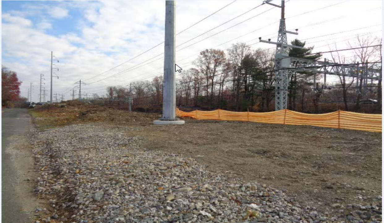
Structure 875N track pad abutting public road
