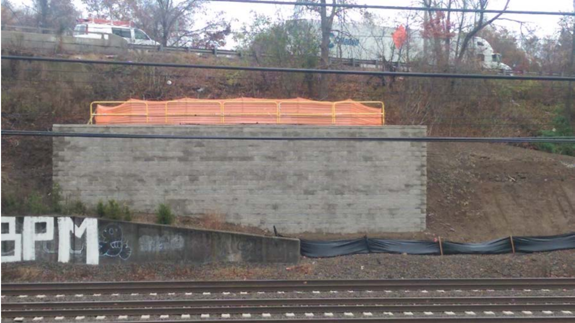
Containment wall located at 878S
