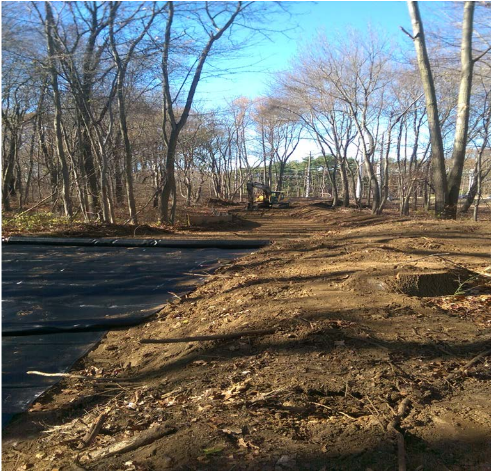
Clearing/Grading near Winkle Bus Entrance
