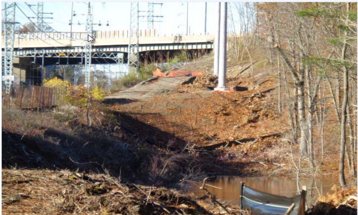
Structure 879N – work area
