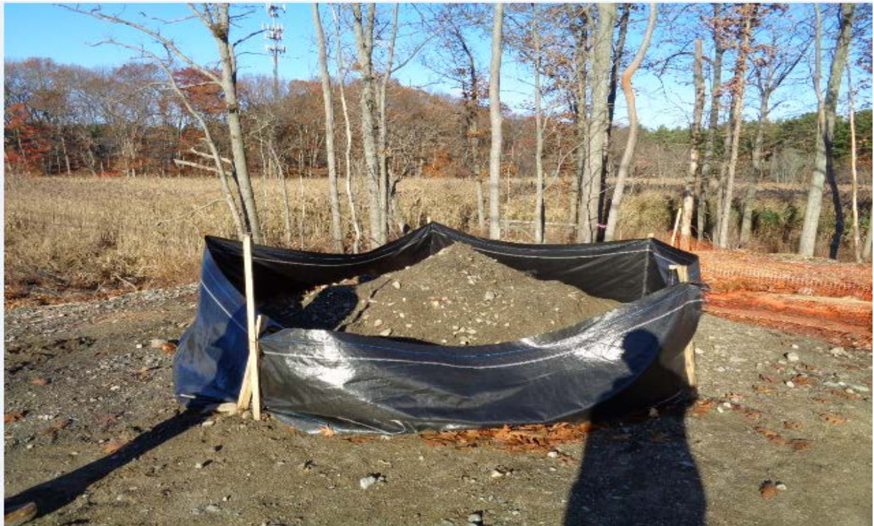
Structure 886N – Soil stockpile
