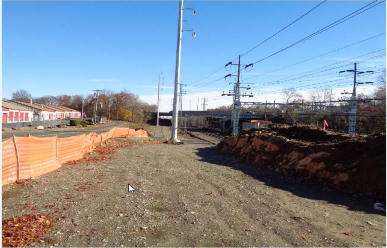
Structure 877N – Access road and erosion and sediment controls
