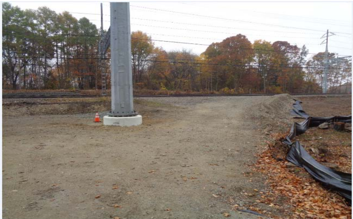
Structure 882N diversionary embankment along with erosion and sediment controls
