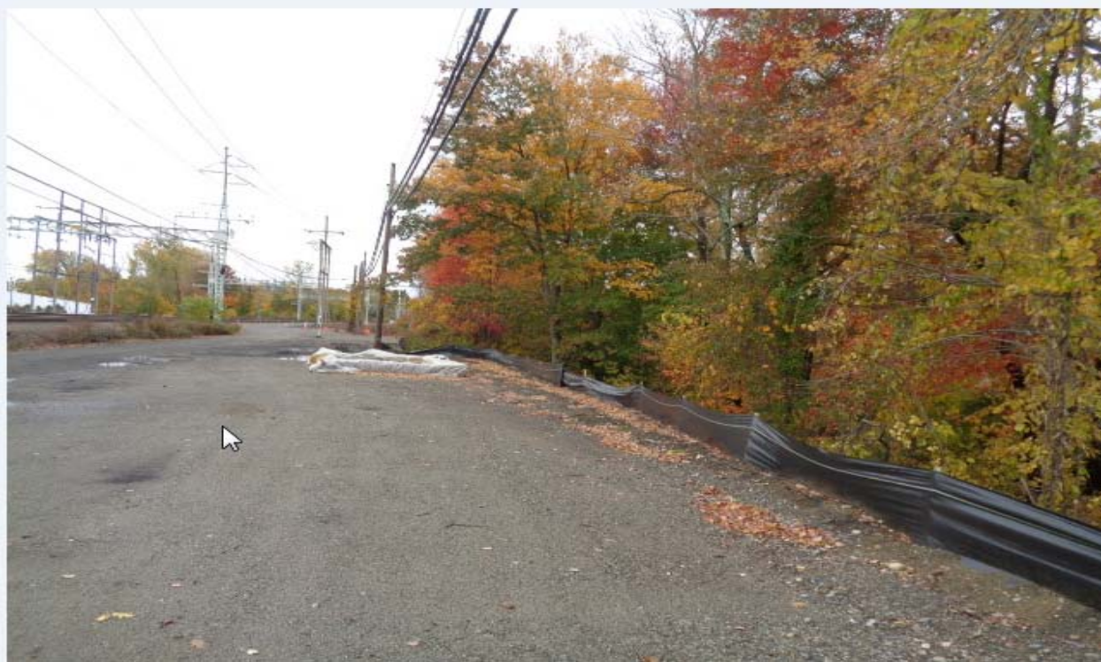
Structure 887N Work area along with erosion and sediment controls
