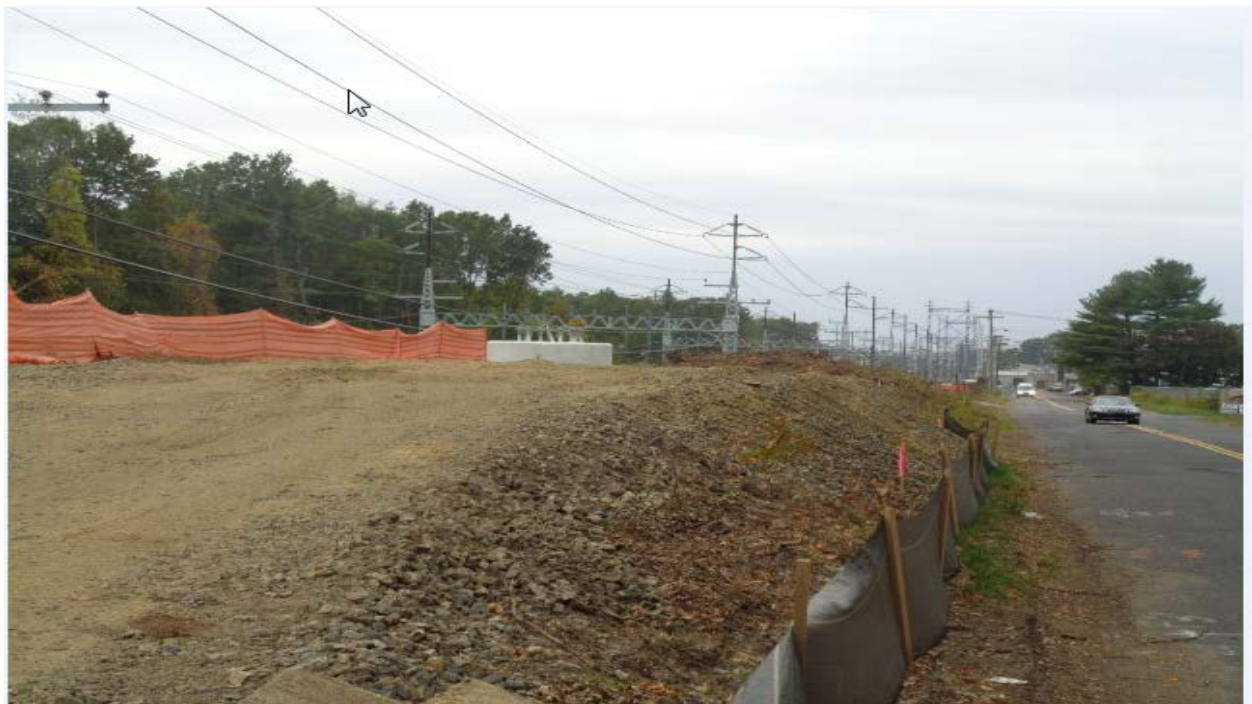
Work pad along with erosion and sediment controls at structure 878N
