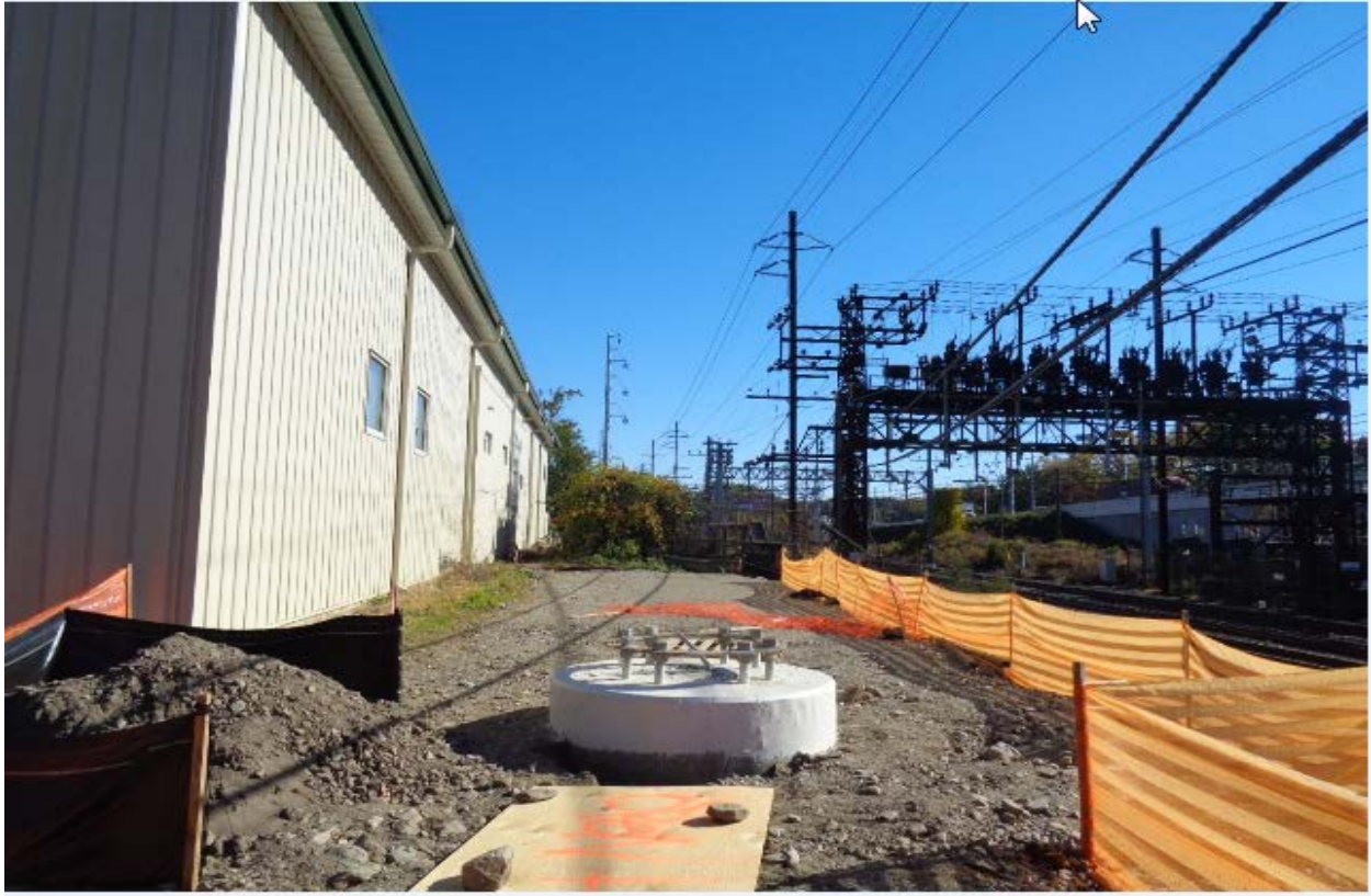
Structure 867N silt fence around stockpile
