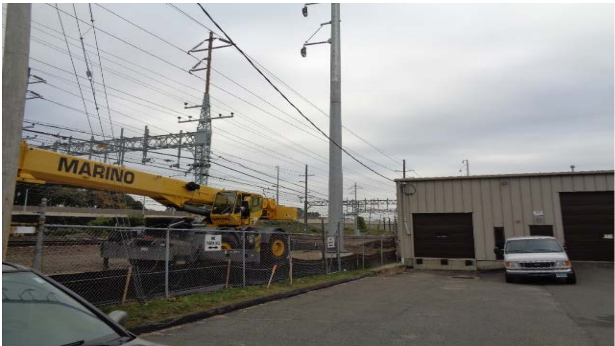
Work area at structure 869N
