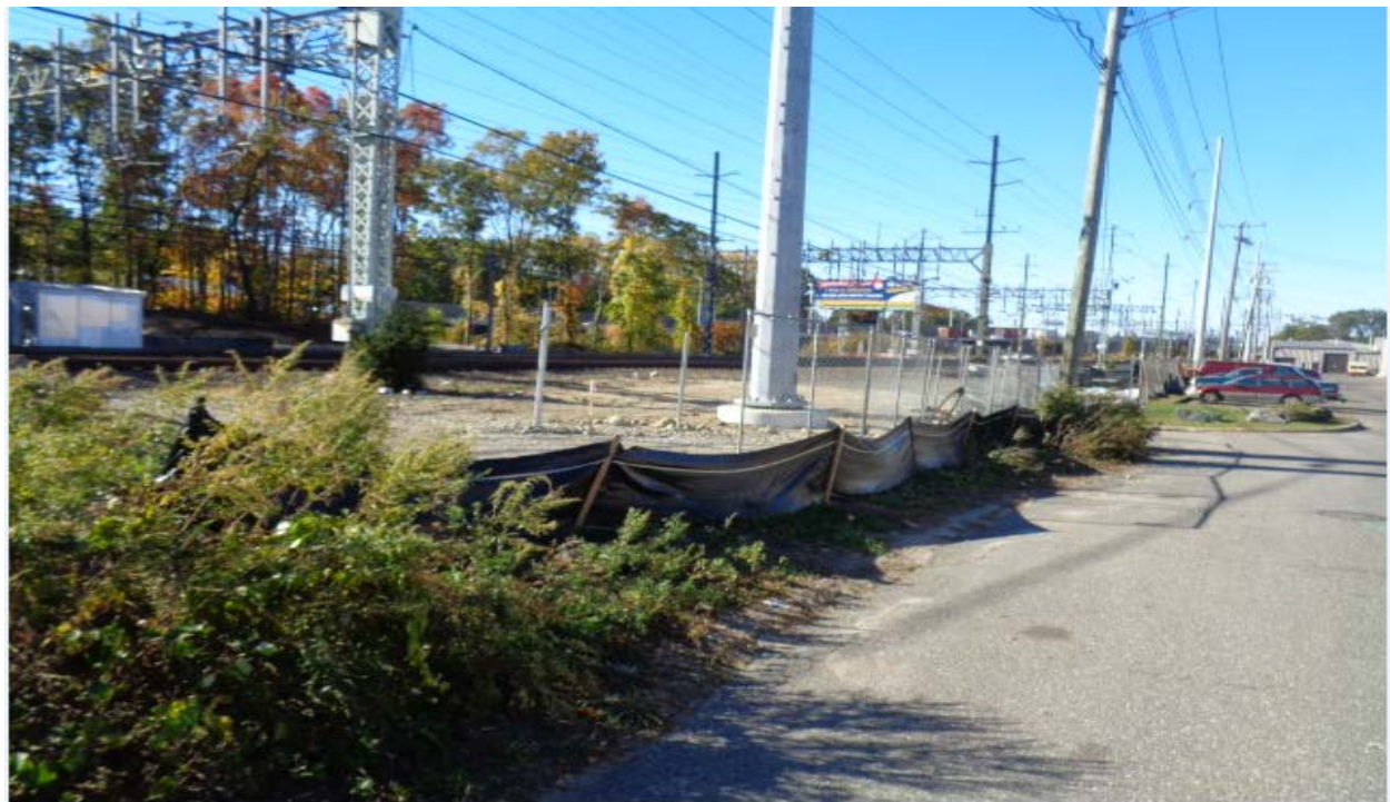
Structure 871N work area
