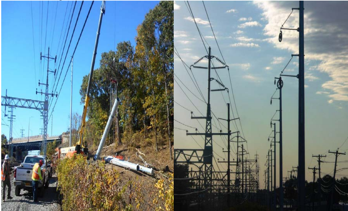
Setting structure 879N and 874N looking west
