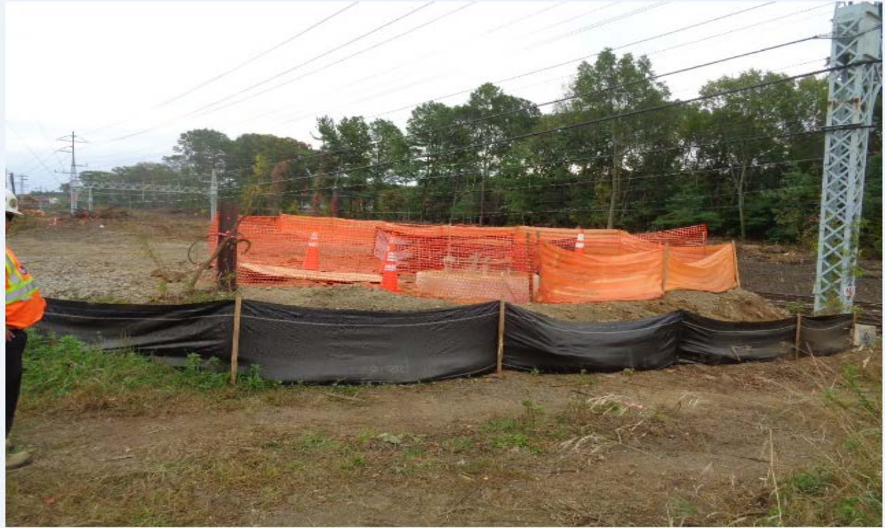
Erosion and sediment controls at structure 874N
