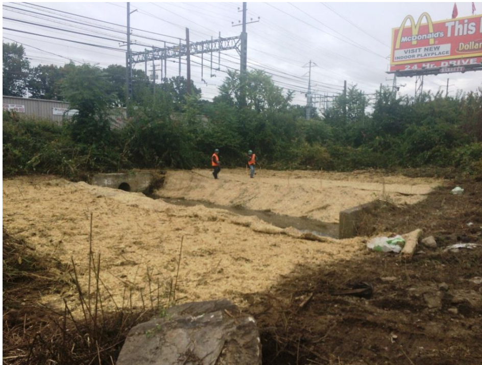
Wetland/culvert area, after stabilization
