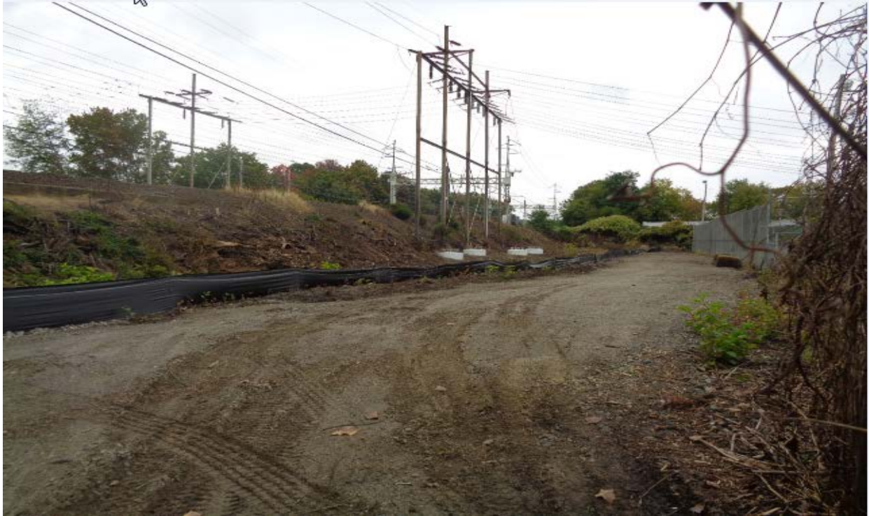
Erosion and sediment controls at structure 887AS
