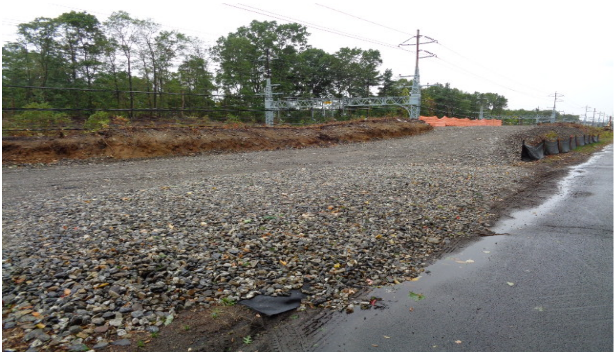
Access road, work pad and E&S controls at structure 878N
