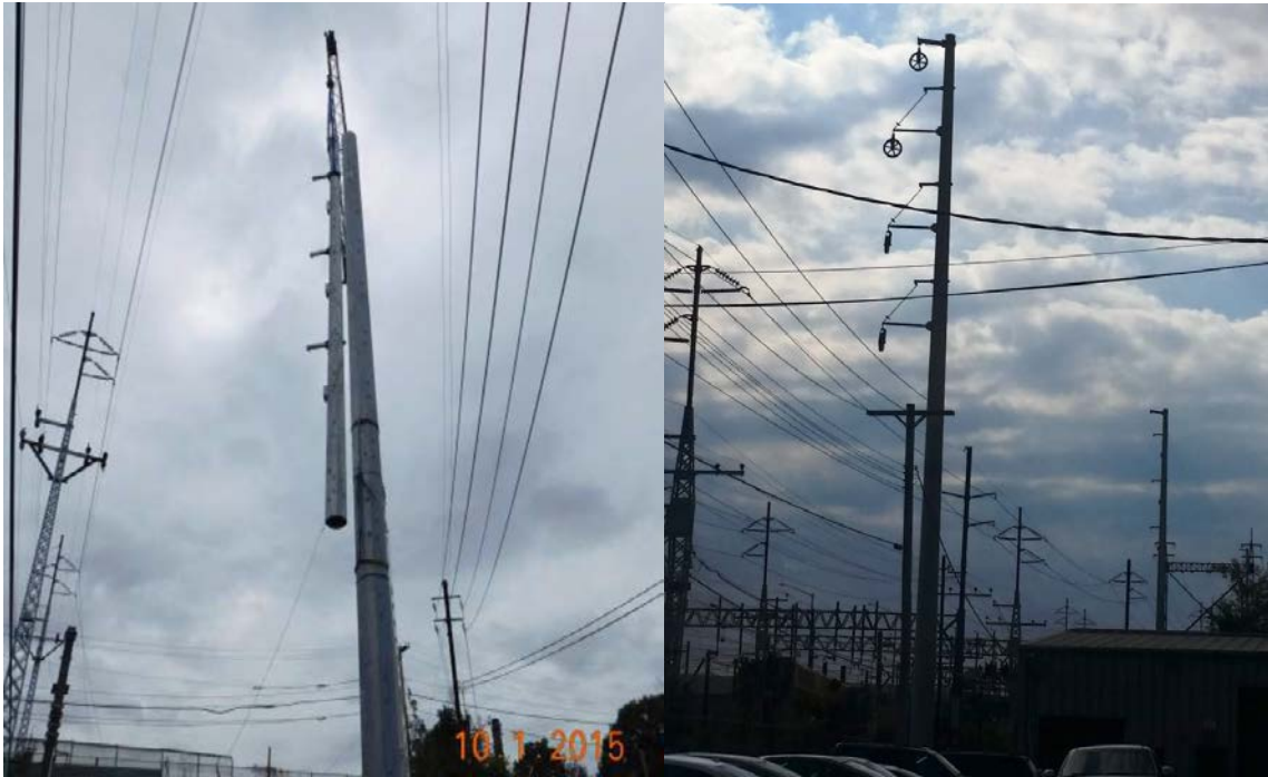
Setting structure 866N and fully dressed structure 871N
