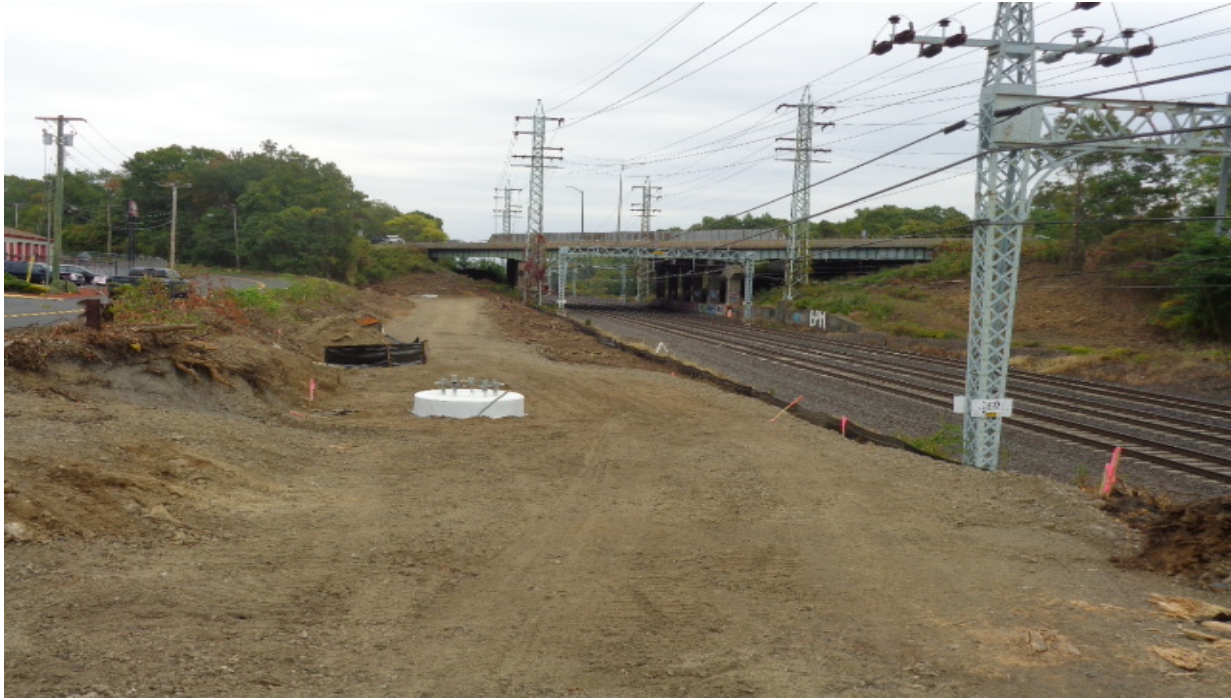
E&S controls at structure 876N
