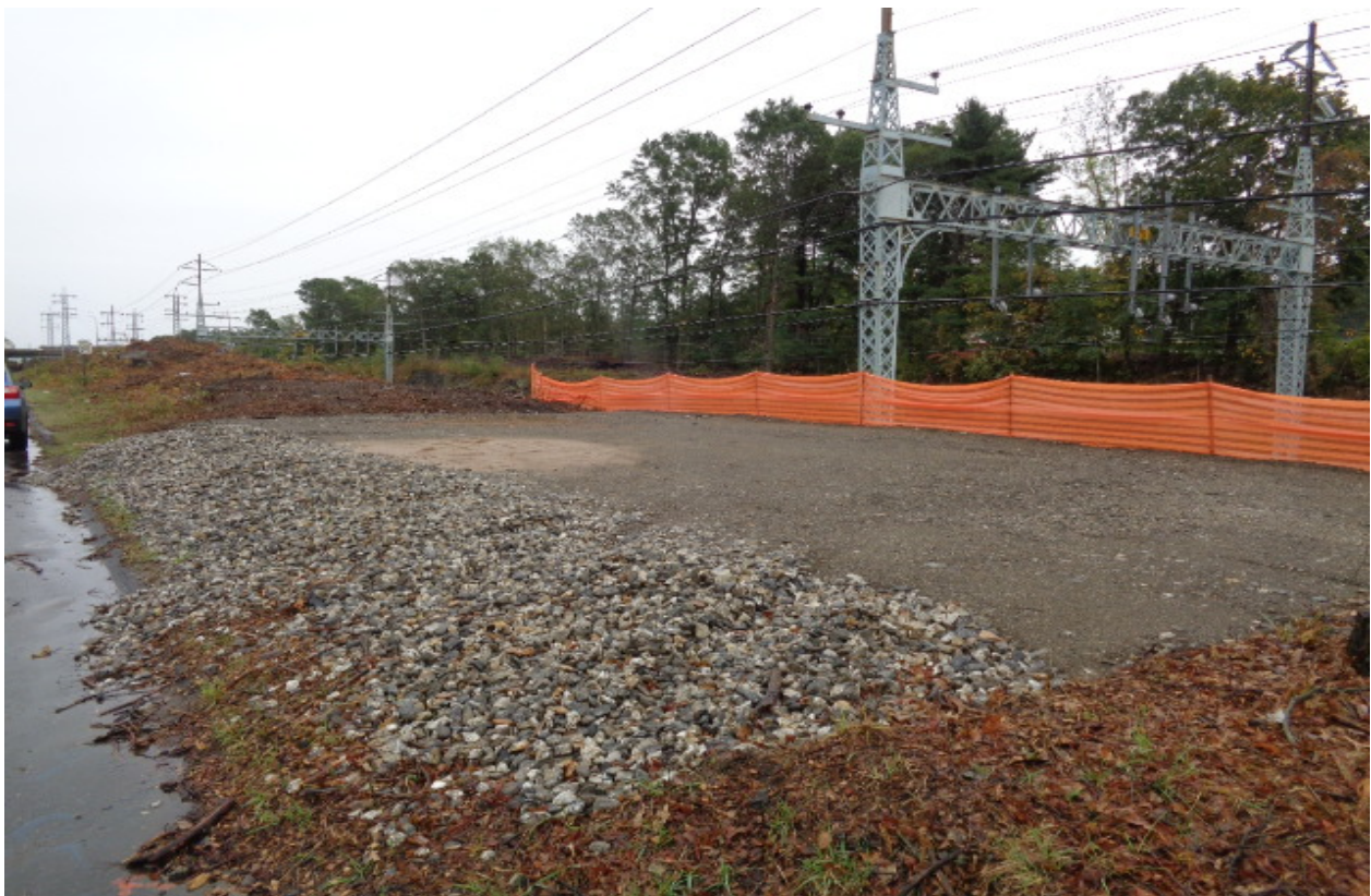
E&S controls along with work pad at structure 875N
