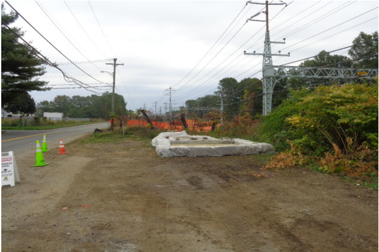
Concrete washout at structure 873N
