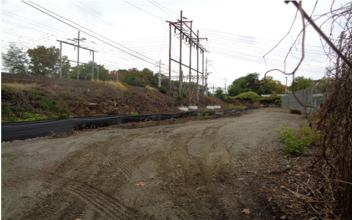
E&S controls, temporary fill removed and temporary stabilization behind Milvon Substation
