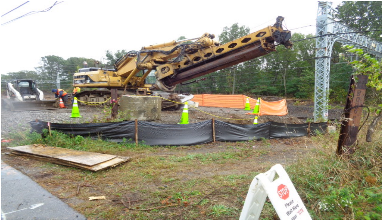
Drilling/E&S controls at structure 874N
