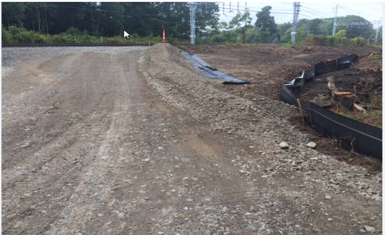
Silt fence, diversion swale and access road at Structure 882N
