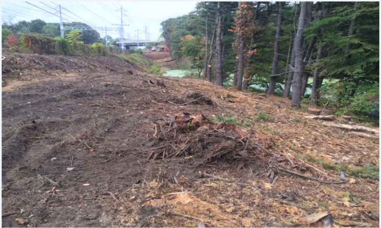
Vegetation clearing around structure 882N
