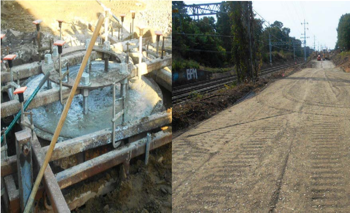
Foundation at 869N and work pad at 878N
