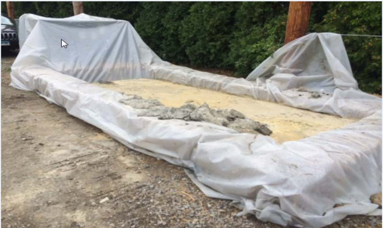
Concrete "washout basin" for Structure 887S
