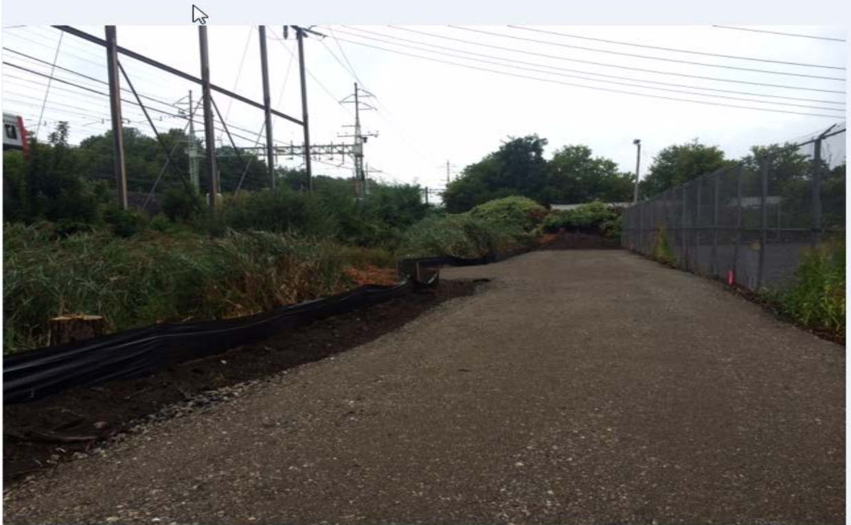
E&S controls, access road and word pad preparation at Structure 887S
