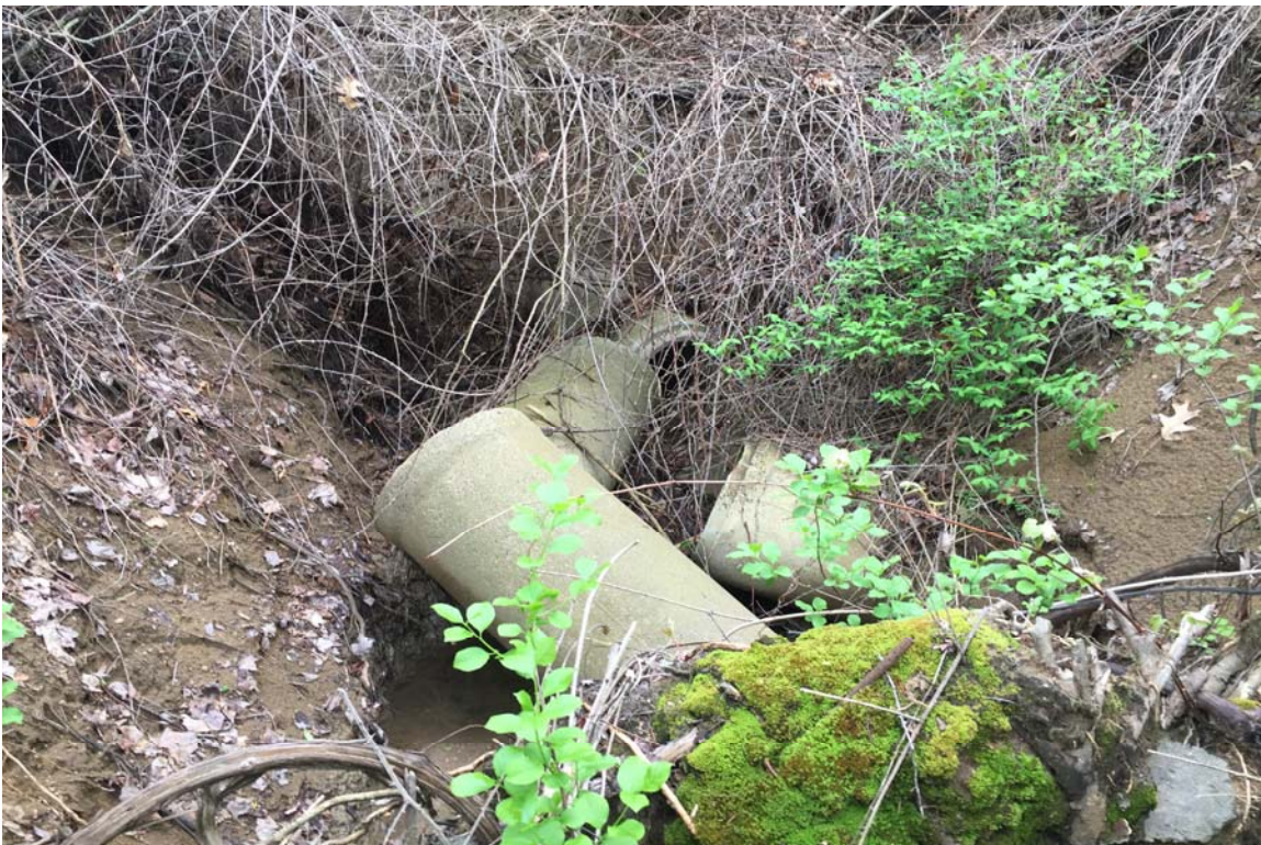
Photo 6: View of eroded and collapsed stormwater outfall from site to Podunk River looking south.
