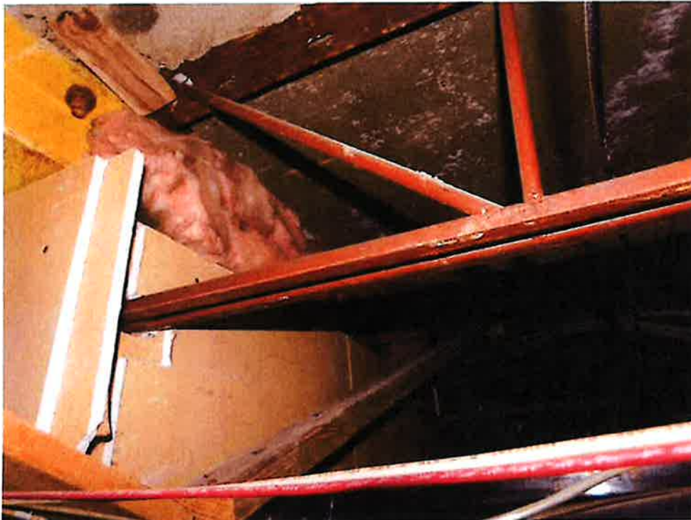
Photo 2: Sample photo illustrating the existing roof construction.
