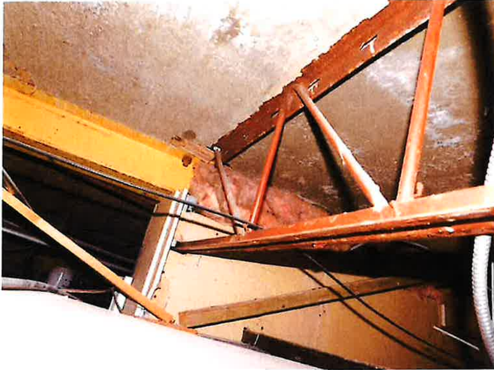
Photo 3: Sample photo illustrating the existing roof construction.
