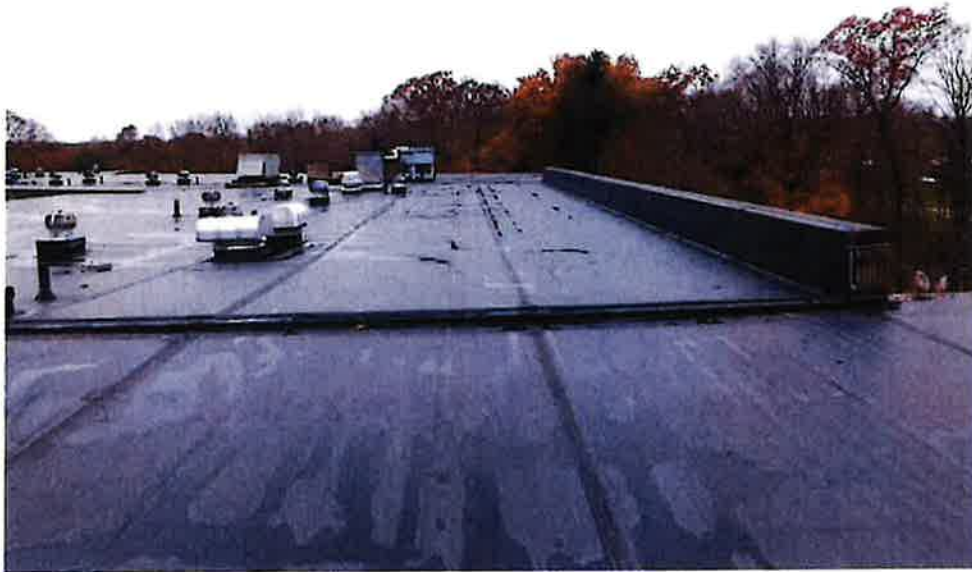
Photo 1: Sample photo illustrating the future equipment location.
