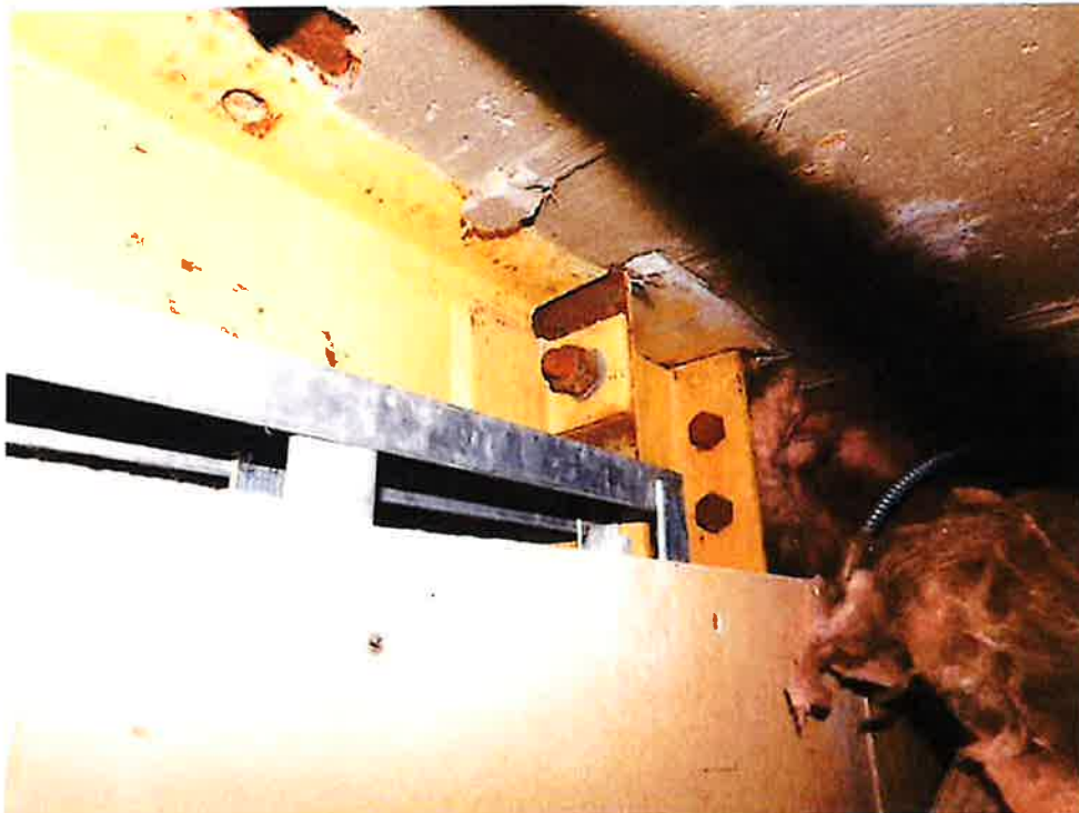
Photo 4: Sample photo illustrating the existing roof framing.
