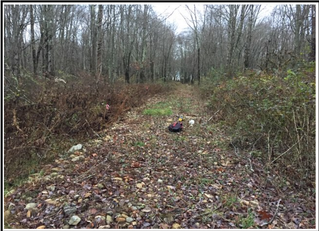
Photo 8: Maintained path looking northeast towards the hayfield (photo taken 11/5/18). The path is raised approximately one to two feet and comprised of stones where adjacent to Wetlands C, D, E, F and G.
