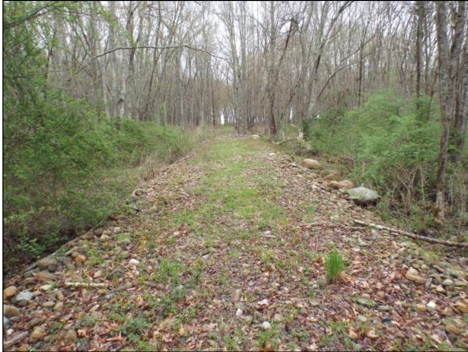
Figure 17. Overview photo of the central portion of the Northern Access Road facing east (note this area has been filled with gravel over wetland soils).
