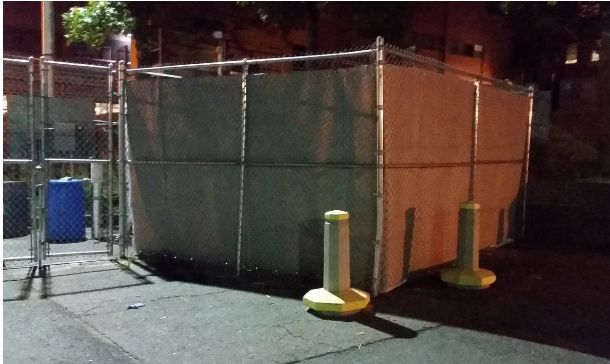
Figure 9. Eight Foot Fence Surrounding Doosan Cooling Module with Noise Treatment
