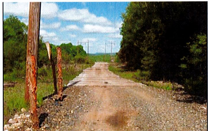
Construction mat access road.
