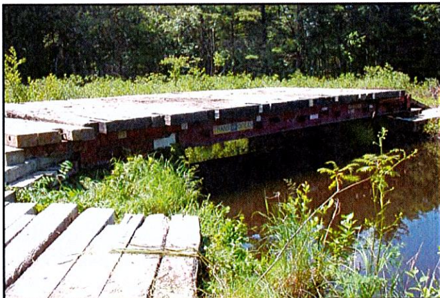
Rail car frame bridge crossing.
