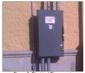
Figure 2: Electrical Disconnect
