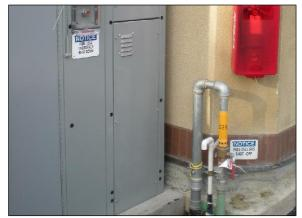
Figure 3: Manual Natural Gas Valve
