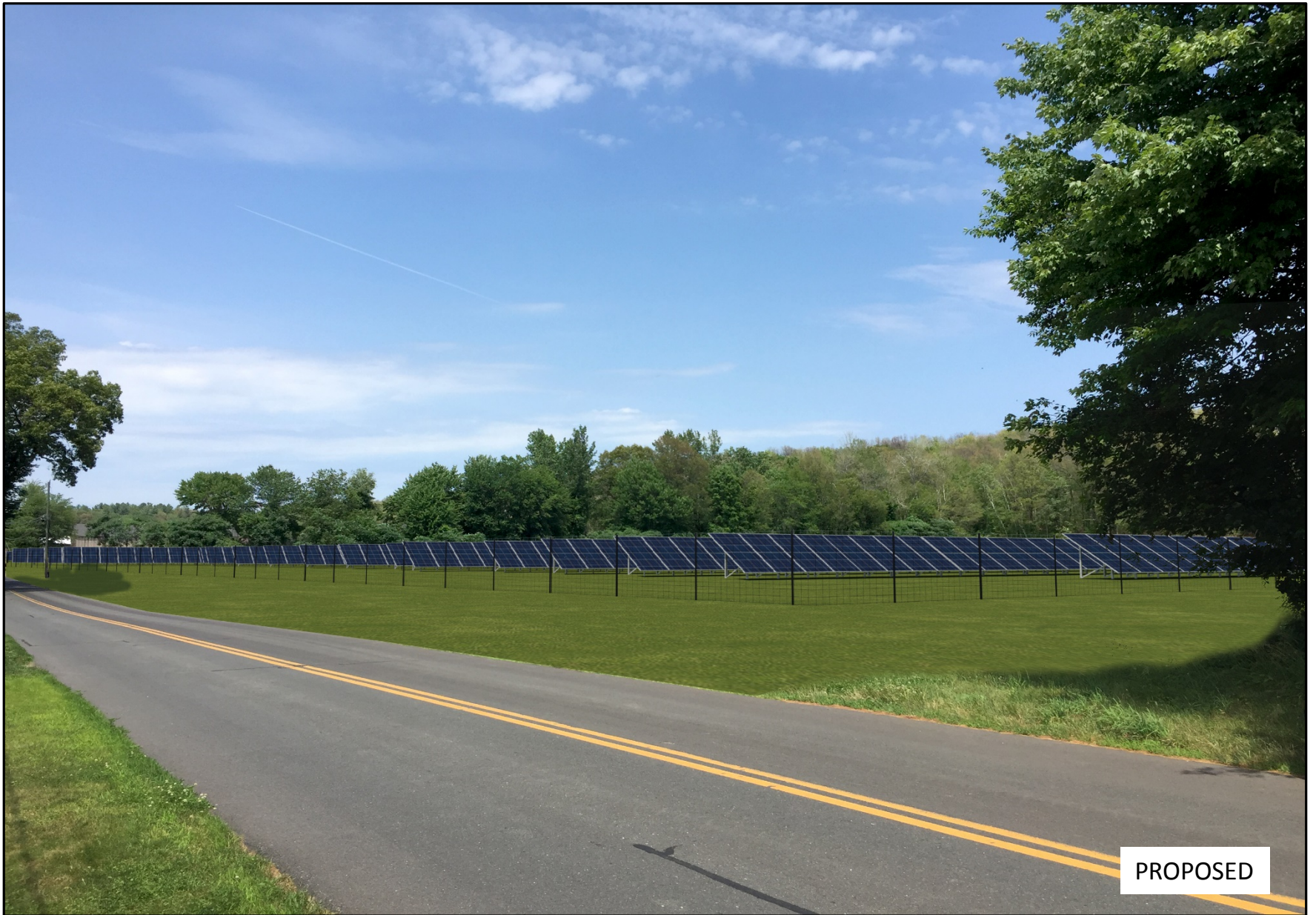
7: West of Charnley Road, looking northeast (Photo 3).
