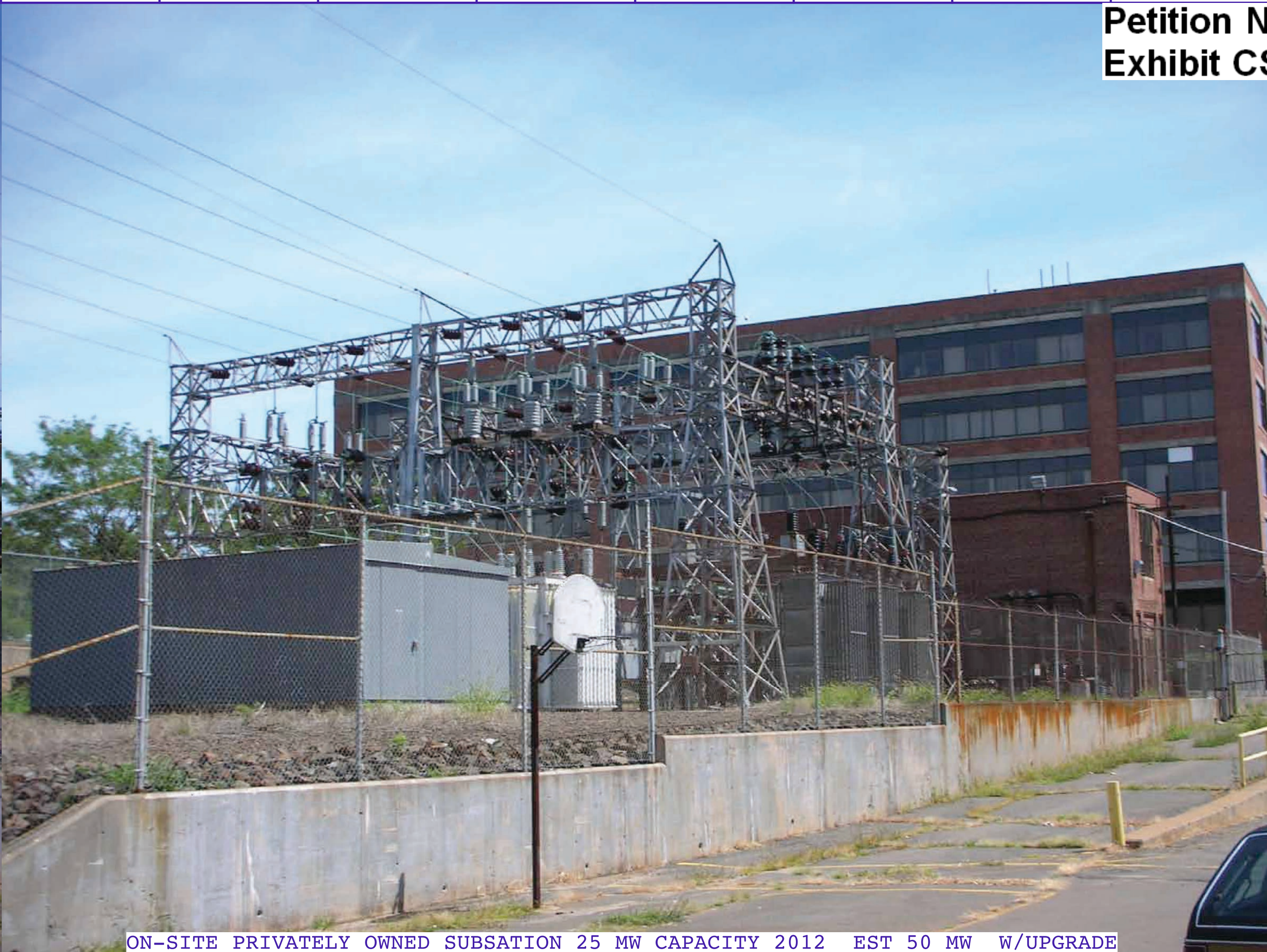
ON-SITE PRIVATELY OWNED SUBSTATION 25 MW CAPACITY 2012 EST 50 MW W/UPGRADE
