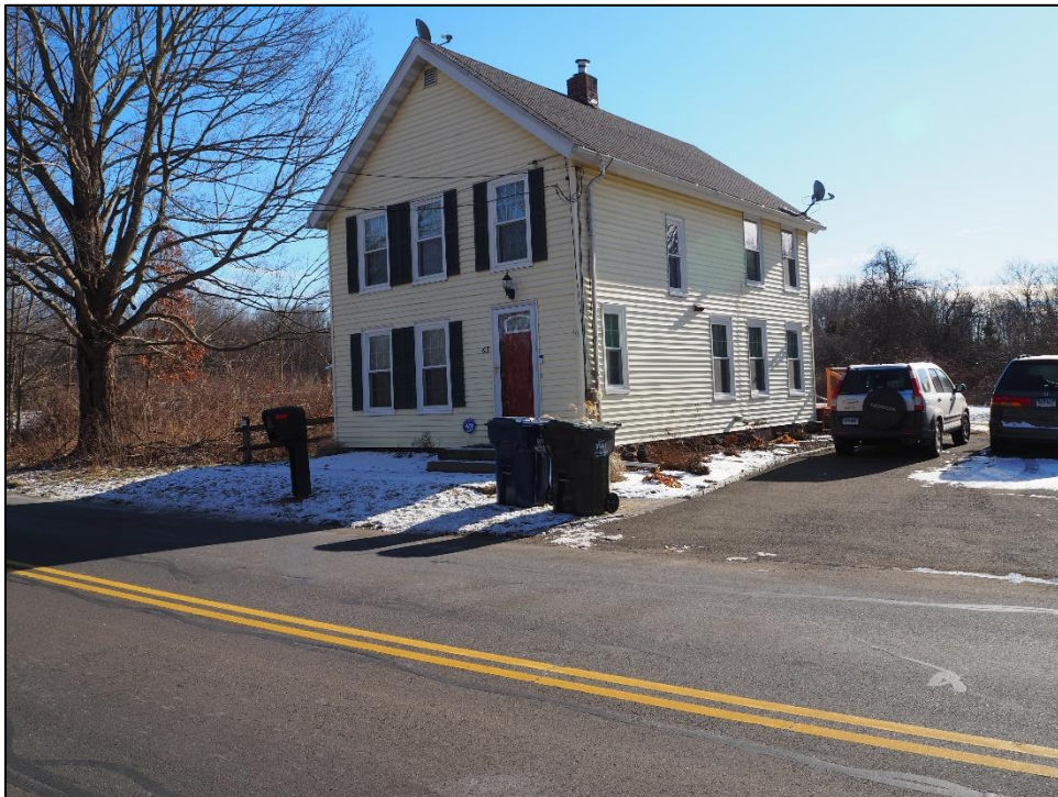
Photo 24. Overview photo home at 63 Maiden Lane (H. Tucker). Southeast view from Maiden Lane.
