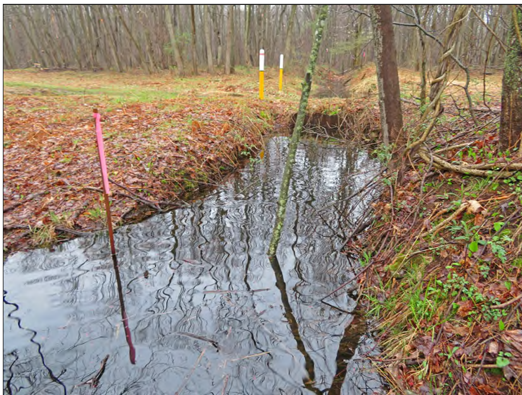
Photo 22: VP-2A outlet ditch with culvert under gas line ROW completely inundated due to artificial/temporary "dam" further downstream; facing northwesterly
