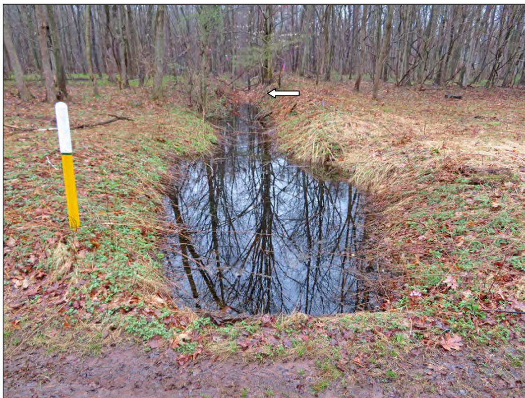
Photo 21: VP-2A outlet ditch with arrow indicating wood debris and leaf jam "dam," facing northwesterly
