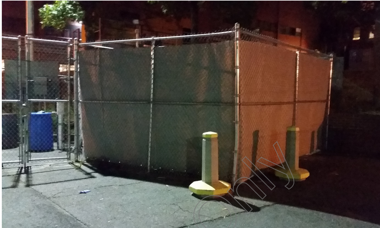
Figure 10. Eight Foot Fence Surrounding Doosan Cooling Module with Noise Treatment
