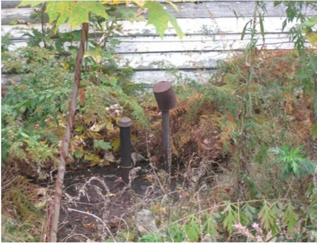
**Photograph 7:** View of a fill port and vent pipe on the northern side of the residence at the subject property.
