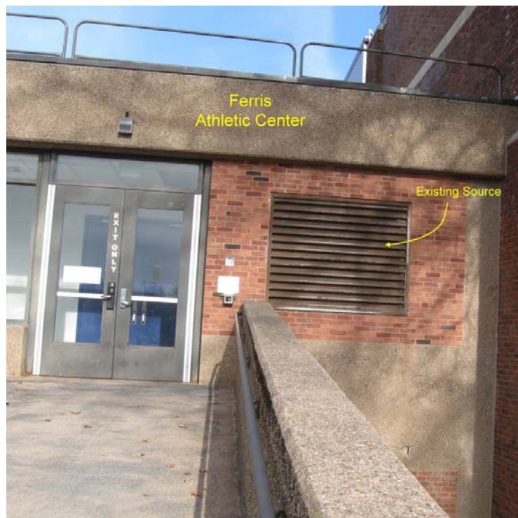
Figure 6: Field Image Showing the Intake Louver Near the Rear Ferris Center Exit
